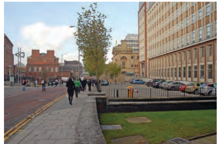
Conventional streetscape with a tired and uninspiring public realm on Surrey Street
