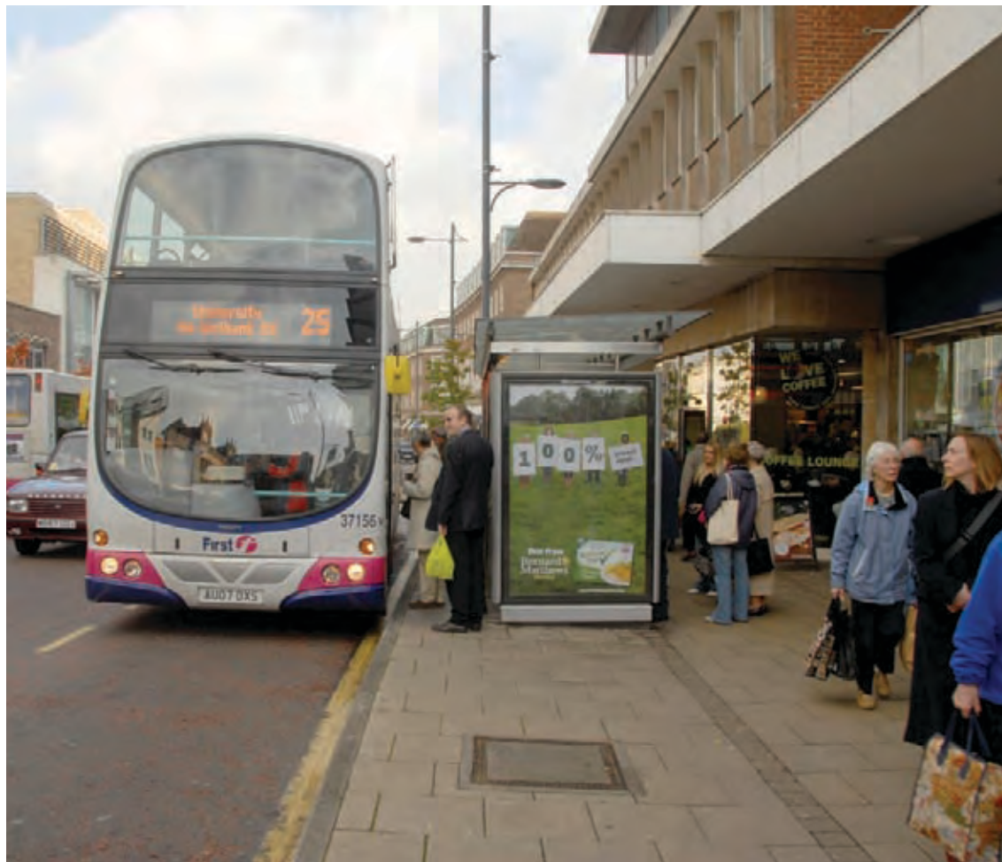
Bus shelters on St. Stephens Street reduce available footway width
