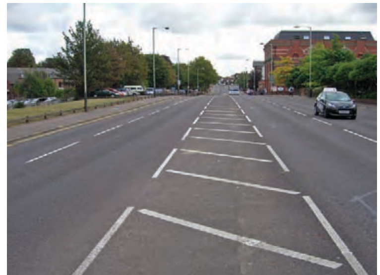
Queens Road is a major barrier for pedestrians
