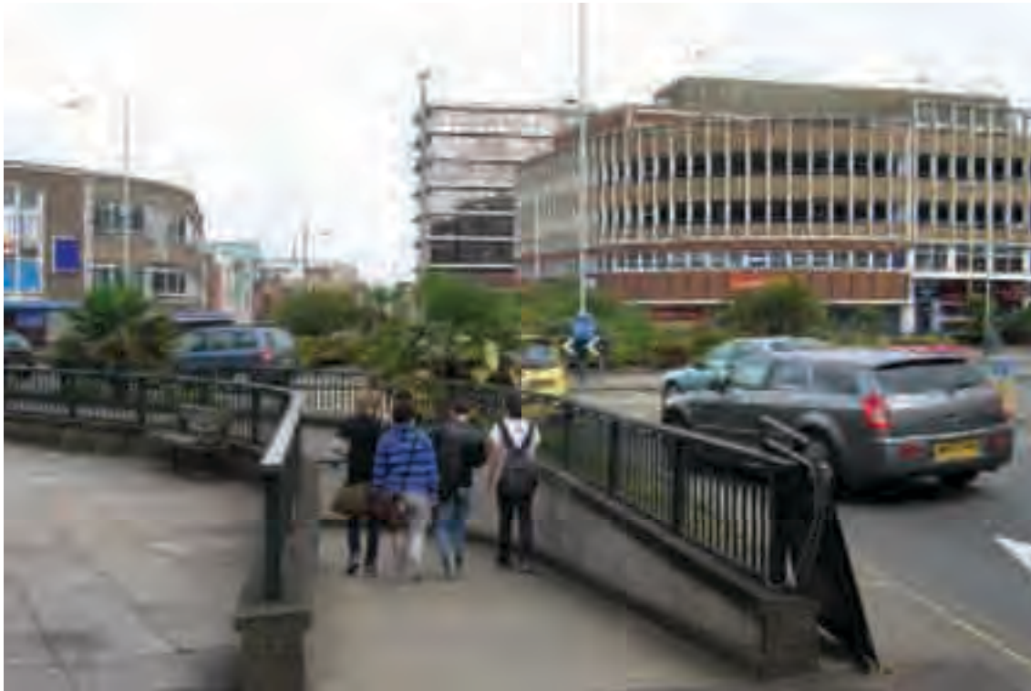
St. Stephens Street roundabout lacks the qualities of a gateway
