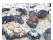
Iron-stained nodules set in lime mortar (a product of the local lime -burning industry).
