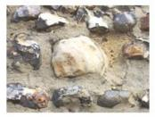
A large quartz cobble stone in the west wall. This is likely to be an 'erratic', brought to the area by a river in pre-glacial times.
