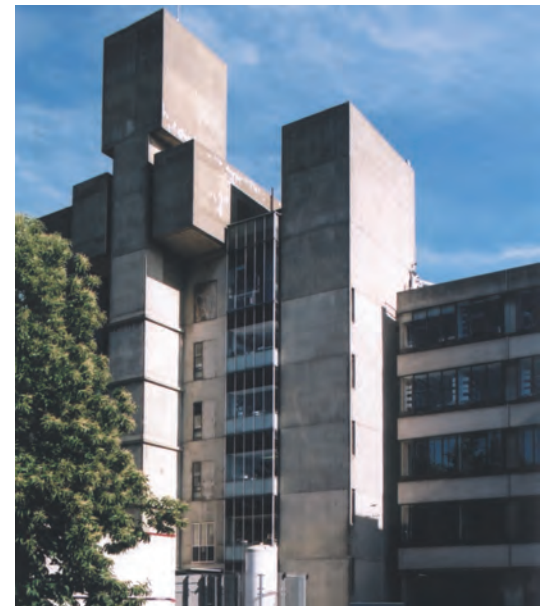
The north elevation of the Teaching Wall is punctuated by the service cores.
