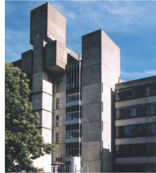
The north side of the Teaching Wall, showing the Chemistry service core.
