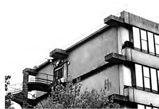
The 'unfinished' west elevation of the Teaching Wall with projecting nibs that were intended to link with a continuation of the building, and a 'temporary' spiral stair.
