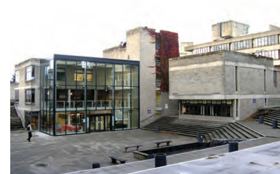
The Square, with the Restaurant (left) and Chaplaincy (right).
