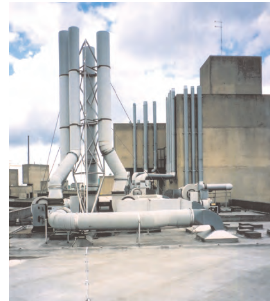
Teaching Wall roof: services and extract ducts have proliferated over the scientific departments.
