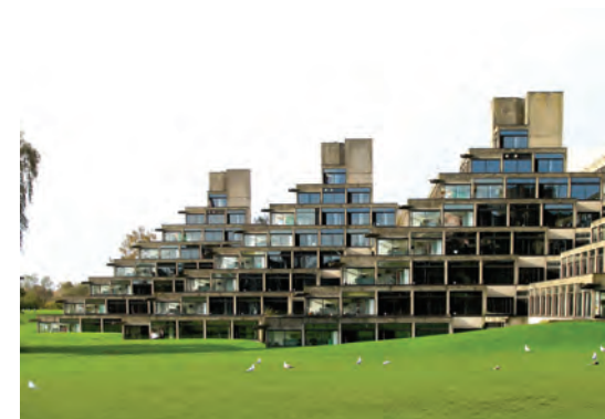
The south sides of ziggurats are the strongest architectural elements at UEA.
