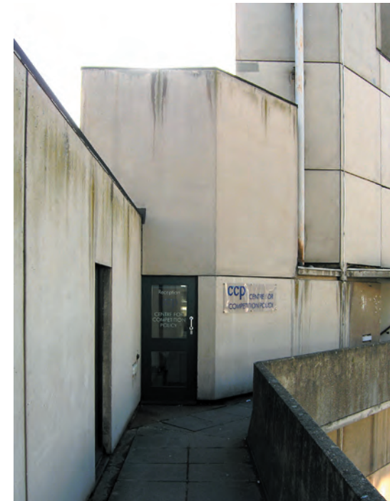
A few offices have taken space in the ziggurat residences. This is the Norfolk Terrace walkway.
