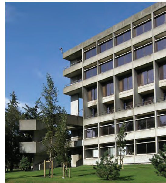
Library: south-west elevation. This phase of the building was completed in 1974.
