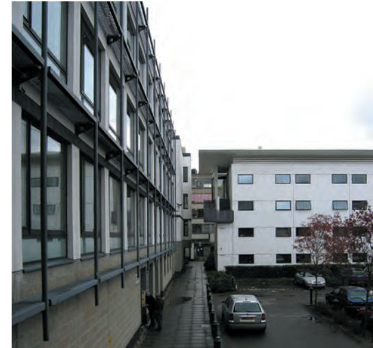
The west elevation of the Queen's Building (left) and the north elevation of Constable Terrace.
