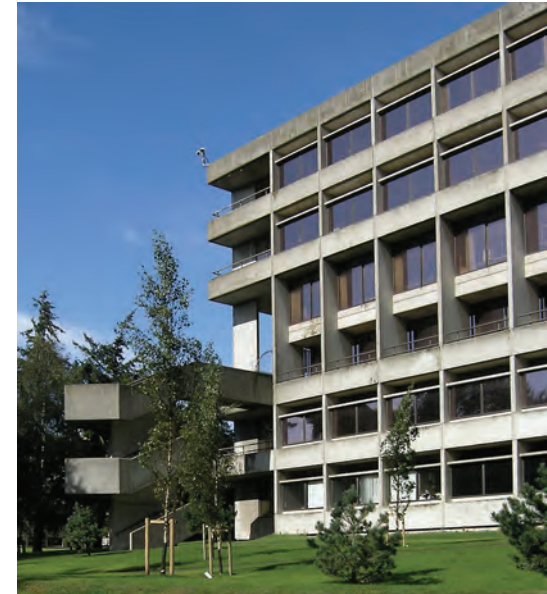
UEA's Library is a free-standing building with a deeply-modelled elevation of precast concrete panels.
