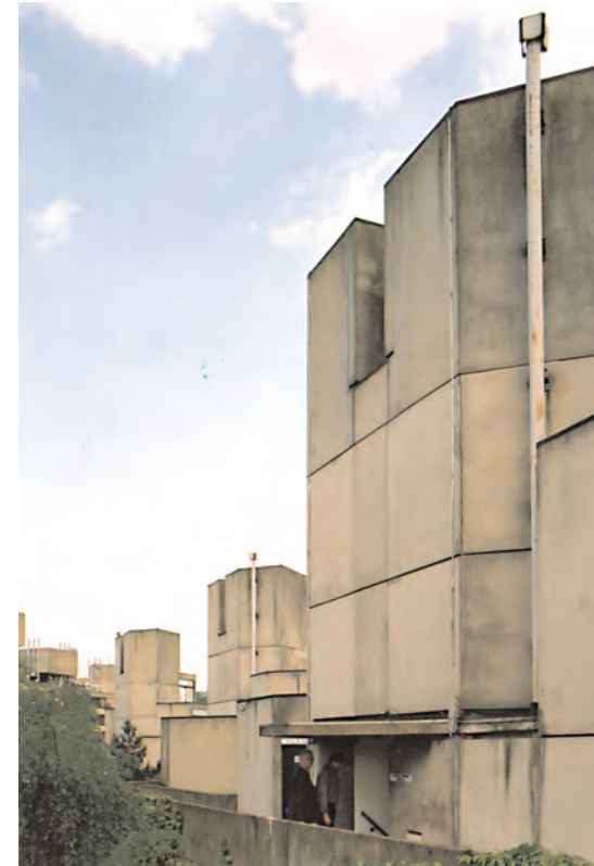
High-level walkway on the north side of Norfolk Terrace. The walkway is an integral part of the ziggurat, unlike the Teaching Wall walkway which is an independent structure. The tall metal flues appeared shortly after the ziggurats were completed.
