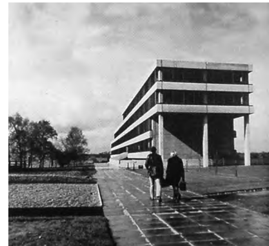
The east elevation of the Teaching Wall in about 1971, after the completion of Arts II but before the Registry was built.
