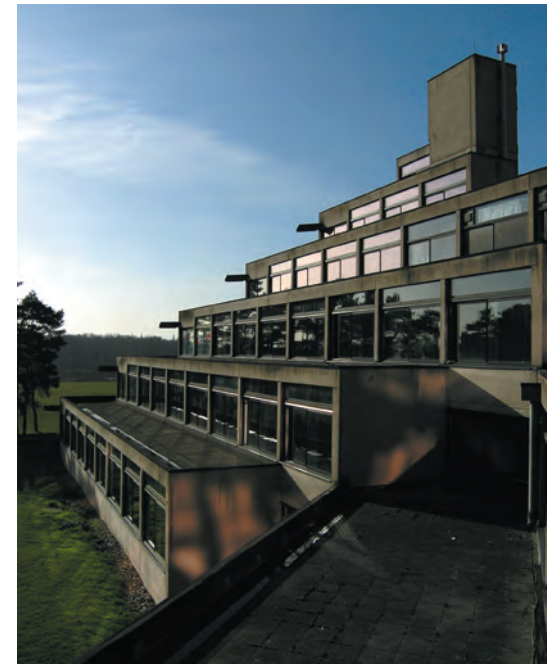
The south front of the ziggurats – which are actually cranked terraces – showing the roof terraces which were intended for use by the students. This has now been stopped for health & safety reasons.
