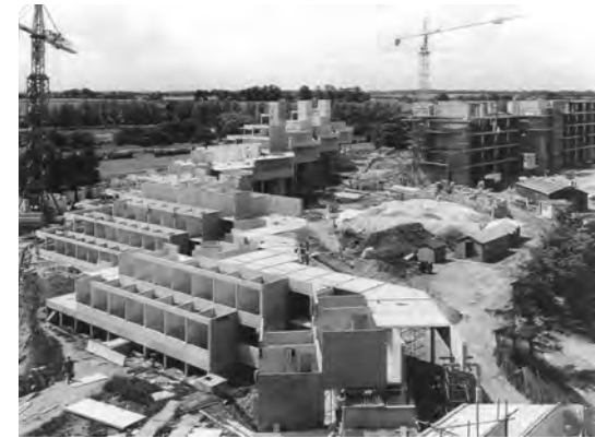
Construction in progress in 1965.
