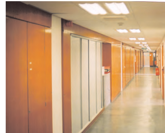
A Teaching Wall corridor that retains Columbian pine panelling. The suspended ceiling and lighting have been changed.
