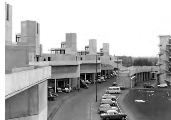
Norfolk Terrace in 1969 looking towards the Biology section of the Teaching Wall. Additional sections of the Teaching Wall and walkway were built in 1970-72.
