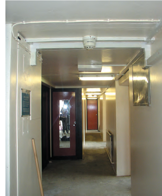
The corridors are tightly dimensioned, but have become cluttered with surface-mounted lights and services.
