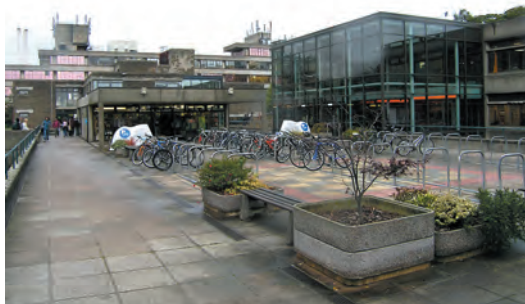
Walkway-level deck over shops, with new glazed link to Union House on right.
