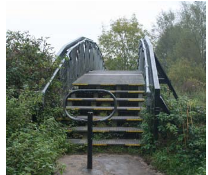
Below: Footbridge near south-west end of the Broad
