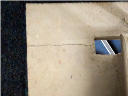
Crack in concrete landing
