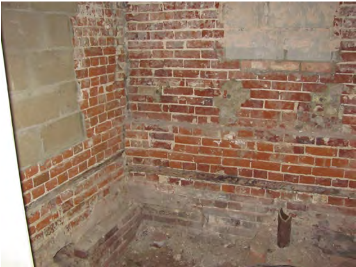
No floor and badly repaired brickwork
