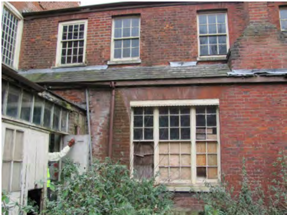
Missing flashing and gutter
