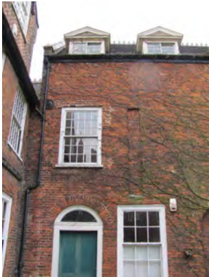
Plant growth over elevation and blocked gutter
