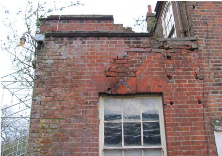
Window head dropped causing collapse of parapet
