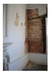
G1 damaged plaster and brickwork
