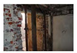
GF2 various props to lintels etc
