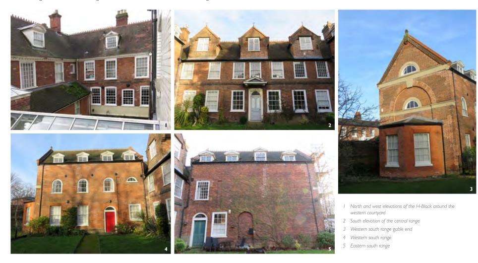
The nineteenth century buildings (the East Cell Range and the South-east Range) are generally plain: they demonstrate the pared back vernacular classicism of the period with shallow hipped or pitched slate roofs and regular sash windows. The now blank wall at ground floor level of the East Cell Range along Bethel Street, the windows in which were at high level anyway, is the only element that specifically reflects the building's use as hospital for the mentally ill.
