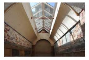
G6 view of panelling and removed plaster work
