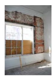
G1 damaged plaster and brickwork
