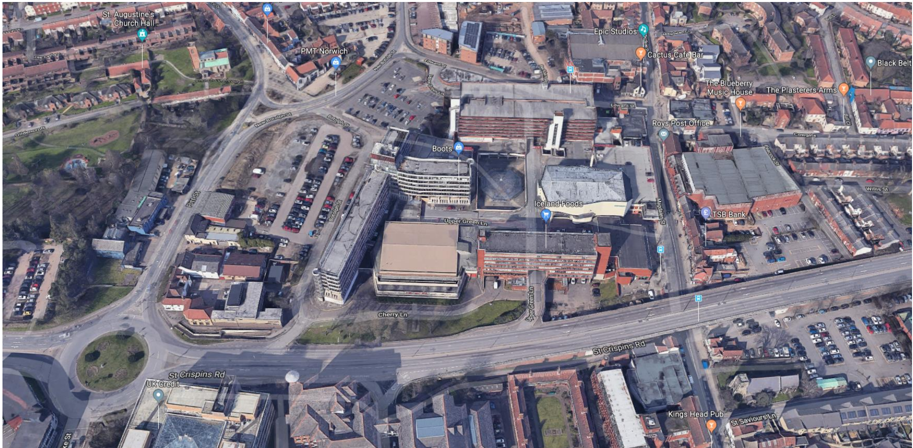
Aerial of Anglia Square from the South looking North
