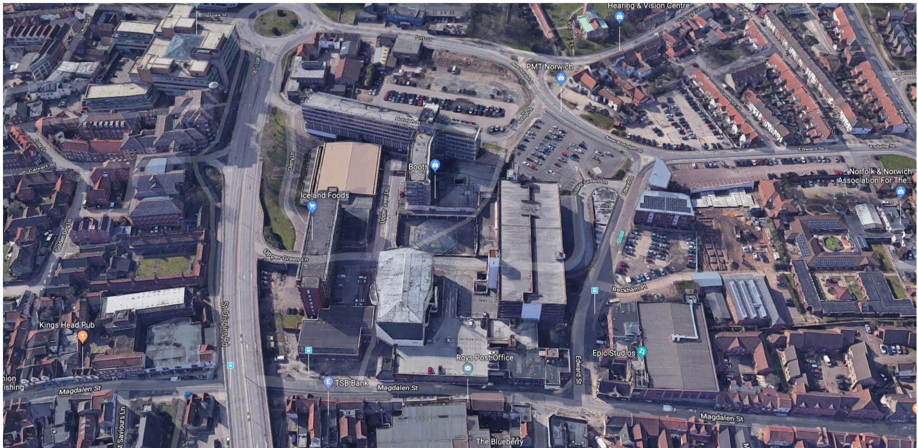
Aerial of Anglia Square from the East looking West
