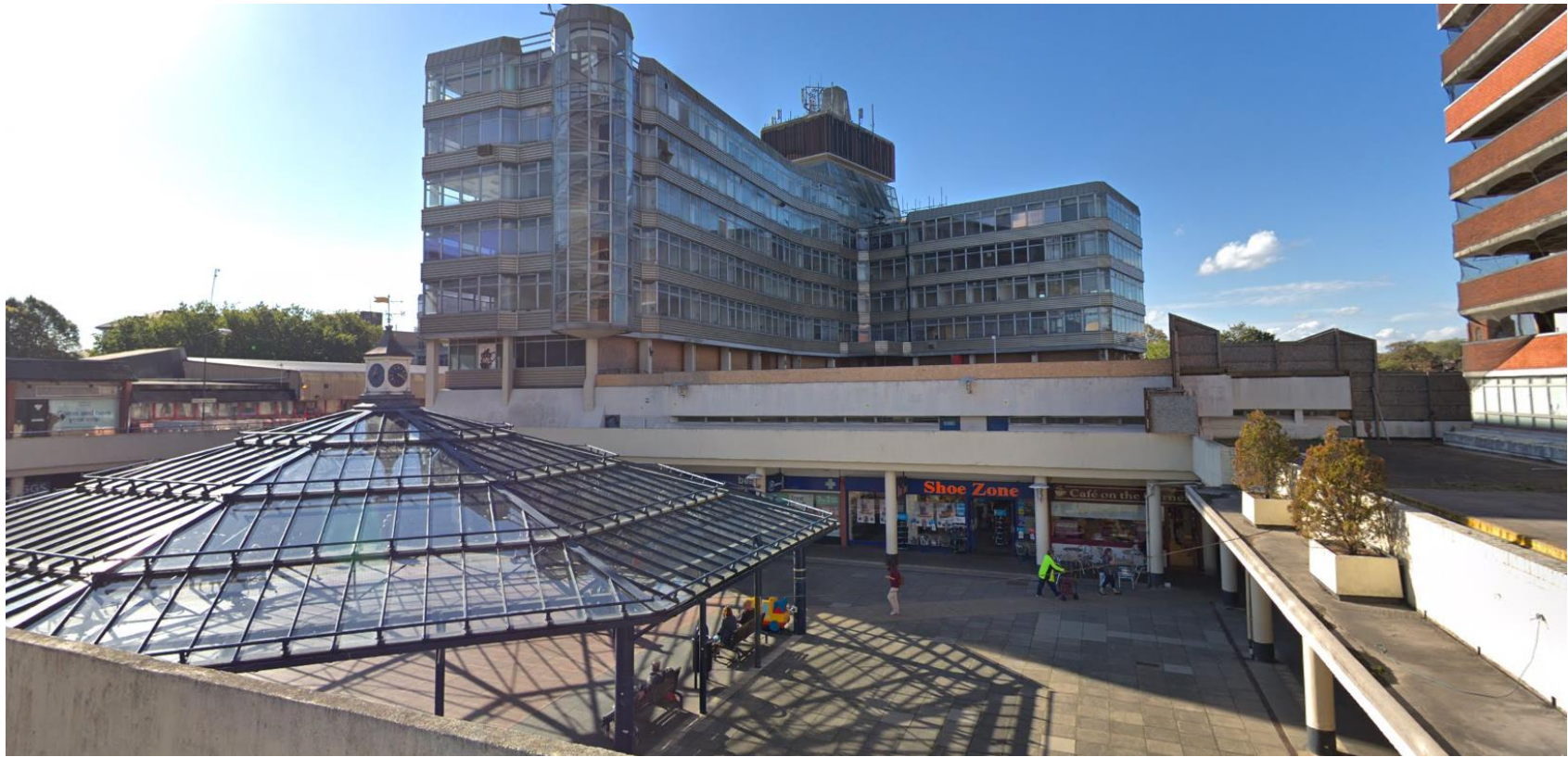
The Shopping Precinct from the deck level looking West
