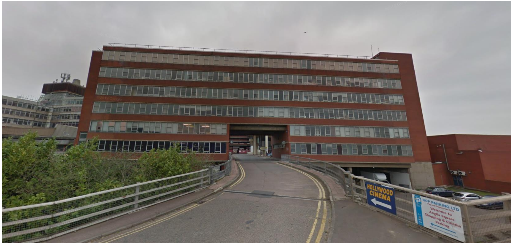
Gildengate House looking North
