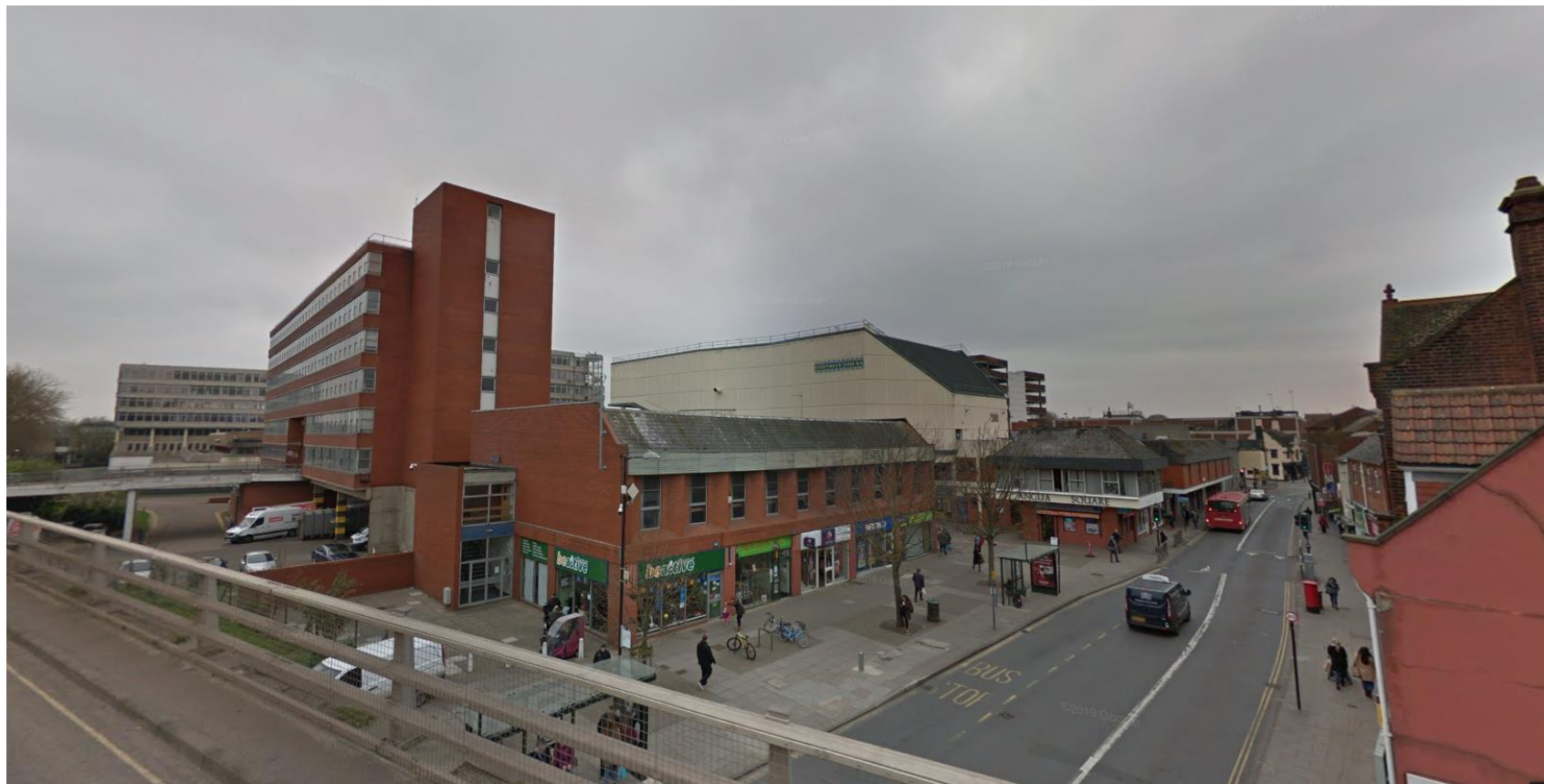
Anglia Square looking North West and North up Magdalen Street
