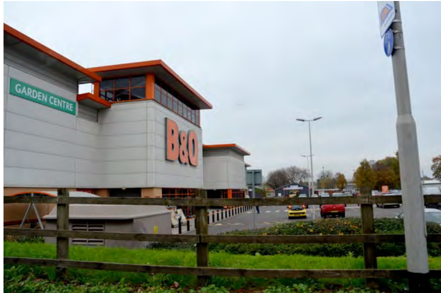
King's Lynn retail park: poor accessibility for pedestrians and cyclists, typical out of town architecture and large open car parks
