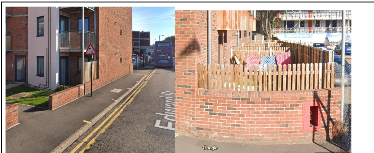
Figure 1 - Ground floor flats on Edward St close to receptor G and on the same road as receptor A. Notice the building facades and rear garden near to the road.
