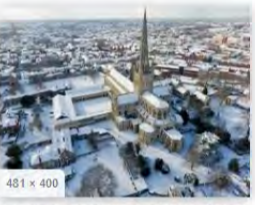
Locations and Grounds - Norwich School norwich-school.org.uk
