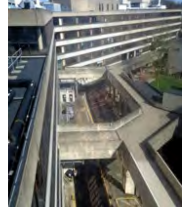
Primary access route via an external raised walkway on south side with bridge connections. (2018)
