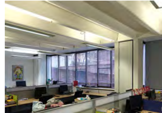
The Postgraduate Study Centre in the Academic Wall has opened up a formerly subdivided area, revealing Lasdun's precast concrete structure and floor slabs (which have unfortunately been painted). (2020)
