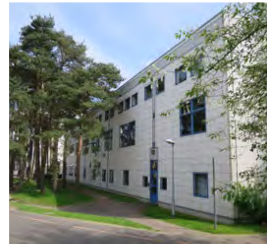
The blue windows and tiled north elevation of Mather’s Lawrence Stenhouse building [9]. (2006)
