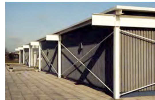
The Reliance Controls factory in Swindon (completed in 1966) was an early work by Team 4, where Norman Foster was a partner. It already displayed an architectural approach that used modern construction materials with exceptional clarity and precision.
