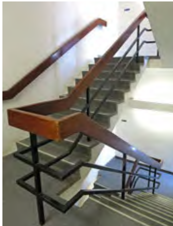
Wide stairs in service towers in Lasdun zones [3, 4, 6]. (2018)
