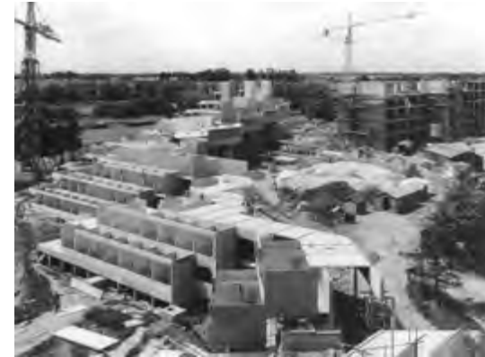
Construction in progress in 1965.
