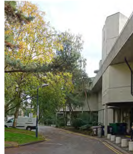
The north side of Suffolk Terrace. (2019)
