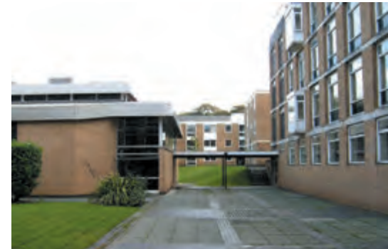
Lancaster University adopted a compact, high-density masterplan, but the buildings and layouts were bland by comparison with UEA. (2006)
