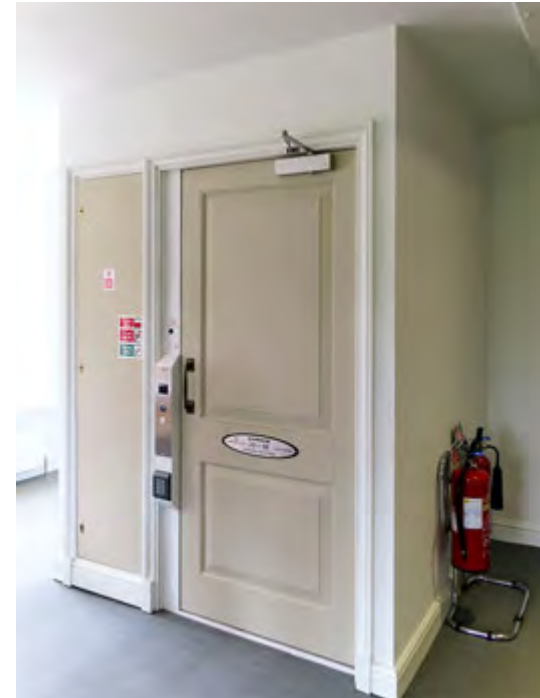
Disabled lift in Earlham Hall. (2018)
