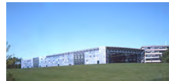
SCVA from the south, before the Crescent Wing was built. The long south-west elevation is largely blank. (1978)
