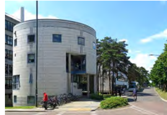
The Hubert Lamb building [8] acts as a landmark at the east end of Chancellor's Drive. (2018)
