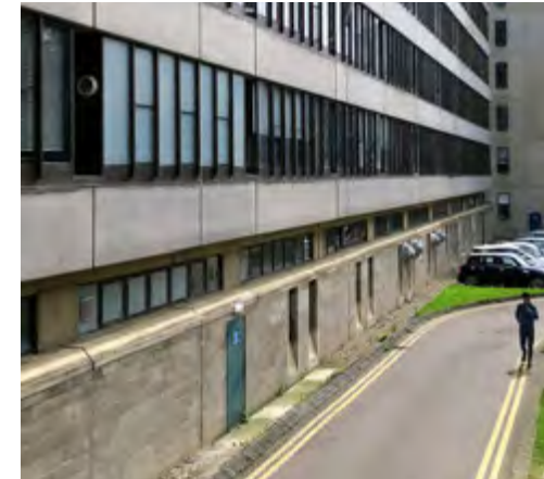
Blockwork external walls at ground level only. (2017)
