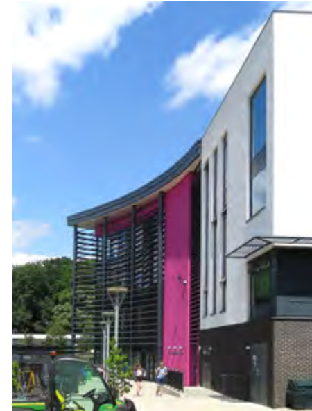
The Julian Study Centre [57], left, is connected to the Medical Building [43], right. (2017)
