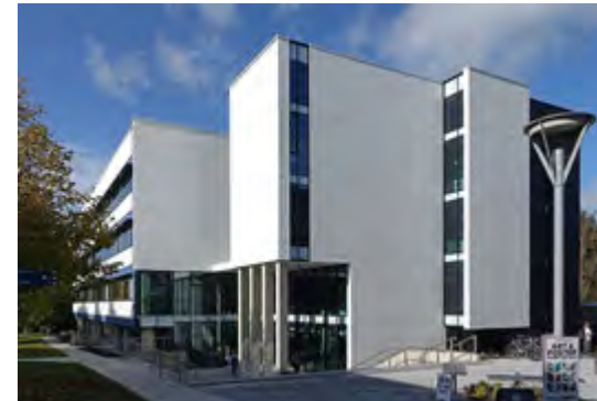
The Science and Engineering Teaching Building from the south-east [60]. (2019)
