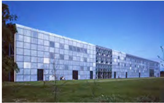
Both vertical and horizontal surfaces of 'tube' clad with solid, glazed, vent or door panels on uniform grid. (1978)
