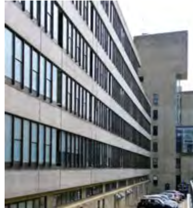
Continuous south facade; north facade (shown) interrupted by service towers.(2017)
