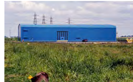
The Modern Art Glass building in a south London industrial estate, where Foster Associates accommodated multiple functions in a single all-enveloping container (completed 1973).
