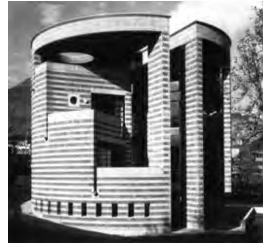
A design by Mario Botta showing the characteristic patterned and cut-away circular forms which he used in many projects from about 1980.
