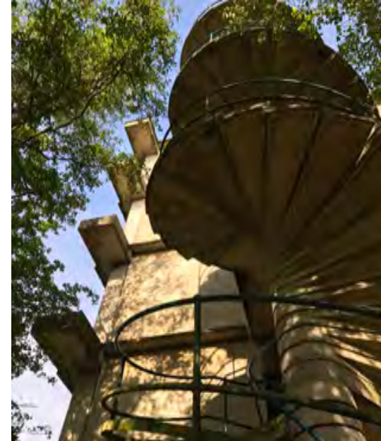
The ‘unfinished’ west elevation [6] of the Academic Wall with projecting nibs that were intended to link with a continuation of the building, and a ‘temporary’ spiral stair. (2018)
