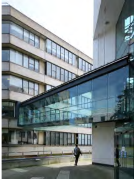
The bridge from ZICER [44] does not connect to an Academic Wall service core. (2018)
