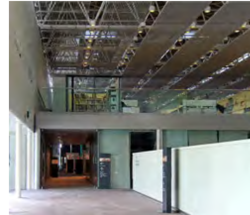
Two enclosures across full width of clear internal cross-section, with mezzanines over. (2017)
