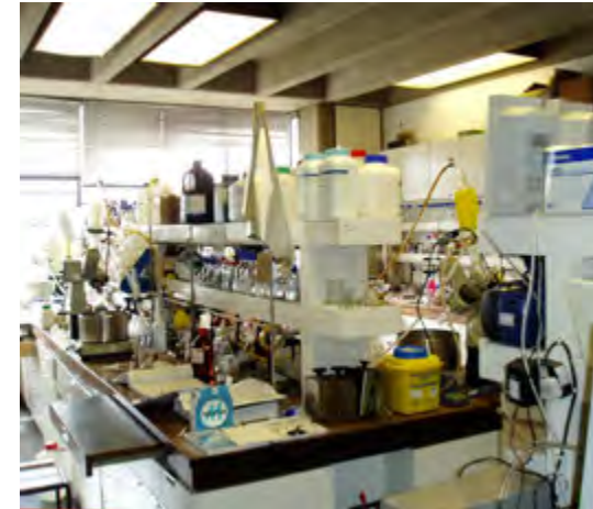
Few chemistry laboratories retain the original fittings of the 1960s. Note ceiling of exposed, unpainted precast concrete T-beams and original light fittings. (2006)
