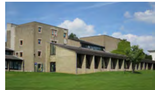
The Music Centre [21] by Arup Associates. The converted squash courts, now the Careers Centre [22], is the four-story building on the left. (2018)
