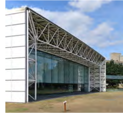
Extruded 'tube' of uniform cross-section with cut ends. (2018)
