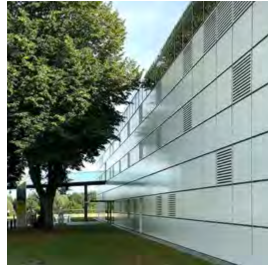
SCVA’s original cladding was corrugated, like the panels on a Citroen van (above), but the replacement cladding has a smooth white finish (below).
