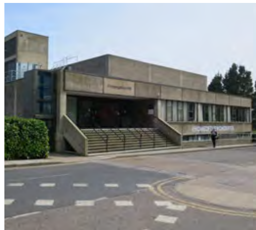
Congregation Hall [23] (former sports hall). (2018)
