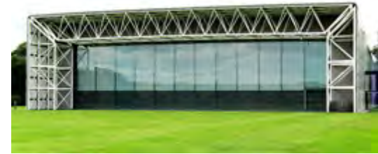
The exposure of the structural lattice at each end of SCVA hints at the 'separation of functions' tendency in high-tech architecture, whereas Foster's overall design strategy is to provide a continuous external envelope. Sealing and waterproofing between the lattice members is problematic. (2018)
