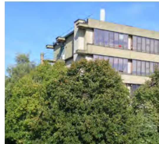
The ‘unfinished’ west elevation [6] of the Academic Wall with projecting nibs that were intended to link with a continuation of the building, and a ‘temporary’ spiral stair. (2018)
