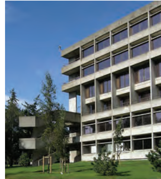
UEA's Library is a free-standing building with a deeply-modelled elevations of precast concrete panels. (2006)
