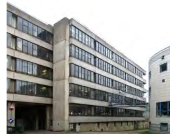
The north side of the Academic Wall at the junction between the original Lasdun Chemistry element [4] (left) and the F&M Sciences element [5] (right), where the building depth is greater than the original 50 ft (15.25m). The bridge link to the Humbert Lamb Building [8] (far right) cuts into the Academic Wall elevation. (2018)
