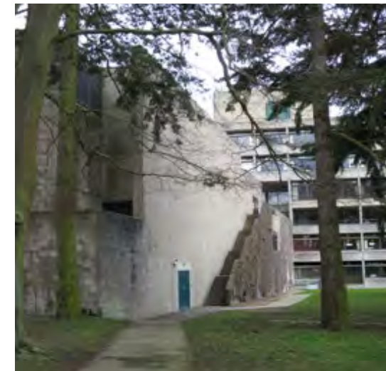
The blank south-west elevation of the Lecture Theatre block [13], facing the harbour. The external stairs to the Library [14] walkway are little used. (2018)
