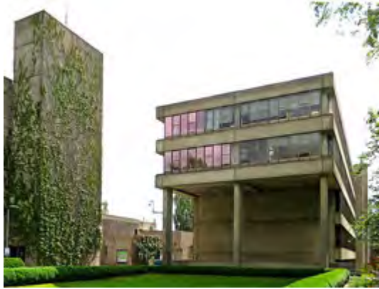
East end [3] of Academic Wall has a finished elevation. (2017)
