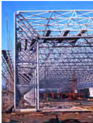
Vertical and horizontal structure forming lattice of 2.4m depth, defining clear internal cross-section. (1977)
