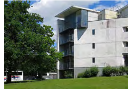
The west end of Constable Terrace (1992-93) is modelled to act as a landmark to Chancellor's Drive, but is now largely hidden by trees. (2017)
