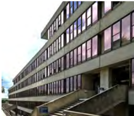
Alternating bands of glazing and precast concrete spandrel panels of uniform design on south and most of north elevations. (2017)
