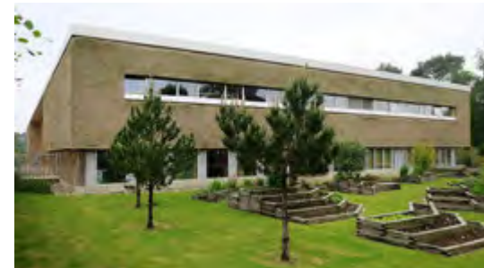
The Enterprise Centre has thatched cladding; view from the north [58]. (2018)
