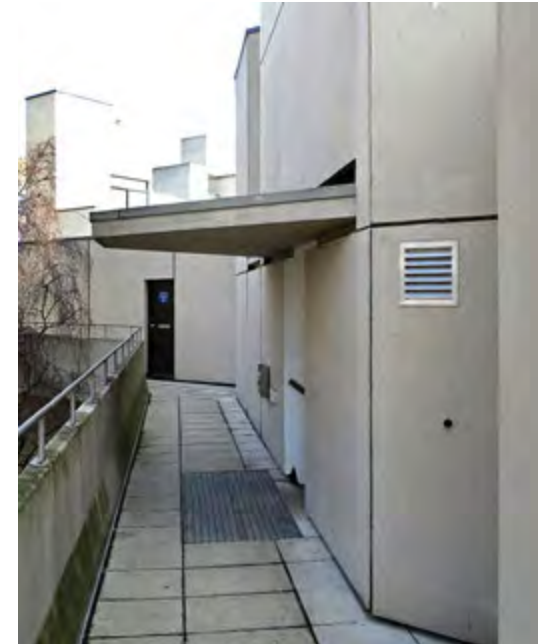
High-level walkway on the north side of Norfolk Terrace [106]. The walkway is an integral part of the ziggurat structure, unlike the Academic Wall walkway which is an independent structure (2018)
