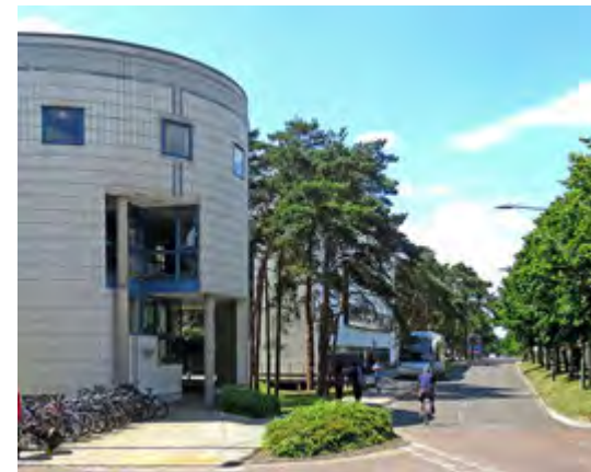
The Hubert Lamb building of 1984-85 adopts a circular form with cut-away sections, seen in Mario Botta work. Chancellor's Drive continues to the west. (2017)
