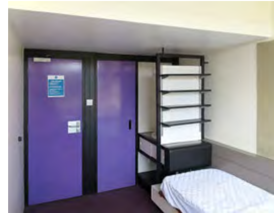
The refurbished study-berooms in the zigurats retain the character of the original design. The change in ceiling level between the front and back parts of the room can be seen. (2018)
