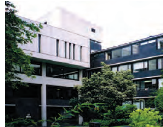
Lasdun argued that, over time, the dark brick-clad parts of the Royal College of Physicians building would change more than the white mosaic-clad parts. (2006)
