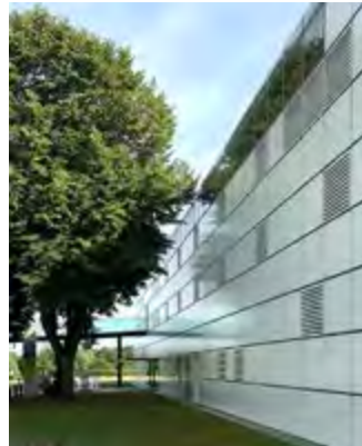
Minimal disruption to smooth face of 'tube' (bridge and entrance canopies only). (2018)
