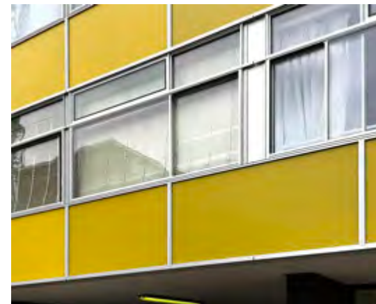
When the slender single-glazed aluminium windows of Grade II listed Great Arthur House in the City of London, designed by Chamberlin Powell & Bon and completed in 1957, required replacement, a glazing and curtain walling system was developed that incorporated double glazing and retained the slender window profiles. The replacement was completed in 2019.
