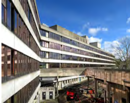
Linear building approx. 15m wide by 400m long with three 45° cranks and three steps. (2018)
