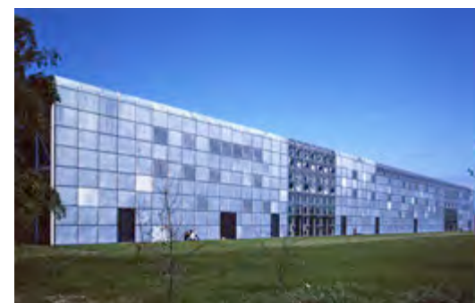
The south-west elevation of the SCVA with the original corrugated aluminium cladding panels. (1978)
