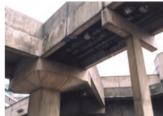
The dramatic concrete world under the Teaching Wall walkways. (2006)
