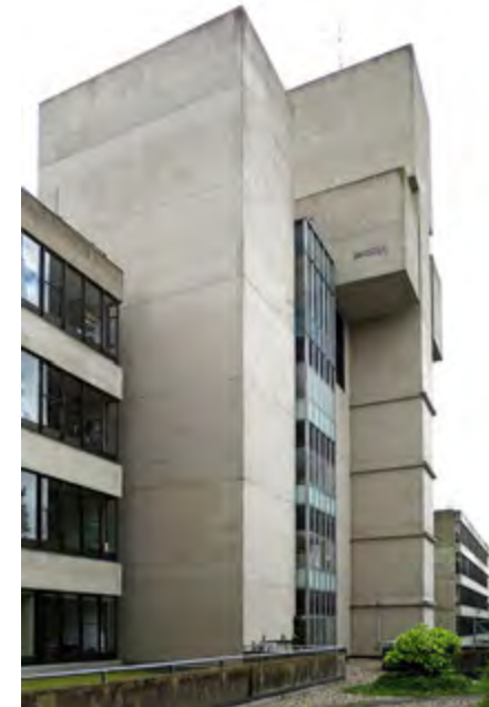
The north elevation of the Academic Wall is punctuated by the giant service cores. (2018)
