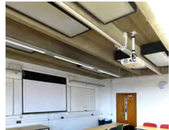
Mixed conservation achievements – here original lights retained and precast concrete unpainted, overlaid by non-original features (Lasdun zone [3, 4, 6] shown). (2018)
