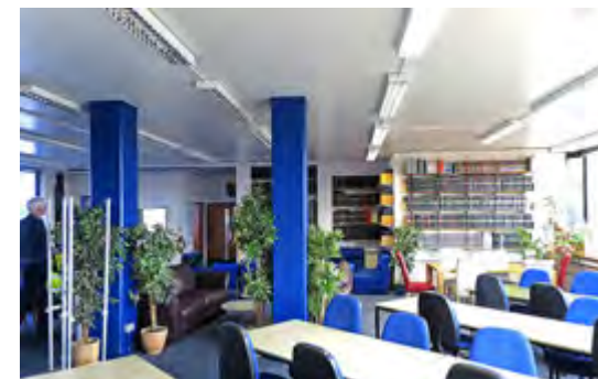
Open floor in the Academic Wall without non-structural partitioning, in a Feilden & Mawson element, indicated by flat insitu slab not precast ribs. (2018)
