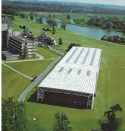
Separation between SCVA and neighbouring buildings. (1978)
