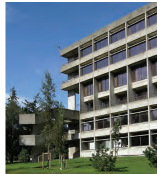
Library [14]: south-west elevation. This part of the building was completed in 1974. (2006)
