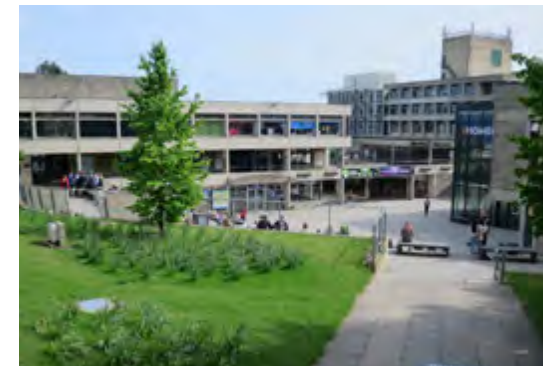
The square, with the Union House [17] on the left, Restaurants [16] on the right and the Library [14] at the back. (2018)
