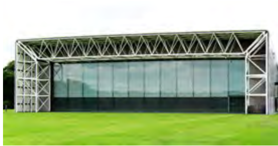
At cut ends of 'tube' the structure is exposed with glazing set back to the dimension of the clear internal cross-section. (2017)
