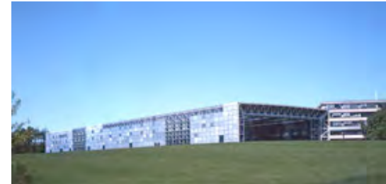
View of the original SCVA from the south, before the Crescent Wing was built. (1981)
