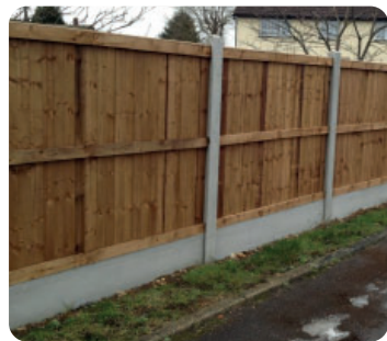
Timber feather-edge fencing with concrete posts and gravel boards
