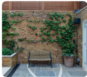
Use of multi-tone or reclaimed bricks to reflect urban grain and reference the lighter tones of Cambridge buff brick
