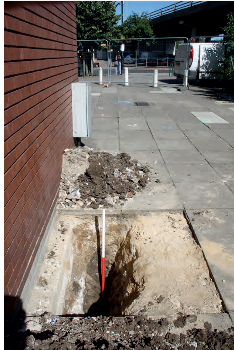
Plate 2: Test Pit 5, looking east
