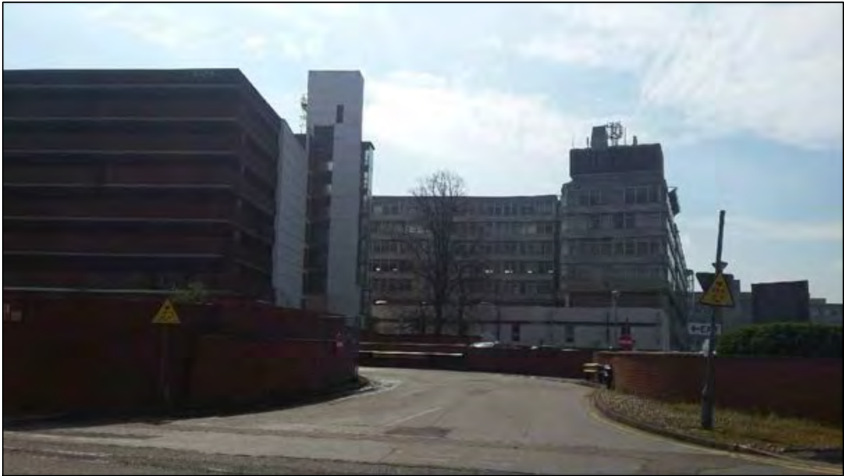
Plate 3: View of northern access road, facing south
