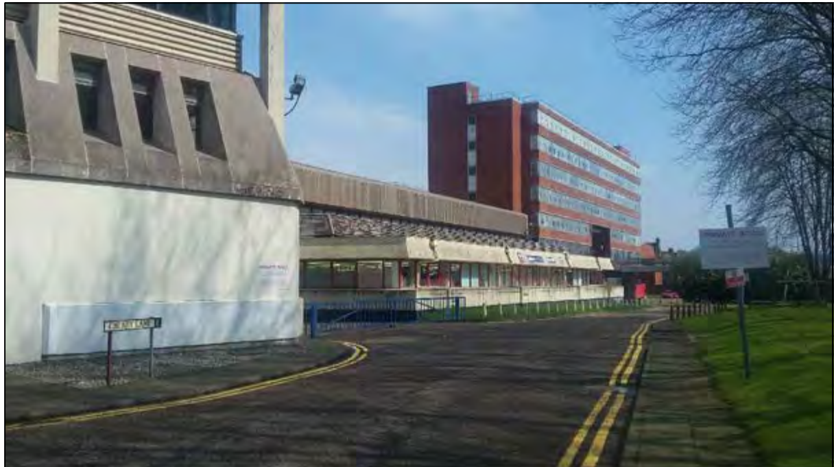
Plate 10: View of buildings in south of site, facing northeast
