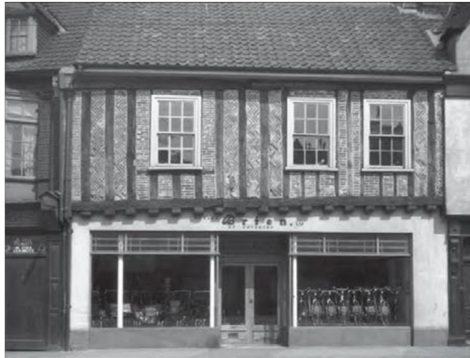
1990s wirecut brickwork
