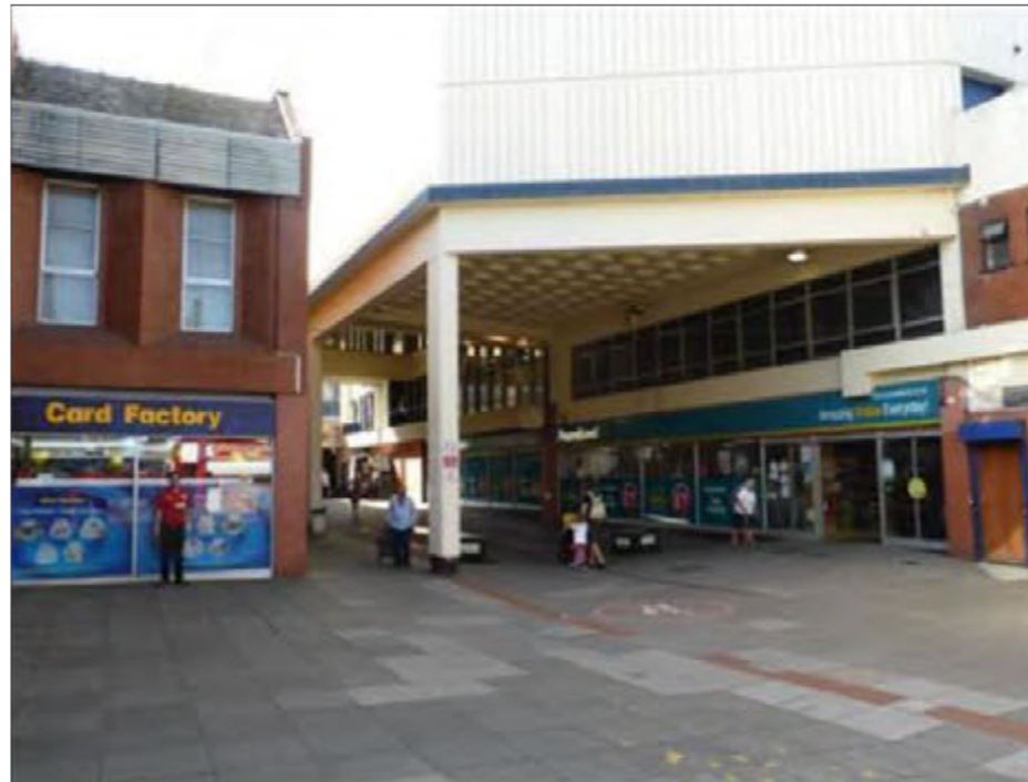
1990s wirecut brickwork
