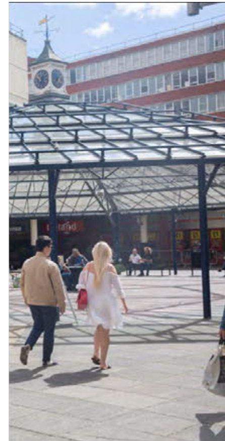
Brick detailing on Montefiore Hospital
