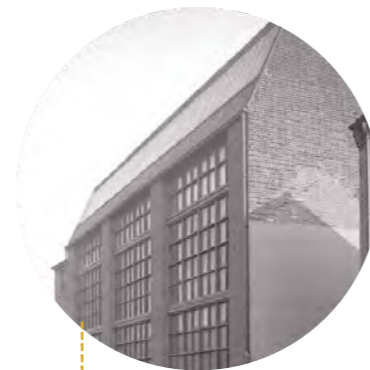
Full bay window (industrial character)
