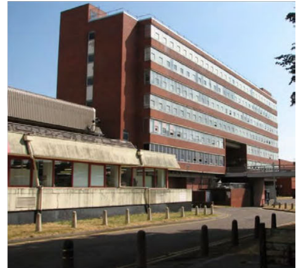
1930s Brick corbelling detailing
