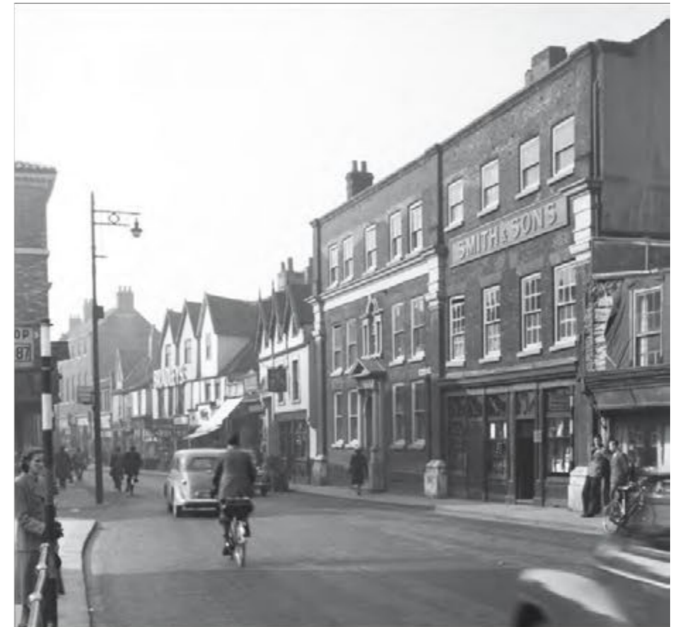
1930s Brick corbelling detailing
