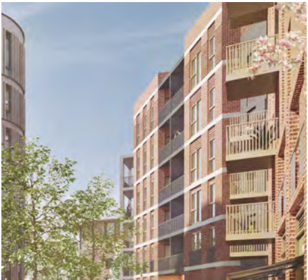
Bolt on Balcony in a Recess Example
