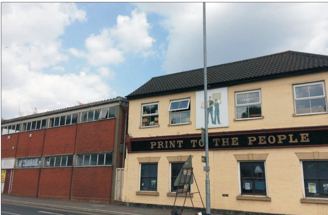
PHOTOGRAPH 12: Building B11 and Building B12
