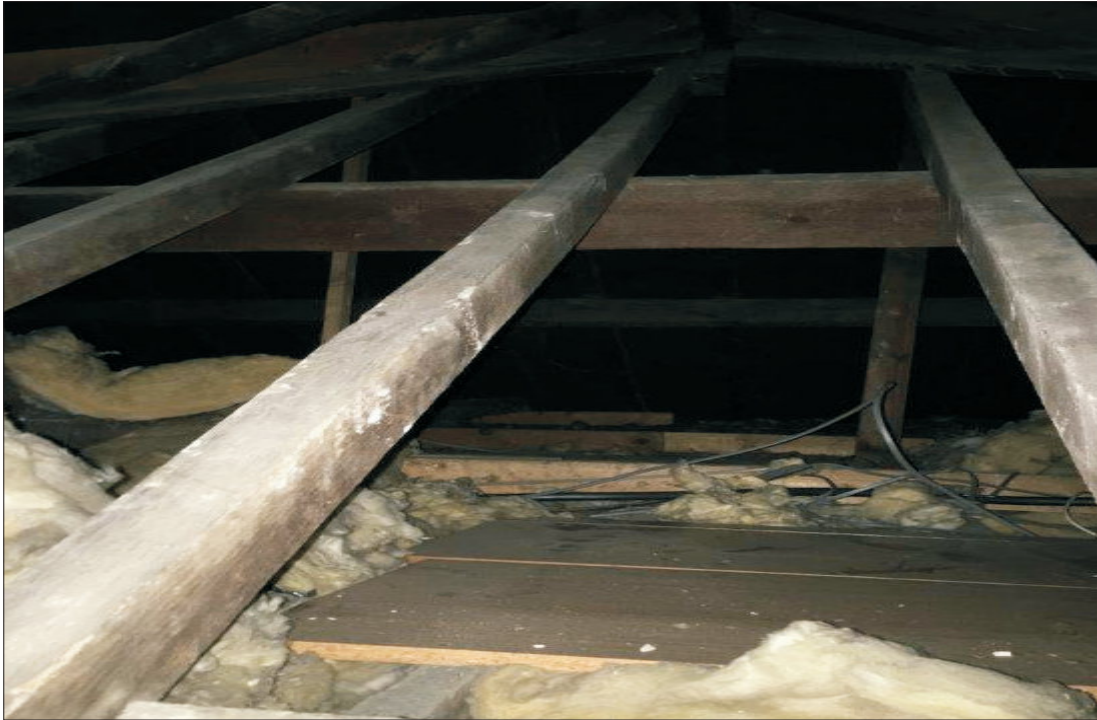
PHOTOGRAPH 9: Loft space of Building B8
