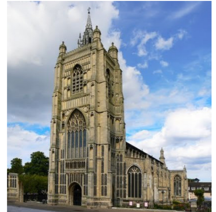
Figure 5.6 Church of St Peter Mancroft from the SW Source: CgMs
