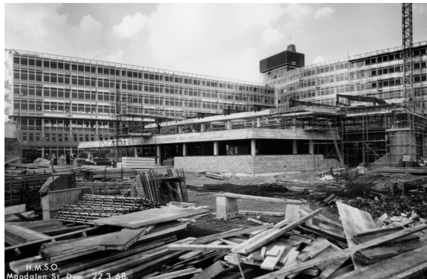
Figure 4.13 Construction of Anglia Square, 1968 Source: Reg Walker
