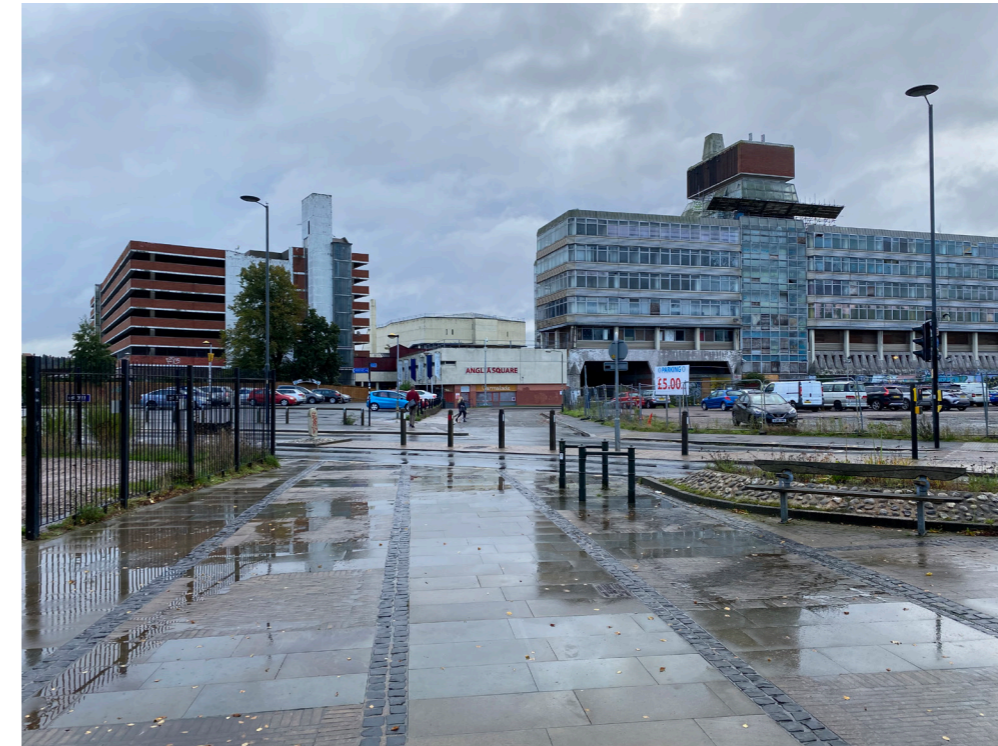
Figure 4.29 Looking towards Anglia Square from the northwest. Buildings, left to right: Multi-storey car park, Hollywood Cinema (in the background), and Sovereign House
