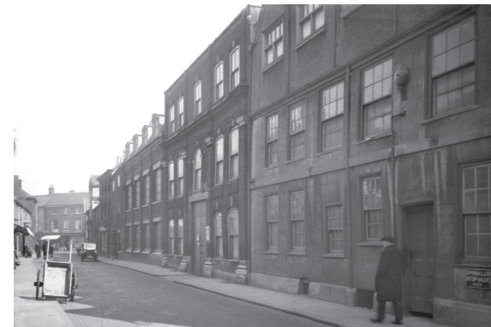
Figure 4.6 Looking north towards 63-65 Pitt Street in 1936. No 65 (the building with the large central doorway), was a C18 house that was converted into a shoe factory during the nineteenth century Source: George Plunkett's Photographs
