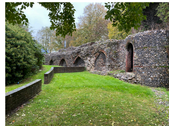
Figure 5.4 Portion of Norwich City Walls
