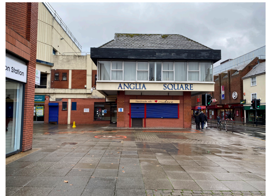
Figure 4.34 Entrance to Anglia Square on Magdalen Street
