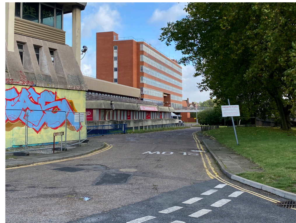
Figure 4.33 Looking southeast towards Gildengate House. Sovereign House is in the foreground
