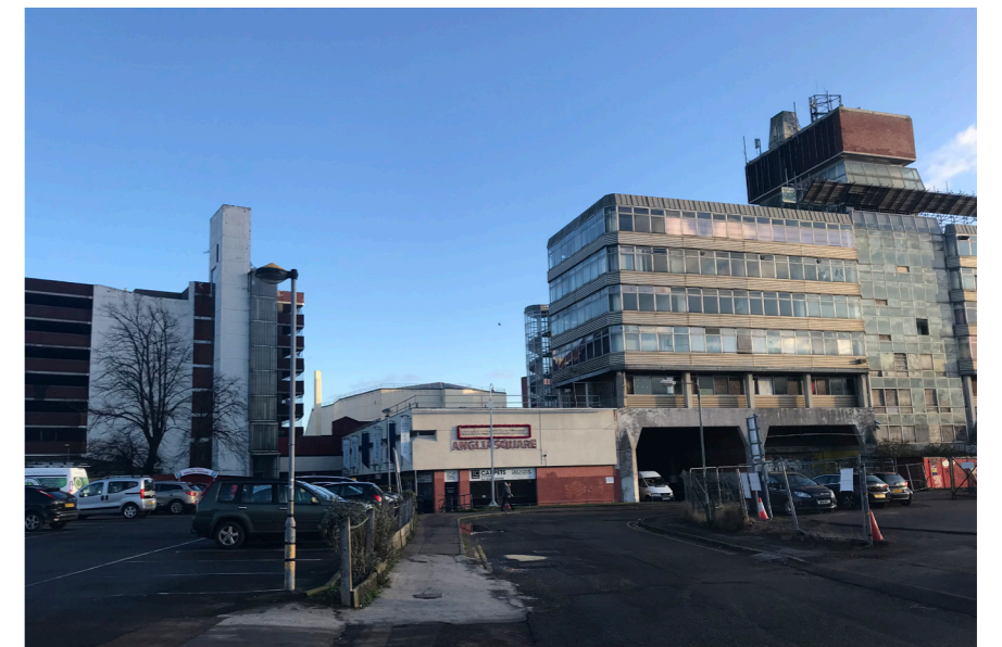
Figure 5.34 Anglia Square surface car parking, the multi-storey car park (left) and Sovereign House (right)
