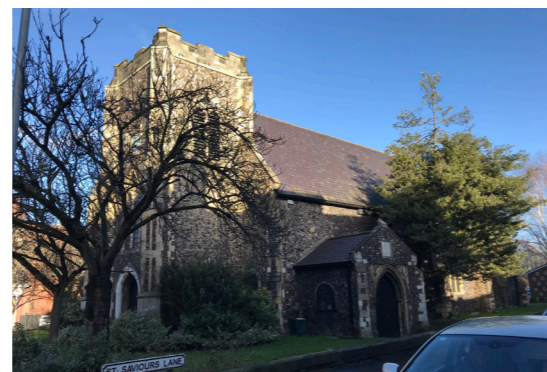
Figure 5.36 St Saviours Lane, Norwich
