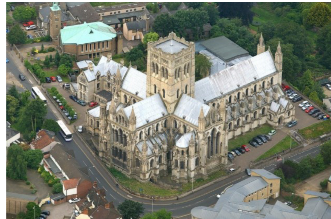
Figure 5.17 Aerial view of the Roman Catholic Cathedral from the northeast Source: CgMs
