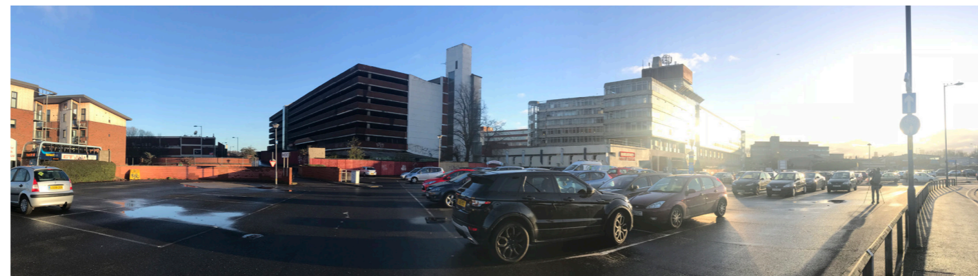
Figure 5.28 Panoramic photograph of Anglia Square from the west
