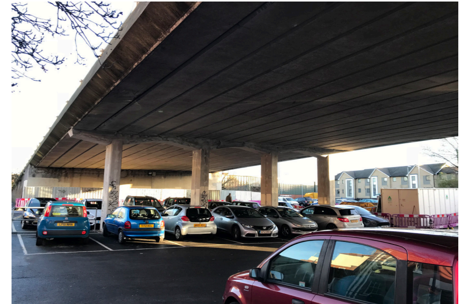
Figure 5.31 Car parking beneath St Crispin's flyover
