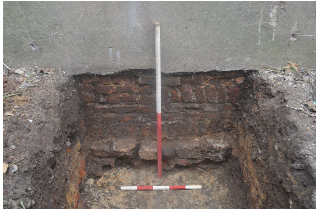
Figure 1: East facing of Test Pit 1 showing exposed limestone foundations.
