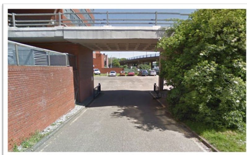
Figure 2: Underpass on Cherry Lane (Source: Google Maps)
