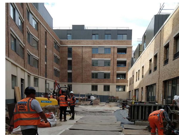
A podium landscape under construction.
