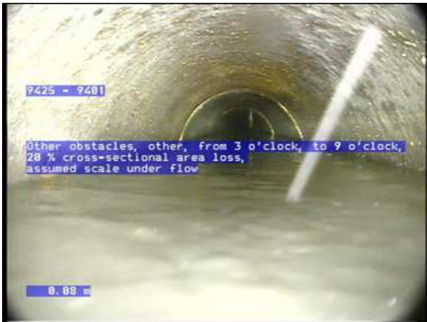
Photo: 36_36_254_A.jpg, 00:00:46 0.08m, Other obstacles, other, from 3 o'clock, to 9 o'clock, 20 % cross-sectional area loss, assumed scale under flow
