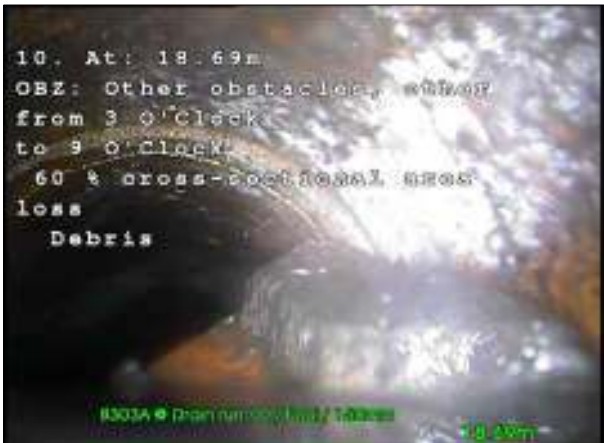
Photo: 21_21_153_A.jpg, 00:02:04 18.69m, Other obstacles, other from 3 O'Clock to 9 O'Clock 60 % cross-sectional area loss Debris
