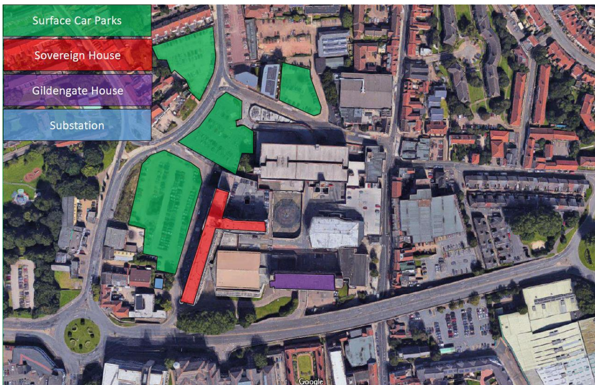
Figure 2 – Highlighted Existing Assets within the Site
