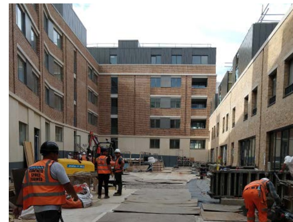
A podium landscape under construction.
