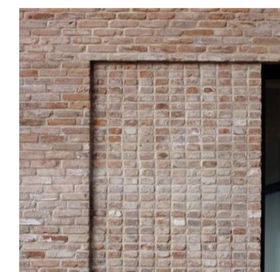
Detail 03c Recessed brick panel: Header courses
