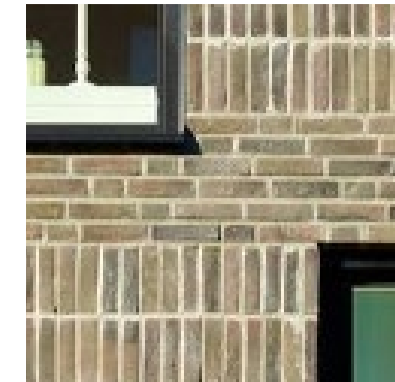
Detail 01b Linear band: Double soldier course
