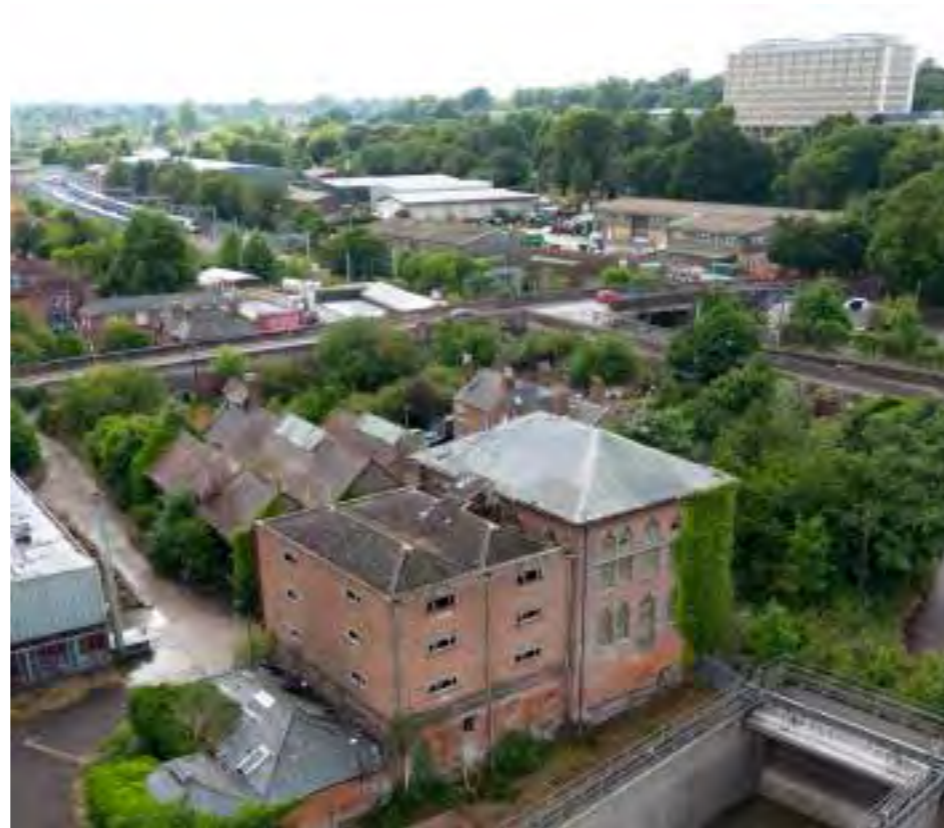
Trowse Pumping Station
