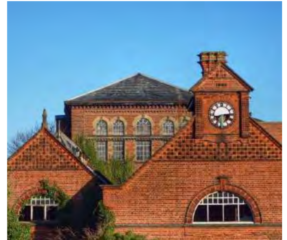
Trowse Pumping Station
