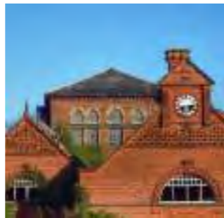
Trowse Pumping Station
