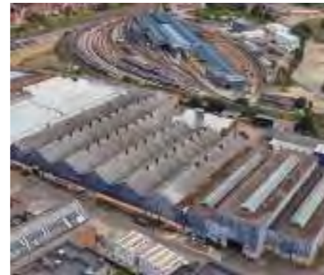
Industrial warehouses north of river
