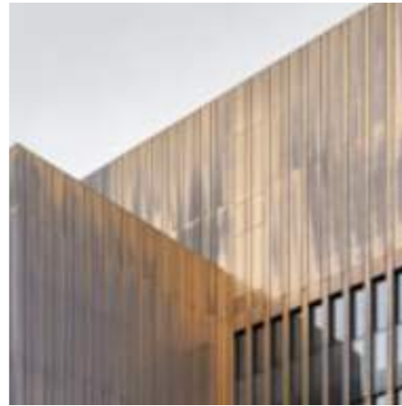
C1 - Metal cladding/roofing
