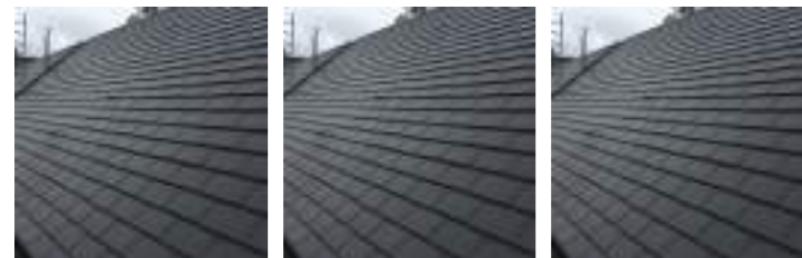
RF05 - Slates RF05 - Slates RF05 - Slates
