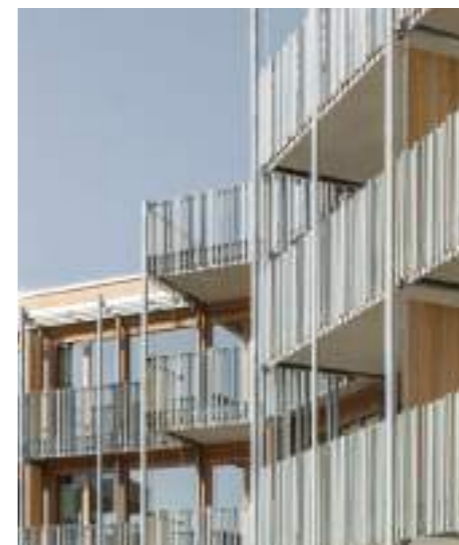
Projecting deck access Strong material character
