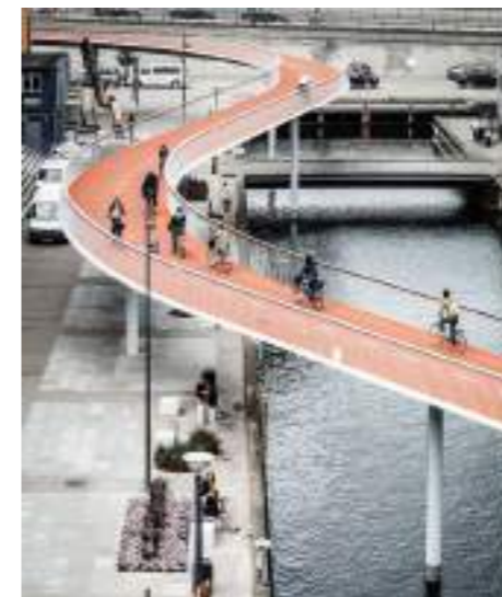
Pedestrian/cycle bridge. Simple coloured surface clearly identifies bridge deck
