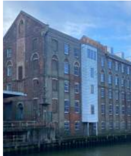
Local projecting bay over river.
