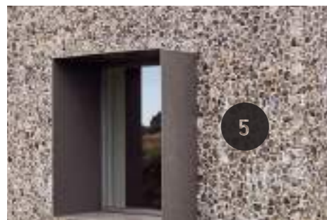
Cobbled wall section
