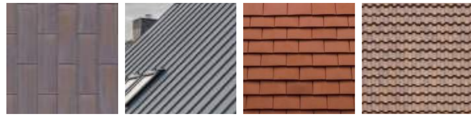
RF01 - Pigmented zinc RF02 - Natural zinc RF03 - Roof tiles RF04 - Pan tiles
