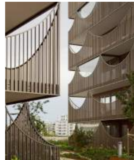
Continuous balconies: This simple building is interesting for it's sweeping balcony design
