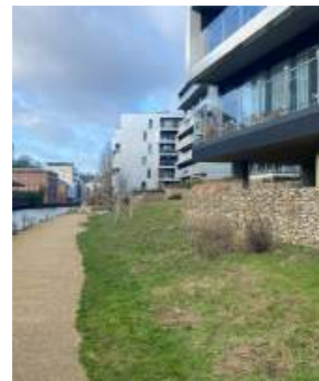
Gabions conceal parking
