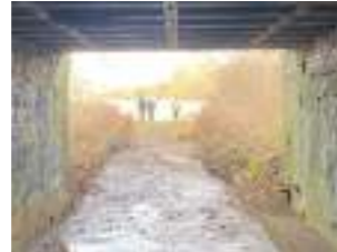
Site photo of the underpass
