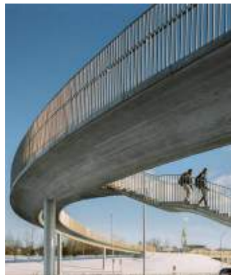
Pedestrian/cycle bridge. Hringbaut, Iceland. The bridge provides both stepped and sloped access and compliments the natural environment.
