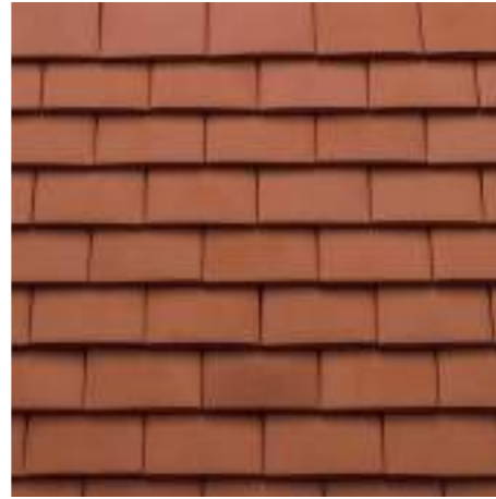
R1 - Roof tiles
