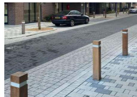
5. Bollards and 20mm kerb demarcate edge of road.
