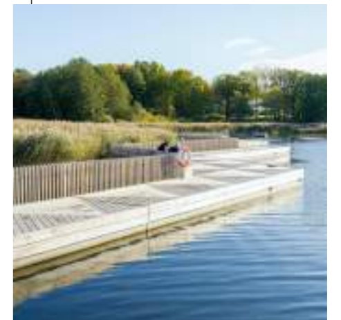
Floating pontoon / moorings possibly as part of the bridge fender
