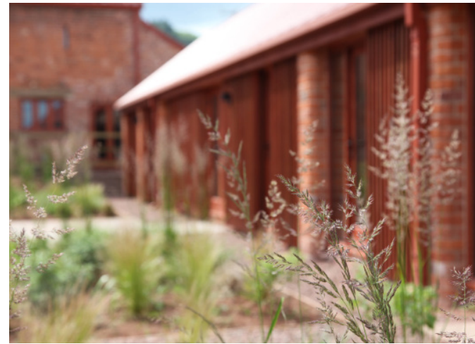
Vertical baffles used within The Parks, Stolon Studio
