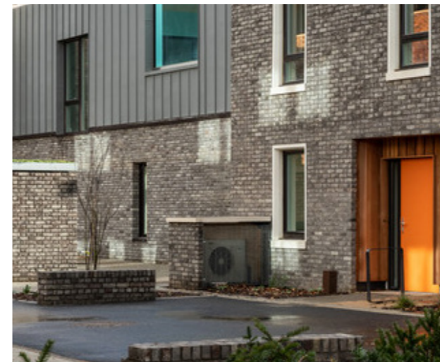
AHUs in dedicated housing at front of terraces
