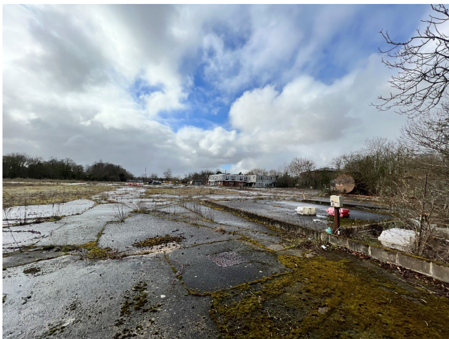
Photo 3: View of May Gurney Site, looking south-west
