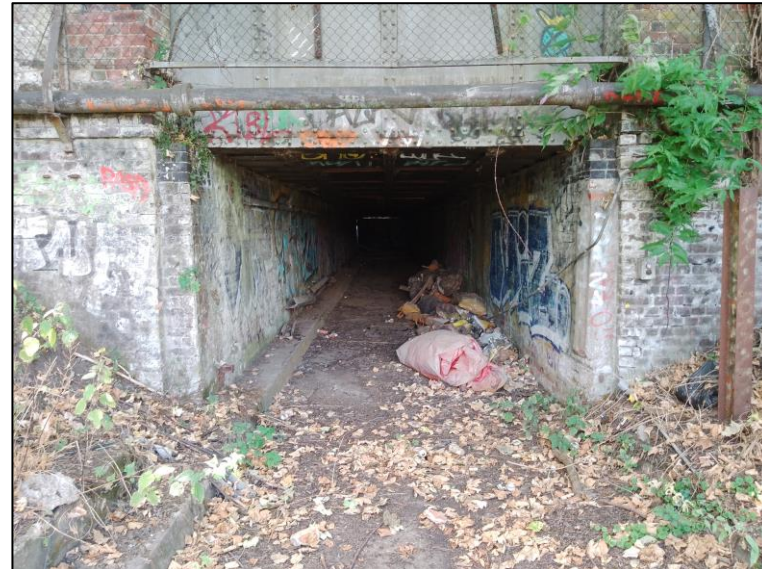
Photograph 12: Former Colemans Subway Tunnel (B6)
