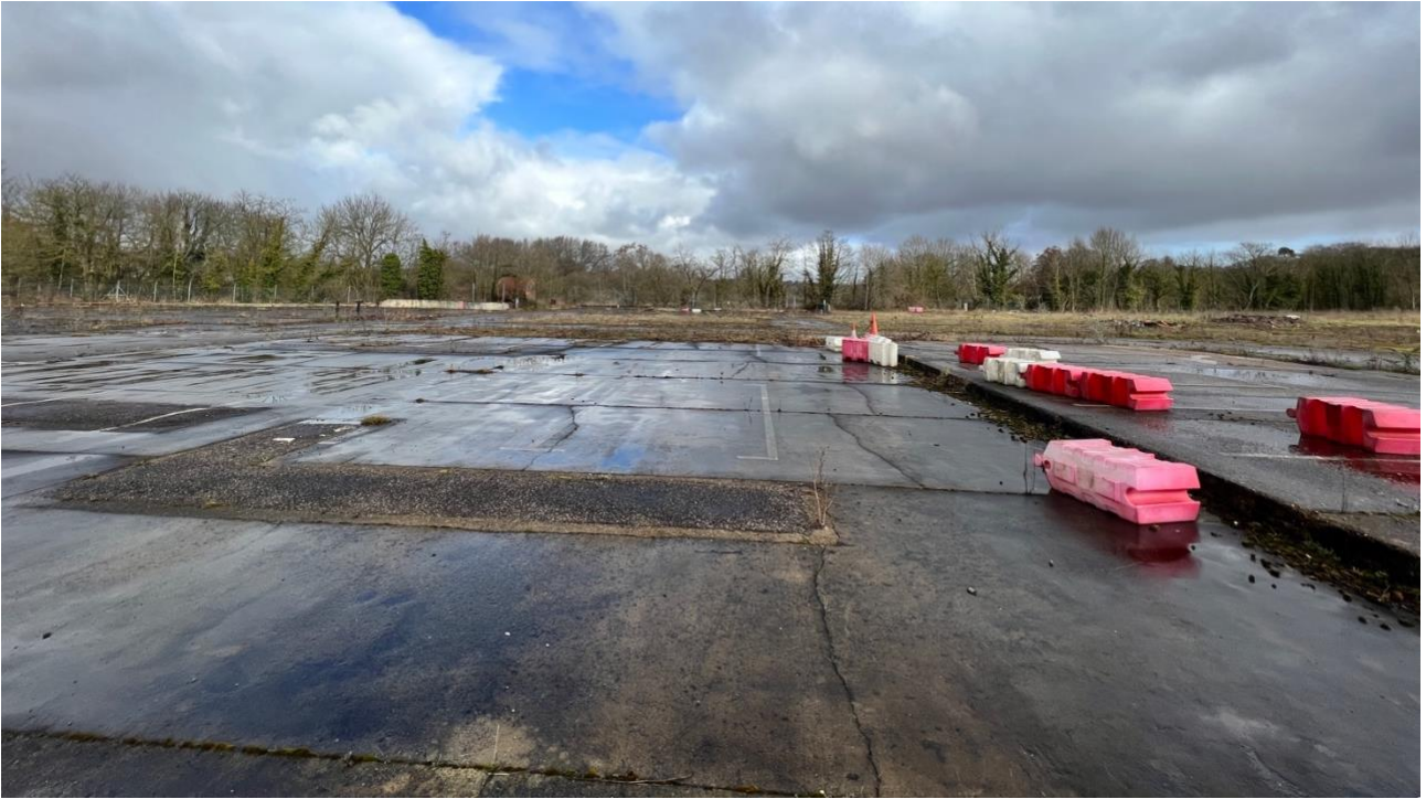
Fig. 26: View north from within the Site.
