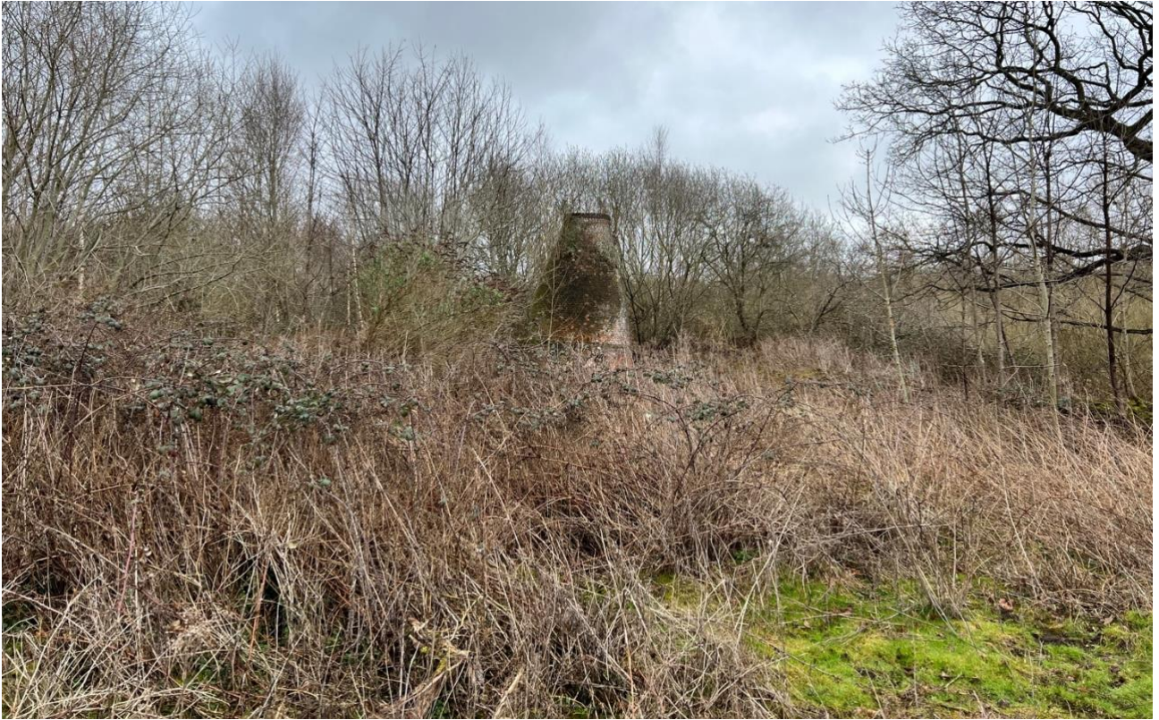
Fig. 35: View south-east from within the Deal Ground portion of the Site towards the grade II listed bottle kiln, currently screened and hidden by scrub.
