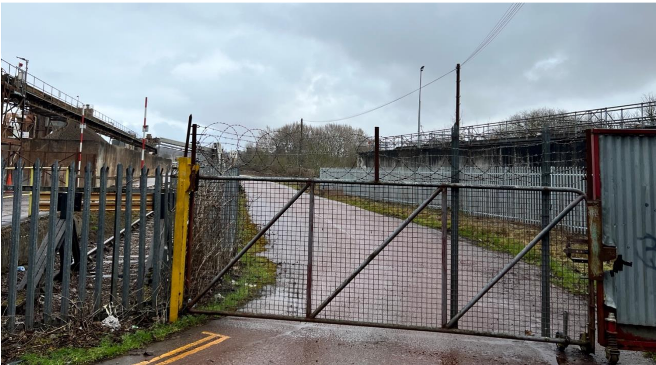
Fig. 29: Secondary entrance/shared access to yacht club. Trowse Depot to the left side of the access road, western side boundary on the right side.
