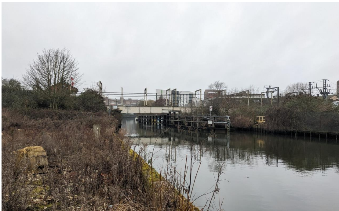
Figure 6 – Photograph of Trowse Rail Bridge taken from north-west corner of the site
