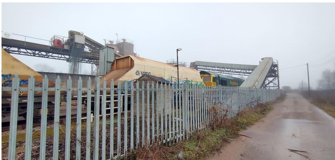
Figure 19 – Photograph of cars at railhead during delivery and hopper dropping asphalt
