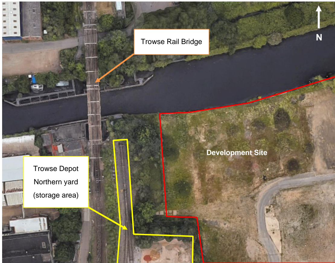
Figure 5 – Annotated aerial photograph of Trowse Rail Bridge Location © Google 2023
