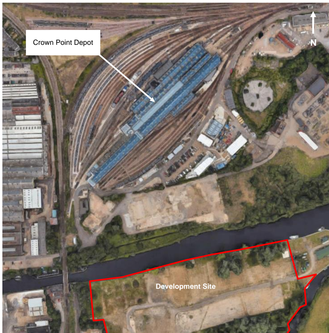
Figure 7 – Aerial photograph showing location of Crown Point Depot © Google 2023
