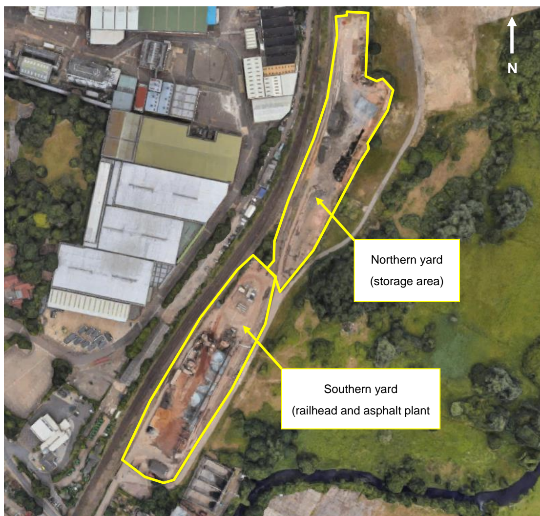
Figure 4 – Aerial photograph showing the location of the Trowse Depot © Google 2023
