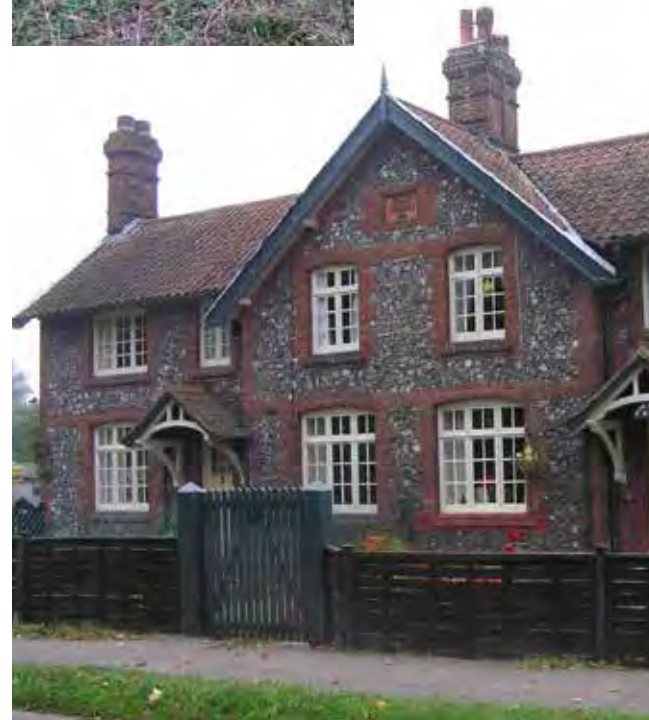
Distinctive Colman estate cottages reflect the availability of flint from local chalk workings. Alison Yardy
