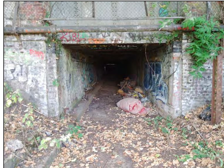
Photograph 12: Former Colemans Subway Tunnel (B6)
