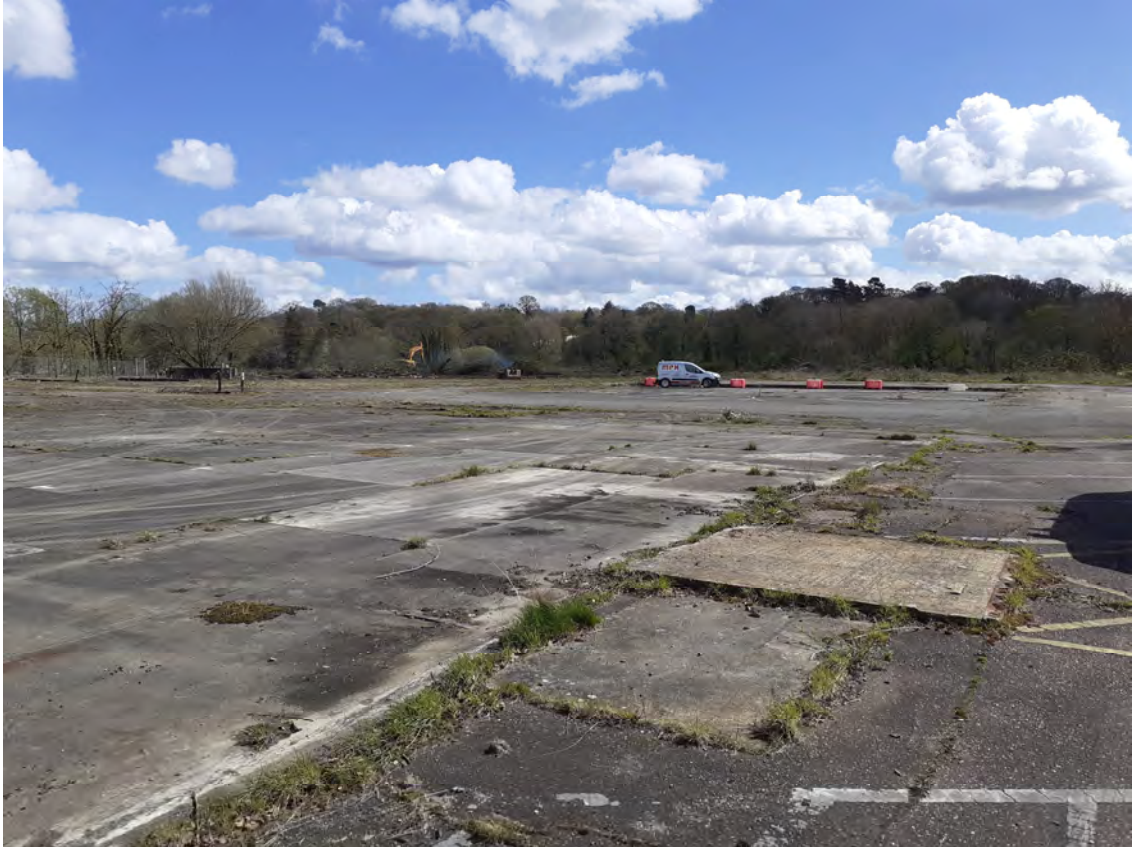
Photograph 26: View to the north east
