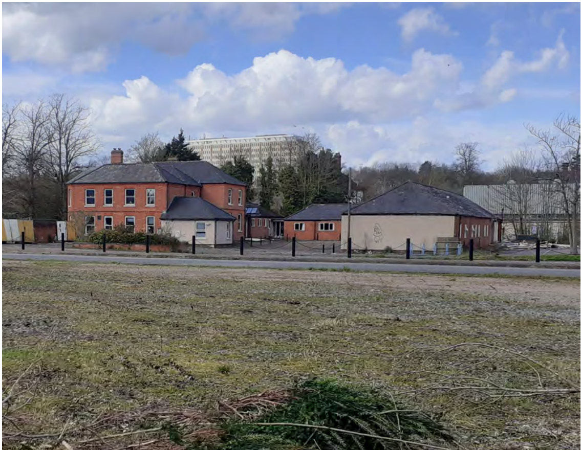
Photograph 19: Office buildings in the south west corner.
