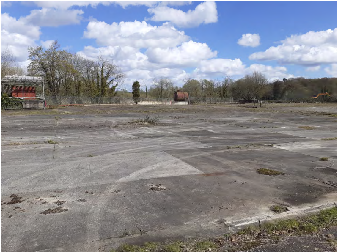
Photograph 25 : Land to the north of the office building. Two large diesel tanks close to the northern boundary.
