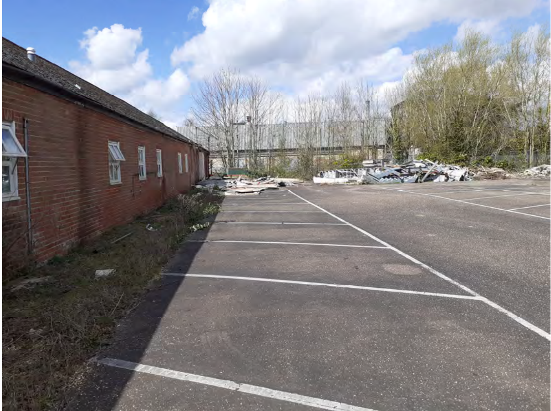
Photograph 20: Heating oil tank and scrap to the north of the buildings in the south west corner.
