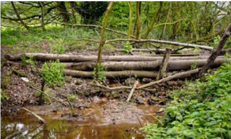
Figure 3.7 Traditional NFM structures, such as leaky barriers, can be used to enhance channel-floodplain connectivity to encourage nutrient deposition
