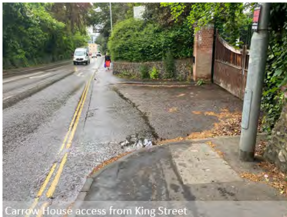
Carrow House access from King Street
