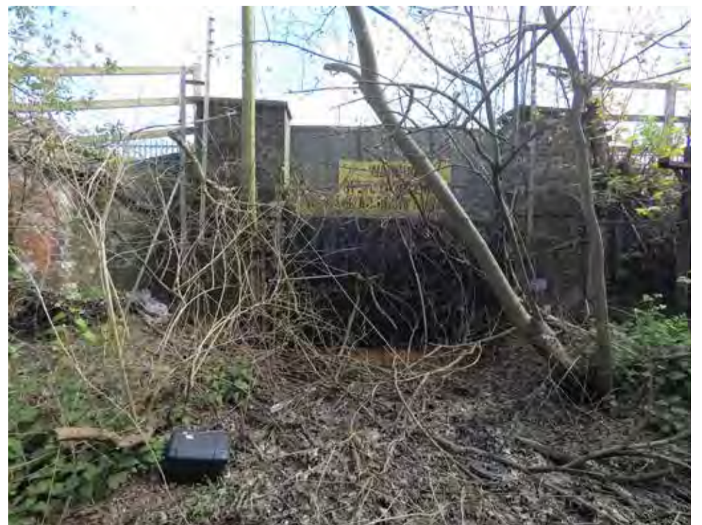
Underpass tunnel entrance on the Carrow Works Site.
