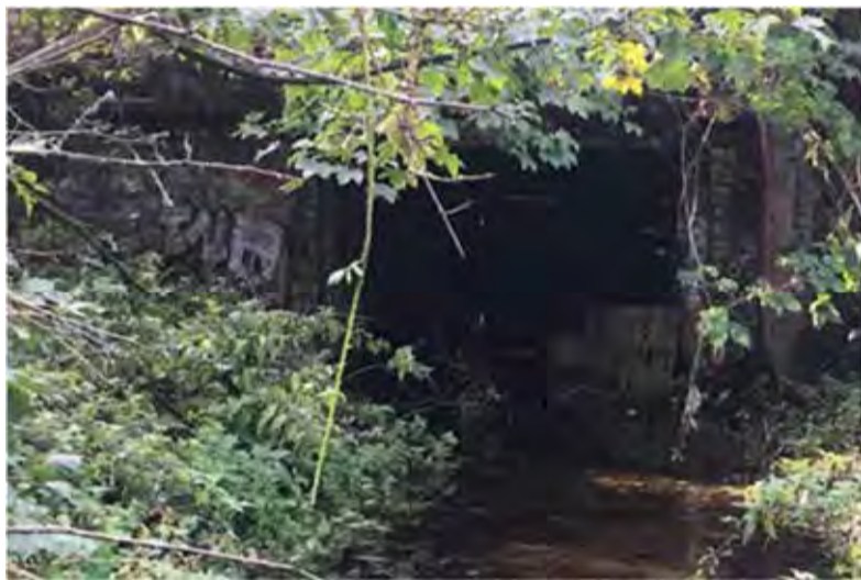
Figure 4-10 - Existing Railway Underpass - East Elevation
