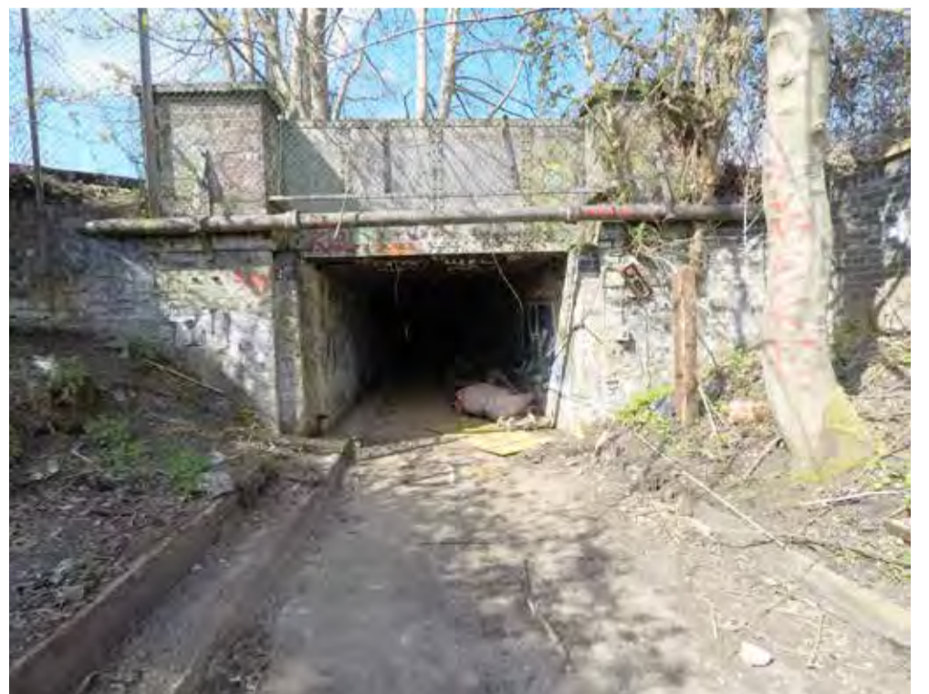
Underpass tunnel entrance on the Deal Ground.
