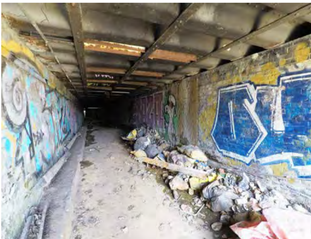
Underpass tunnel from the East entrance on the Deal Ground.
