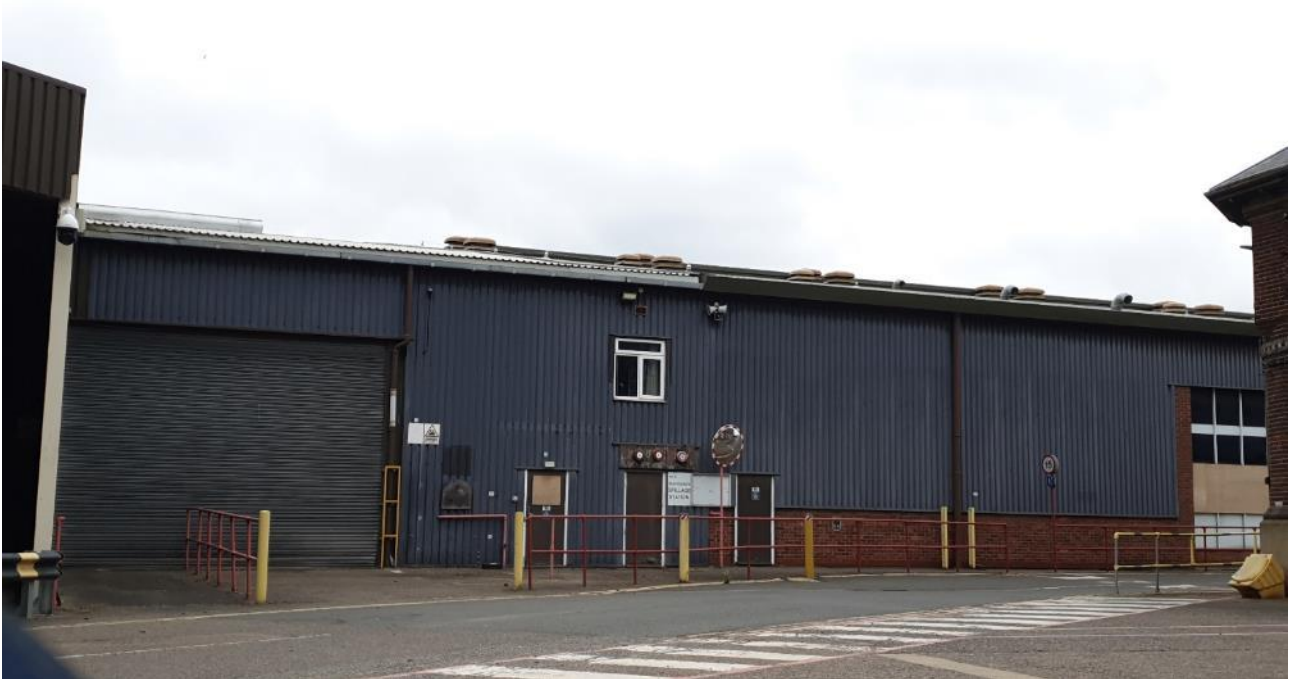
Figure B.18 Factory buildings on site
