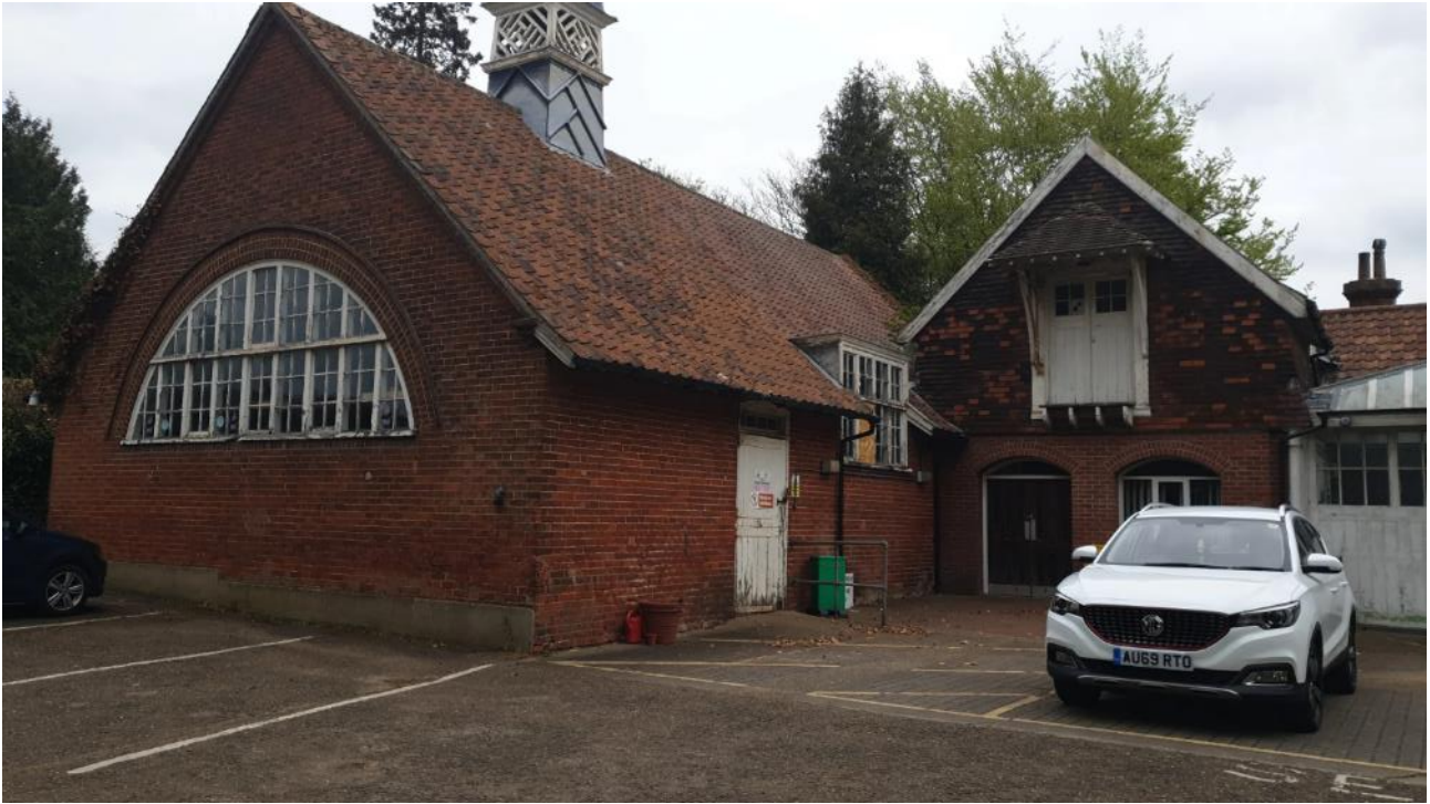
Figure B.1 The locally listed Stables (Building 1 on Figure A)
