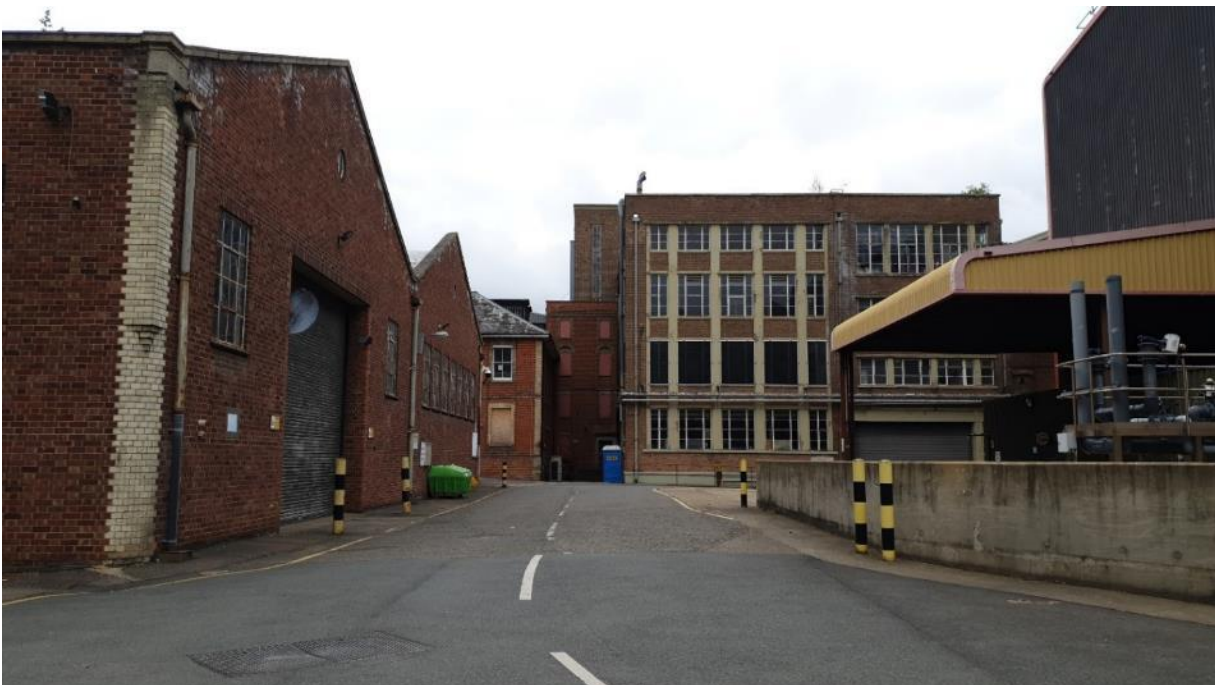
Figure 4.2 Access roads connecting the whole site
