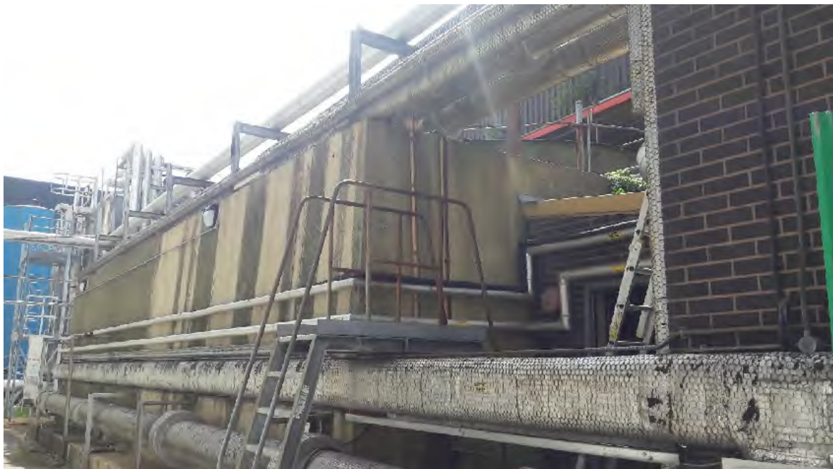
Plate 12: Bund containing water tank and dis-used diesel fuel tank (located behind the mustard seed silos)
