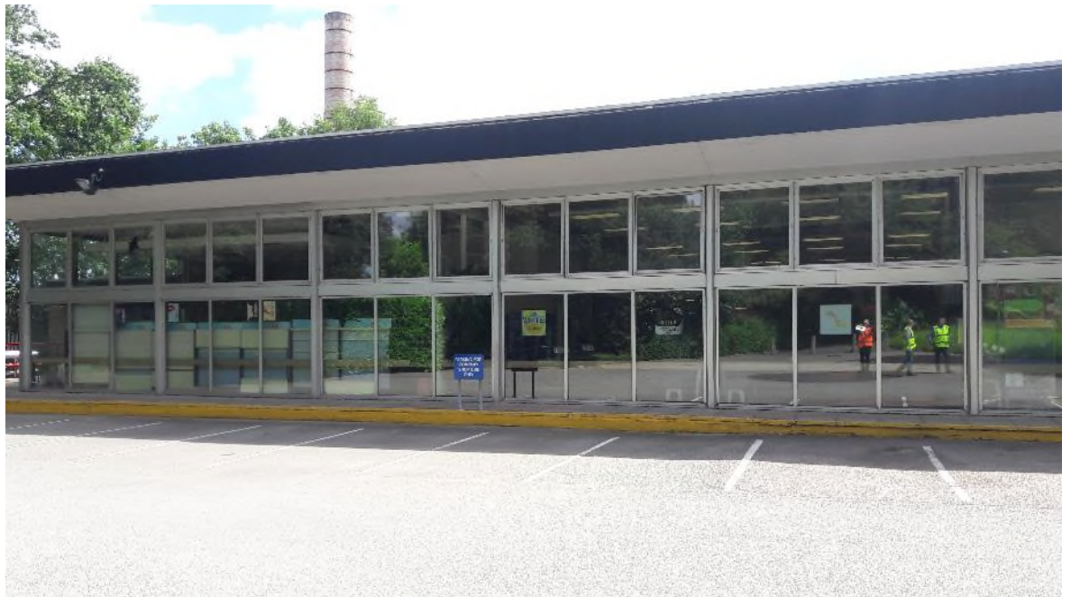
Plate 2: Canteen to the north of the conference centre
