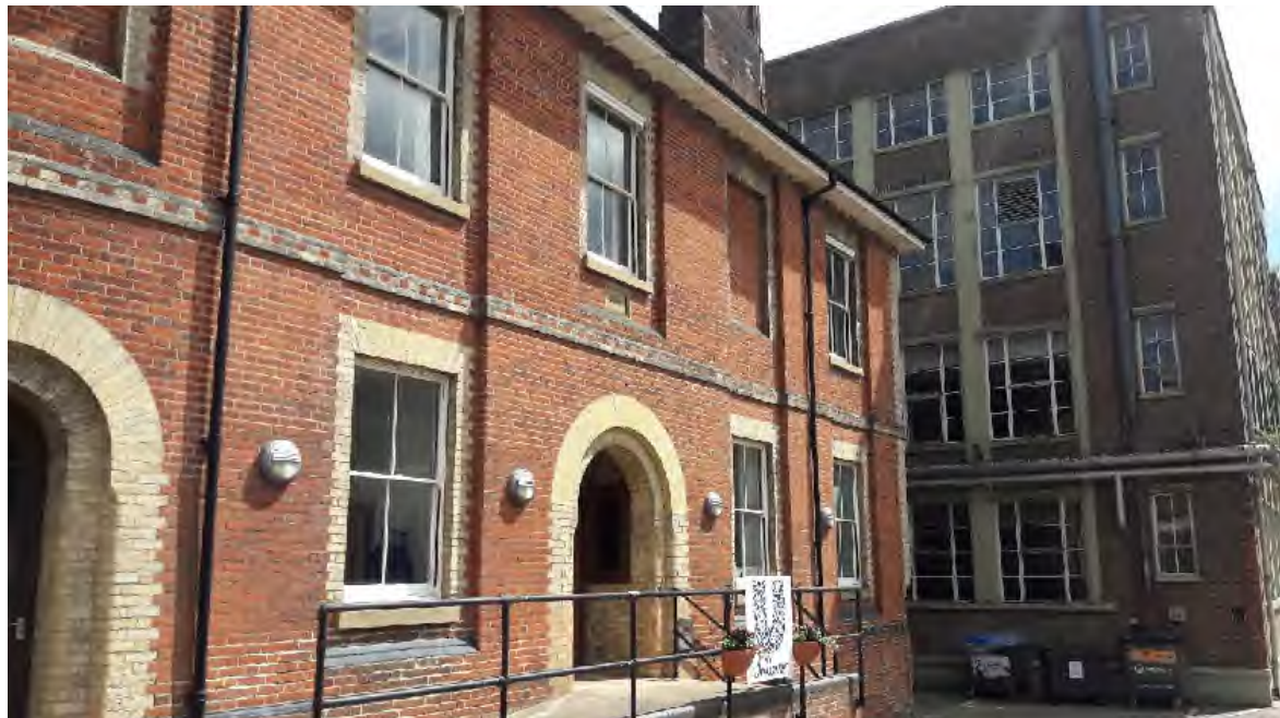
Plate 4: Older (listed) buildings in the northwest of the site. Now largely disused. Former tin production area. BH 'C' is located within
