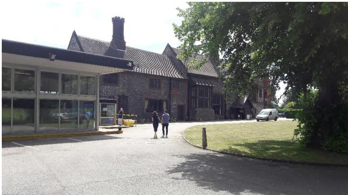
Plate 10: Canteen and conference centre looking southeast
