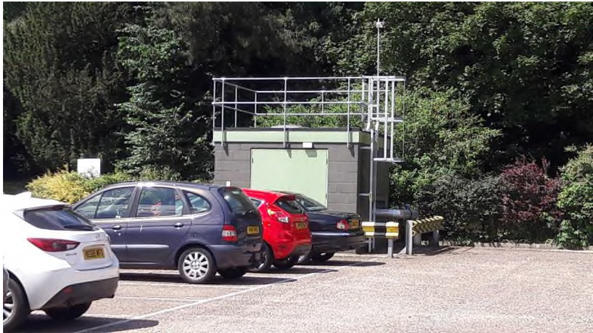
Plate 9: Borehole 'H' located within the conference centre parking facilities
