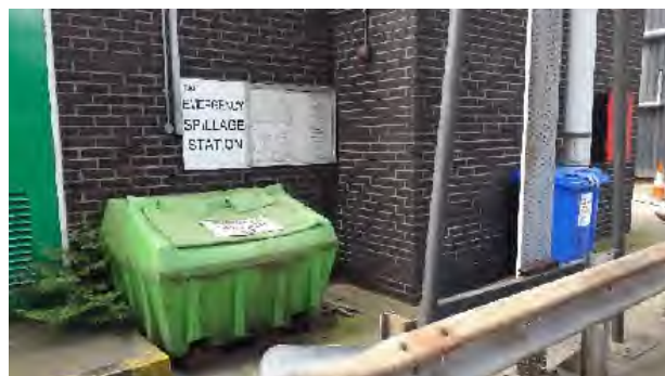
Plate 10: Gas cylinder storage and one of the emergency spillage stations (east of building 107)
