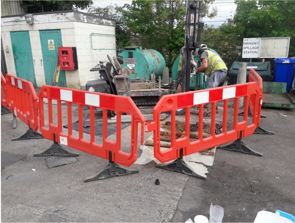
Plate 7: Heras fencing bordering off drilling work in Area 4.
