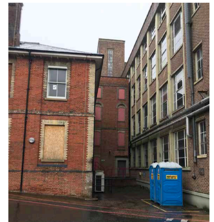
Figure 5.47 Southeastern corner of Counting House, showing connecting wing to Block 5 (Del Rosa) and Blocks 206 A-D
