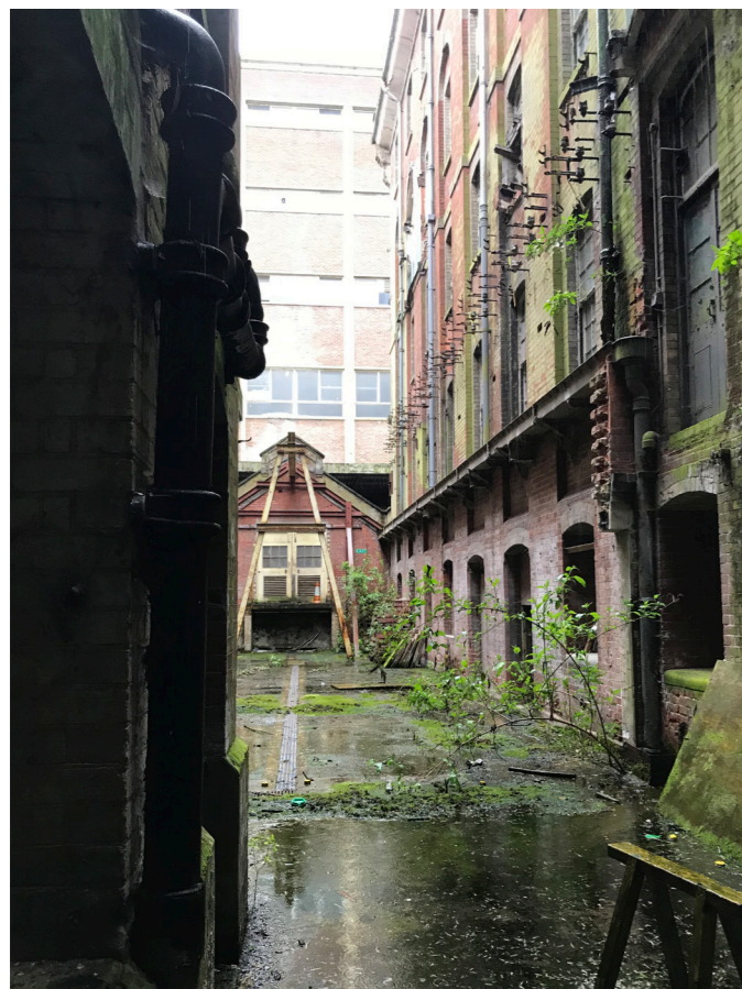
Figure 5.50 Courtyard between blocks 8 and 8A, looking east towards the site of the former electric generator
