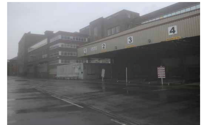
Figure 5.79 View of Jif Plant from southeast. 1994 loading bay in foreground
