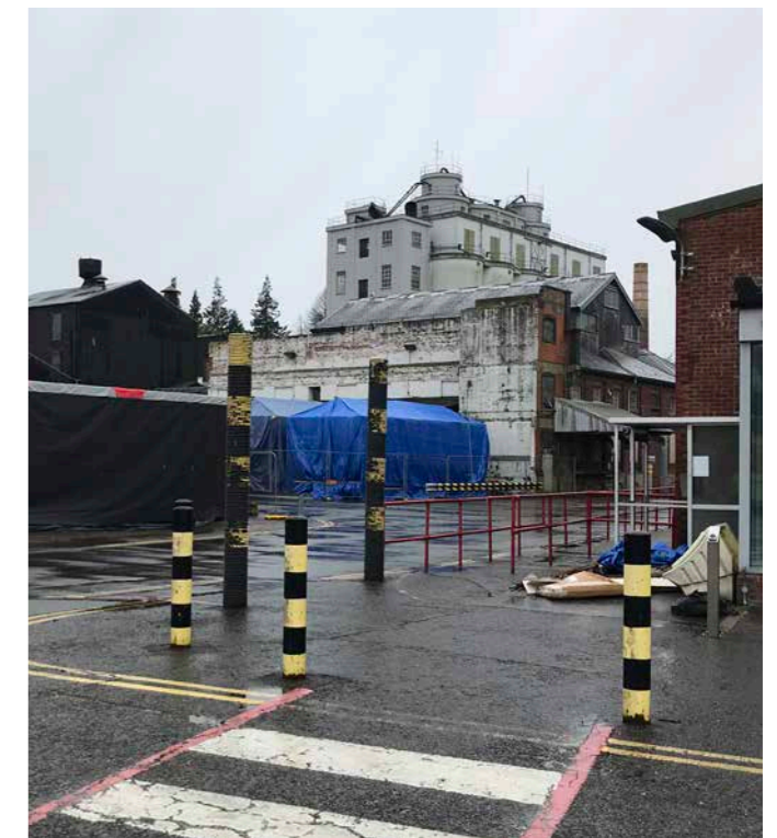
Figure 5.76 View of the Mustard Seed Silos from the northeast
