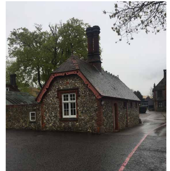
Figure 5.33 View of Gardener's Cottage from south-east
