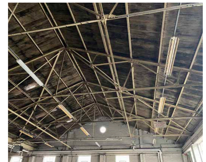
Figure 5.73 Garage interior, showing the steel roof trusses
