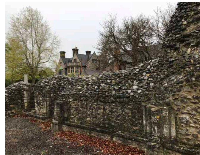
Figure 5.19 South Transept wall base in 2021
