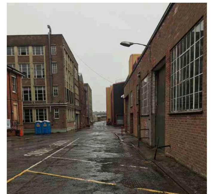
Figure 5.59 Looking east toward Block 206 (left, behind the Counting House)
