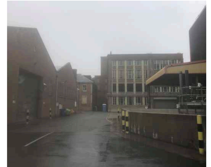
Figure 5.58 South elevation of Block 206 (right, behind metal canopy). Del Rosa' can be seen to the left
