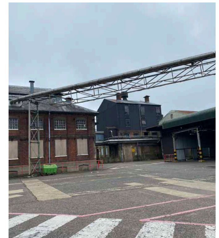
Figure 5.64 Looking towards the northwest corner attic. The Mustard Seed Driers are in the foreground (left)
