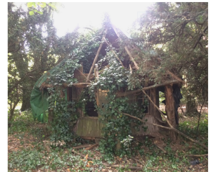
Figure 5.37 The Rustic Summerhouse from the northwest Source: CgMs 2018 Built Heritage Assessment
