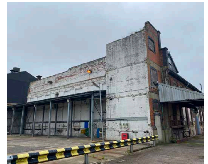
Figure 5.61 View towards east (left) and north (right) elevations
