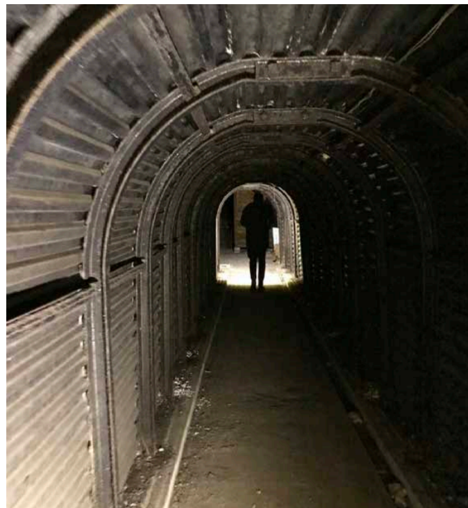
Figure 5.68 Eastern air raid shelter tunnel
