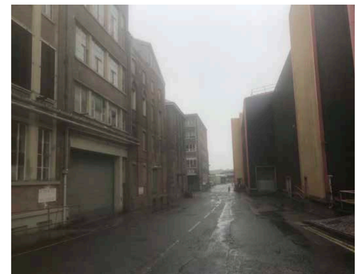
Figure 5.5 'Street' between industrial buildings to the north of the Site
