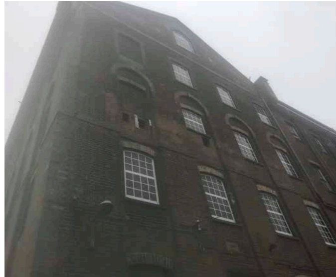
Figure 5.52 Western gable of Block 7A
