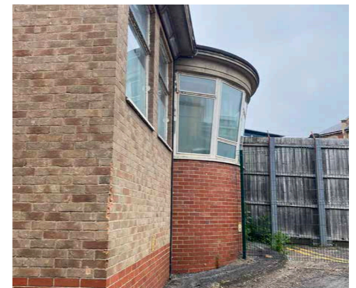
Figure 5.84 The canted corner bay at the station's eastern end
