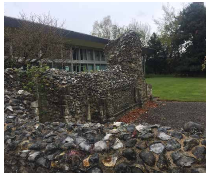
Figure 5.17 View of South Transept, looking north
