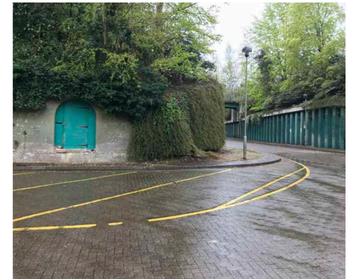
Figure 5.67 Entrance to eastern air raid shelter
