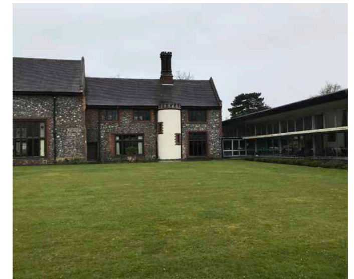
Figure 5.23 East Elevation of Carrow Abbey in May 2021
