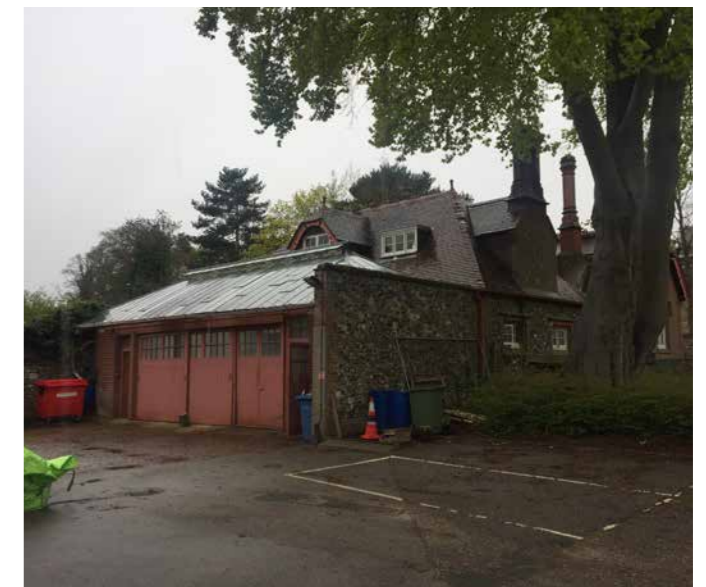
Figure 5.34 Lodge and Garage photographed from the north-west
