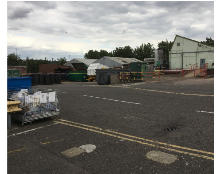
Figure 5.89 View of the Mint Plant from the southwest Source: CgMs 2018 Heritage Assessment
