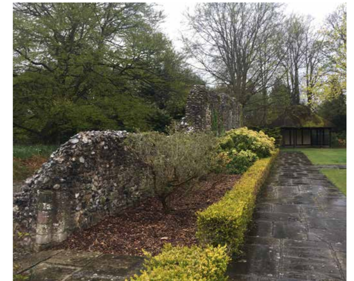
Figure 5.12 Remnants of Cloister walls, looking south
