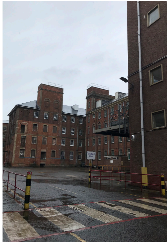
Figure 5.51 View of Blocks 7 and 8A from the east
