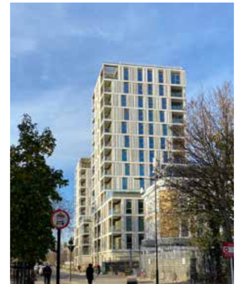
Acceptable approach to design of the tallest gateway building into Carrow Works. Simple and rhythmic forms drawing inspiration from the Silos.
