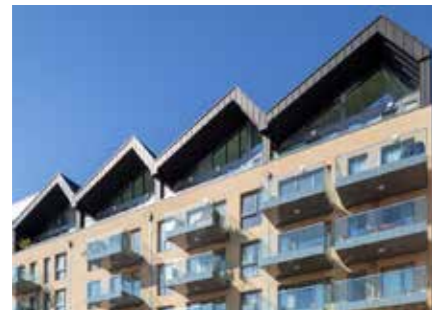
Example of saw tooth roof forms and the use of corrugated panels as primary material to reflect the existing Culinary Unit on the site.
