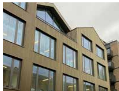
Acceptable contemporary translation of warehouse buildings through the use of coloured corrugated panels as primary material, with simple, large, inset windows. The variance in roof line also helps to create relief along the street scene.
