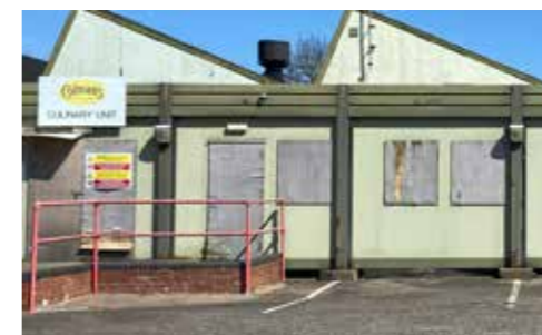
Rhythmic, saw tooth roofs and dark apple green panels to frame the building.
