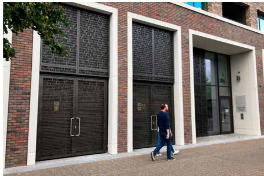
Discreetly located entrance to car park and textured, timber façade to sub-station
