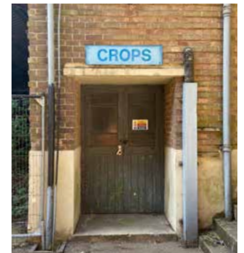
Signage on buildings and inset entrances
