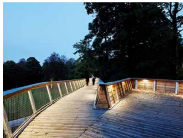
Example of how lighting can make features out of ramped access to promote a feeling of safety. (Image: Atelier Espace Libre)
