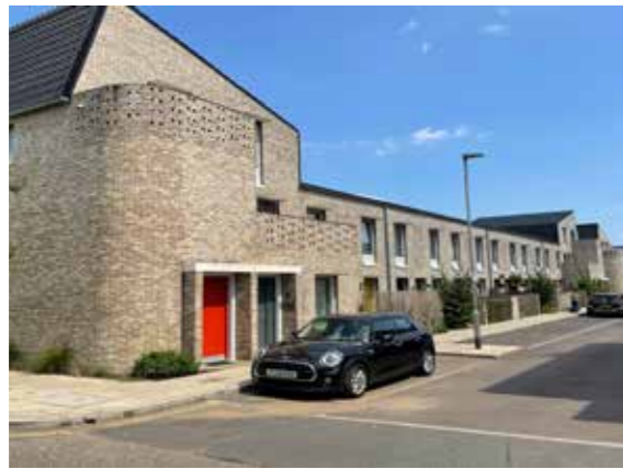
Example of side-on housetypes, sensitively addressing The Abbey and Cottages Character Area. This example at Goldsmith Street in Norwich illustrates an acceptable approach to mews street with discreet on-street parking and varied house typologies that encourage multi-generational living. The diverse mix of homes introduce further interest in the street and roofscape.
