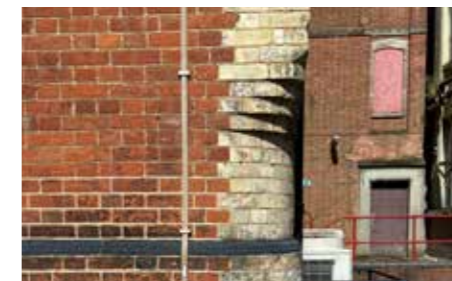
Brick quoining with rounded corner and stepped corbel above
