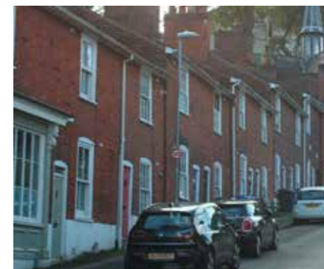
Terraced housing with a consistent frontage
