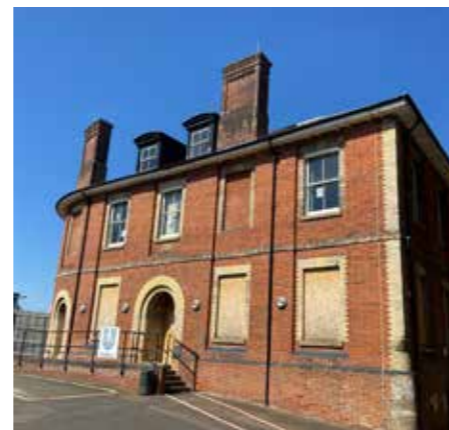
Grade II Listed Offices
