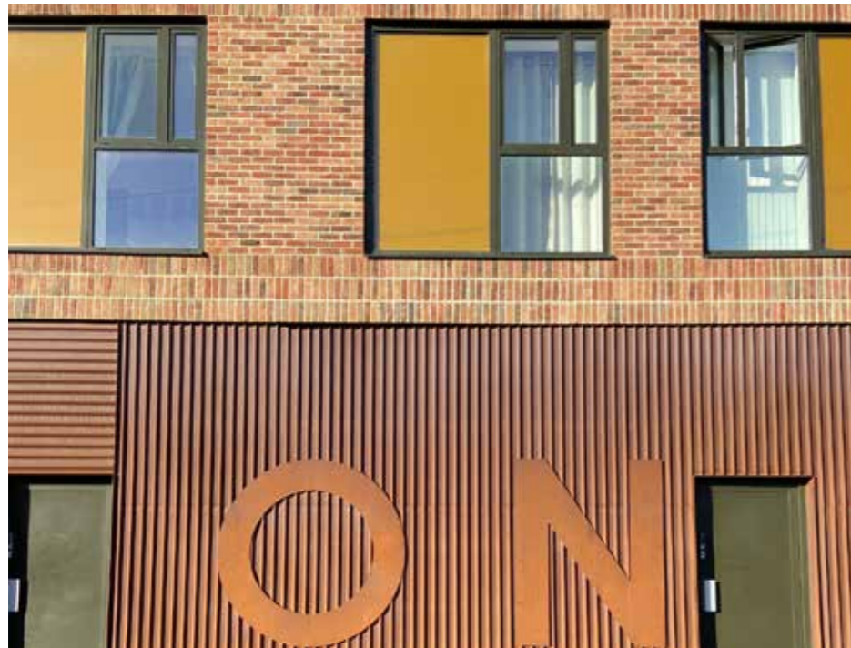
Example of acceptable use of feature colour on window reveals, corrugated panels, industrial inspired signage and brick detailing
