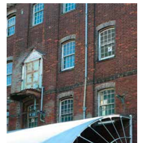
Large, uniform openings with brick arch window detailing and canopies
