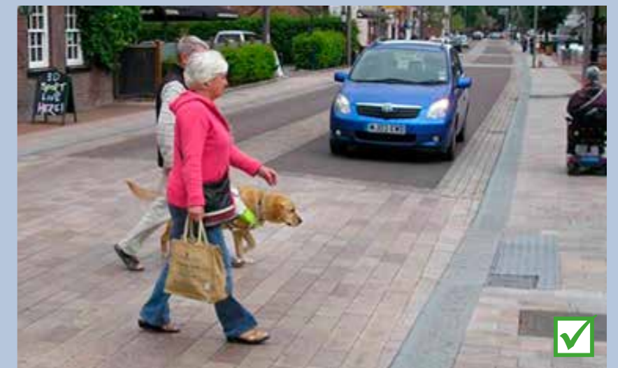
Raised shared surface crossings act as speed restraints to traffic while making it easier for wheelchair and frame users, as well as people with pushchairs, to cross the road.
