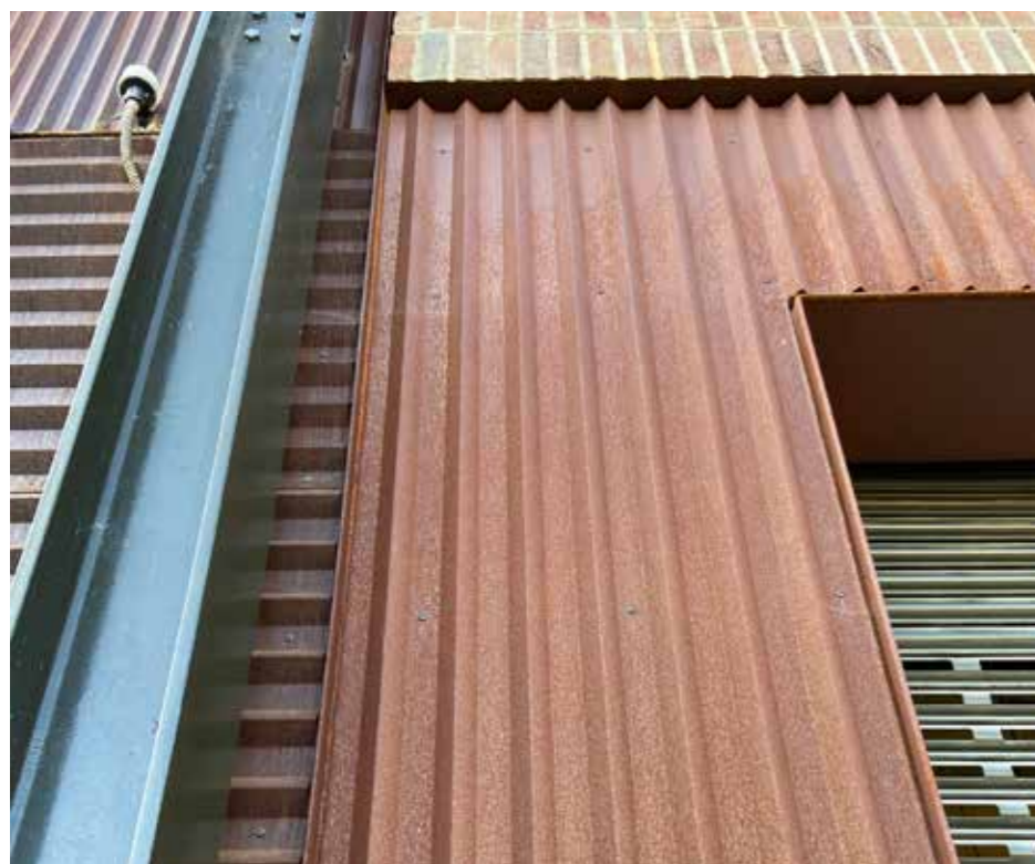
Example of corrugated panels and feature brickwork
