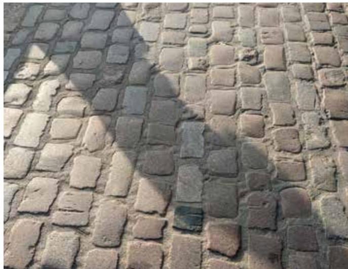
Example of reclaimed granite blocks hard surfacing
