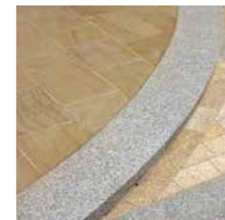
Yorkstone and granite paving.
