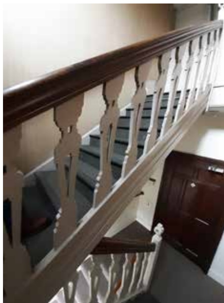
3.59 First Floor Stair F.25
