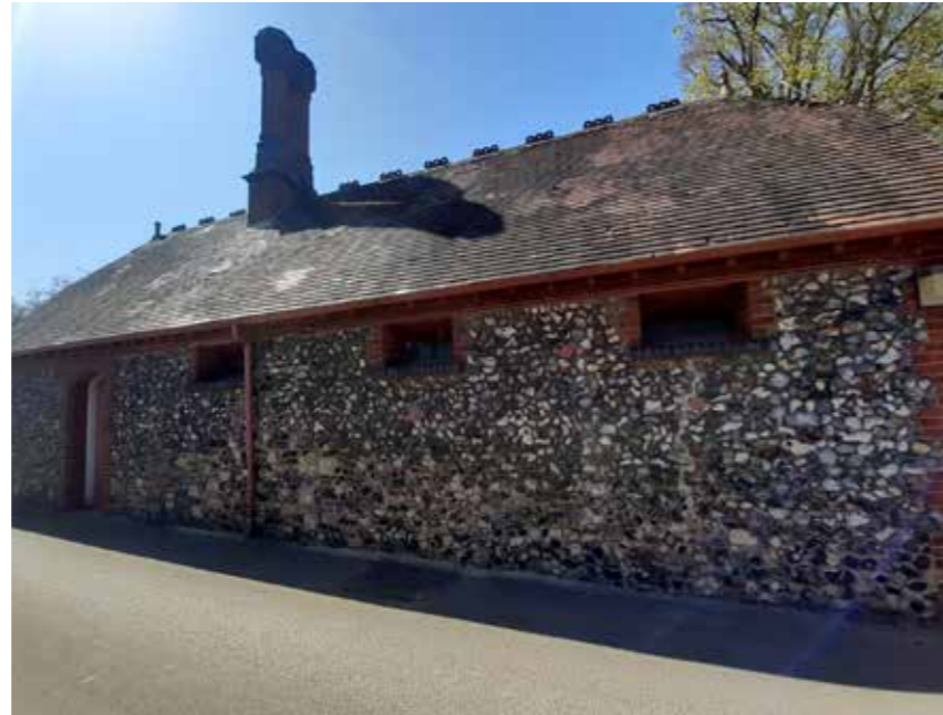
4.11 East elevation former cart shed
