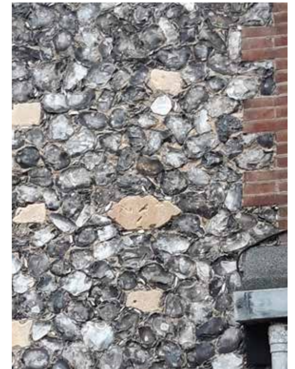
3.18 Wall finish flint and brick 3
