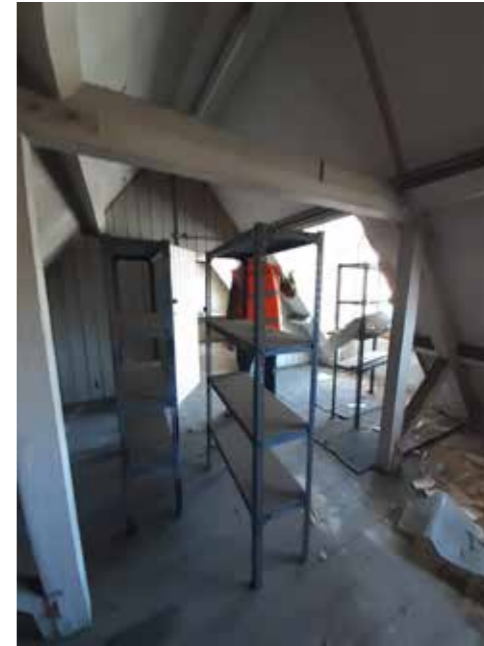
4.33 Gardener's cottage first floor north F.10
