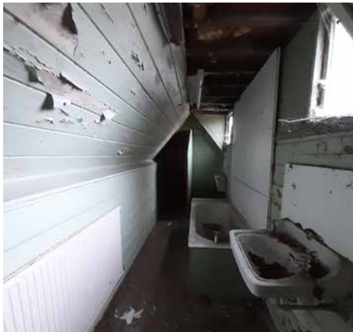
4.25 Lodge first floor F.06
