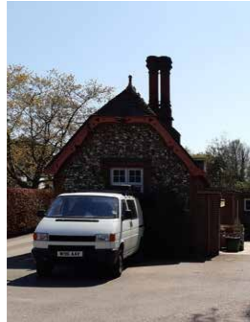
4.12 North elevation former cart shed
