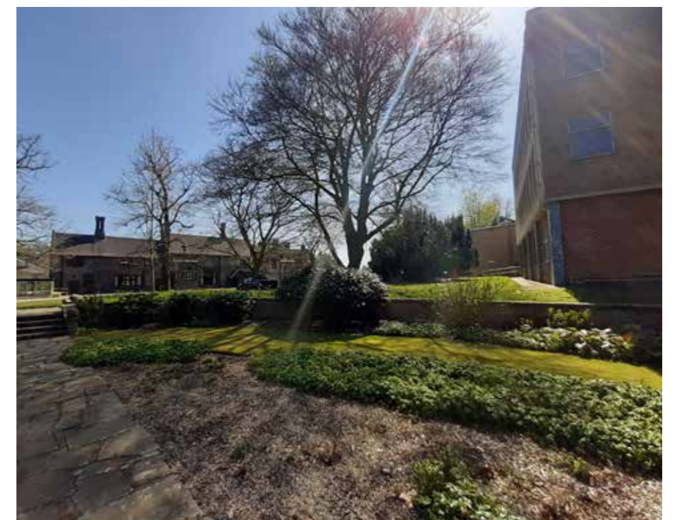
3.3 (West elevation) View of Abbey from the sunken garden (Grade II)
