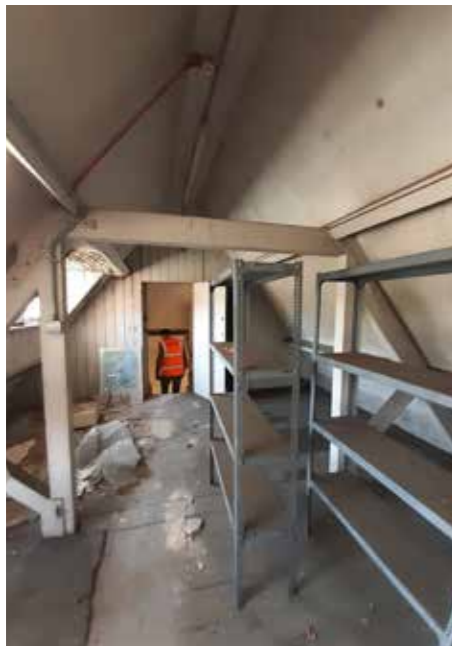
4.34 Gardener's cottage first floor looking south F.10
