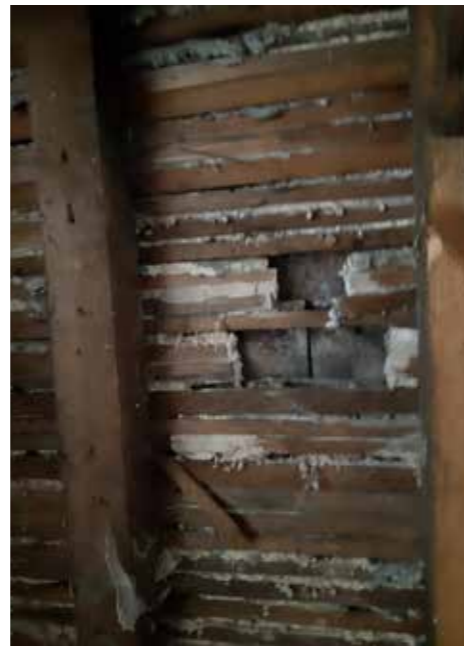
4.26 Lodge first floor F.04 roof (showing underside of tiles)
