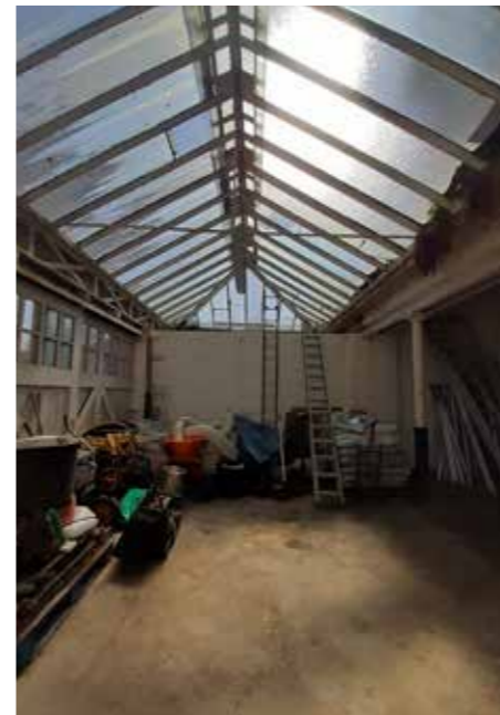
4.27 Gardener's cottage ground floor looking south G.14
