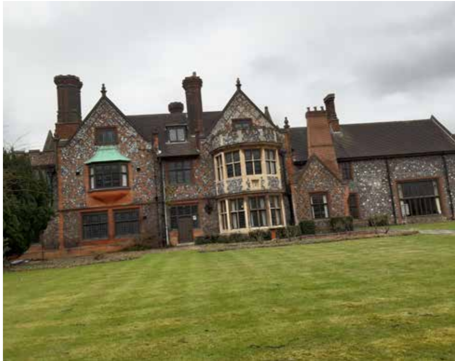
3.13 East elevation of C19 southern range with gable fronts
