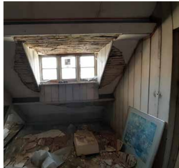
4.36 Gardener's cottage first floor south dormer F.10
