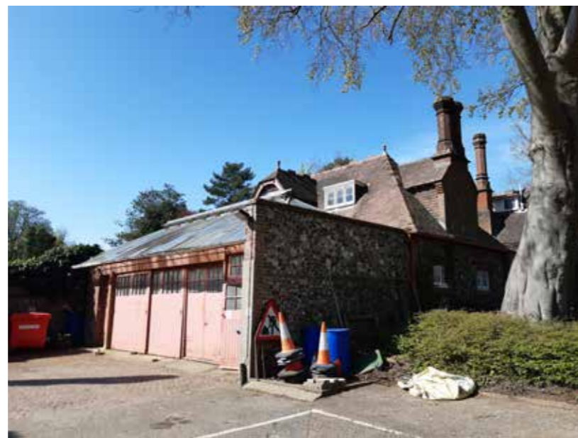
8.3 Level access to gardeners cottage to be maintained
