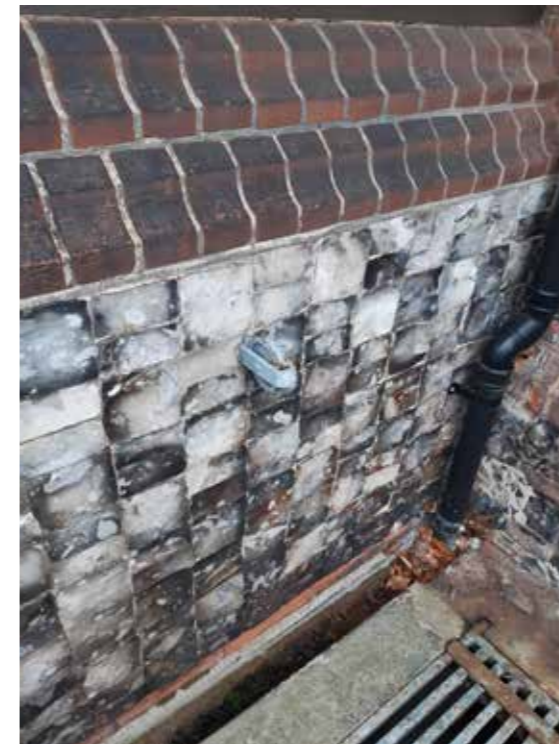
3.17 Wall finish flint and brick 2
