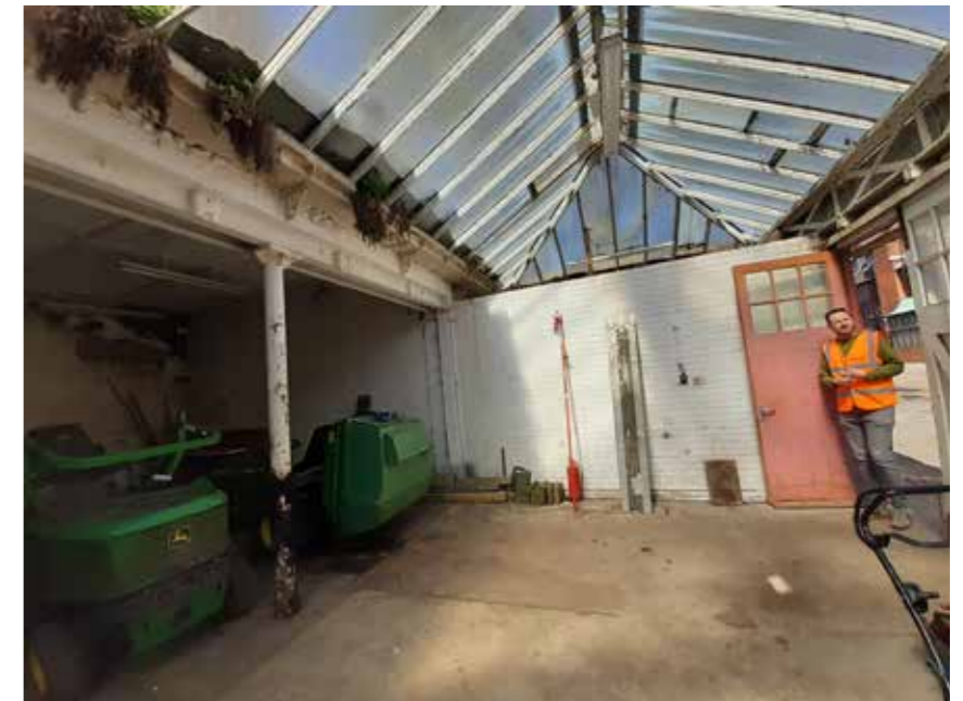
4.28 Gardener's cottage ground floor looking north G.14 and G.13
