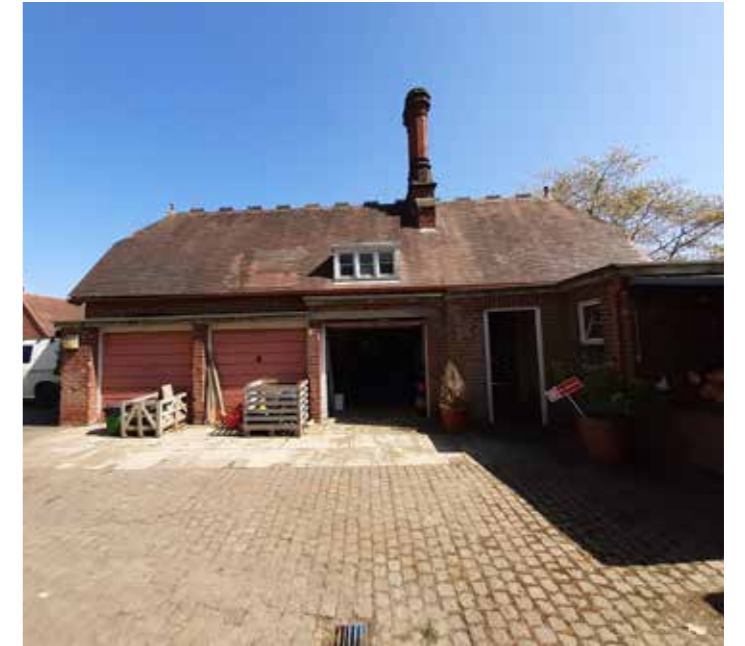
4.13 West elevation former cart shed
