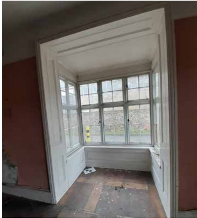
4.21 Lodge ground floor G.01 bay window
