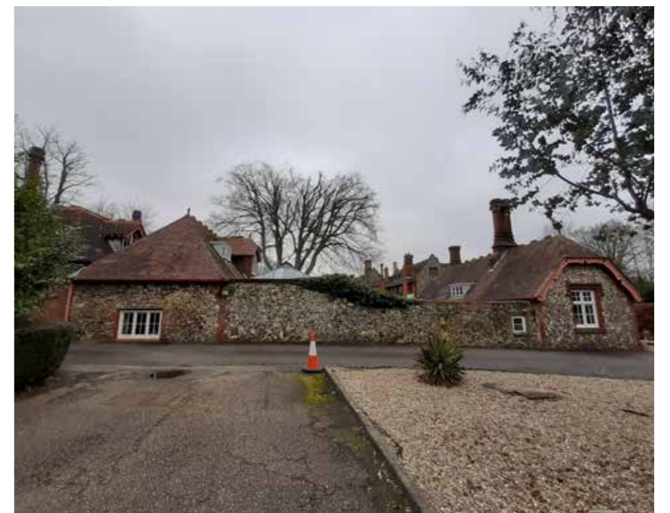
4.4 South elevation of gardener's cottage and former cart shed
