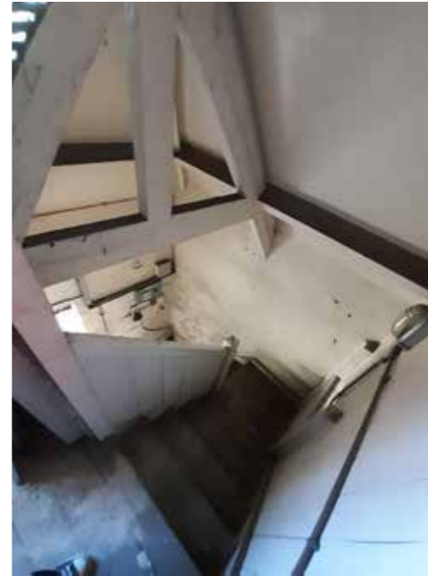
4.31 Gardener's cottage first floor stair
