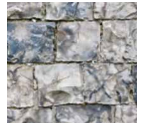
6.15 Knapped flint squared and coursed
