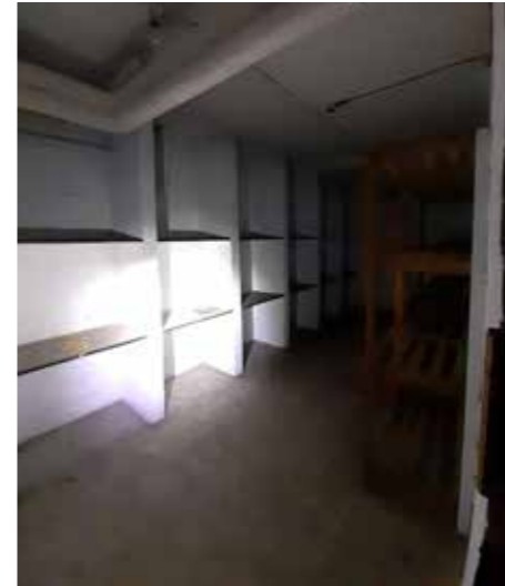
3.20 Basement Room B.09
