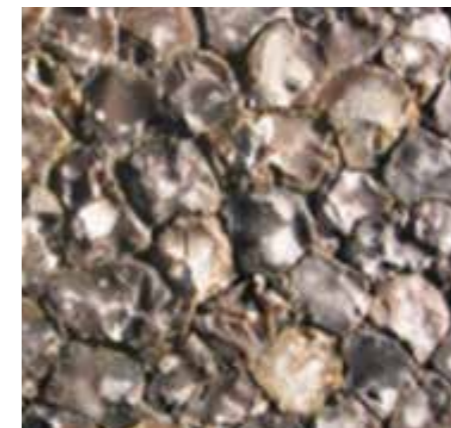
6.14 Cobbled finish of even colour, laid randomly with coursed flint
