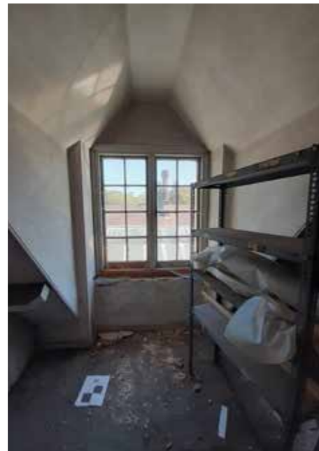
4.35 Gardener's cottage first floor middle dormer F.10
