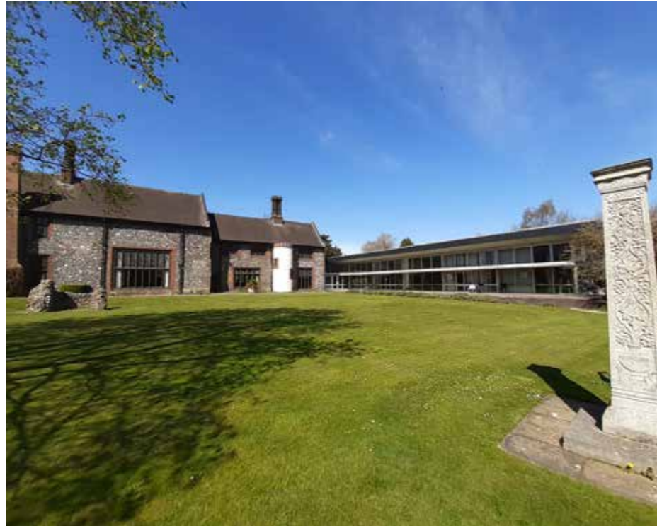
3.5 Dining Hall to north of Abbey (east elevation)
