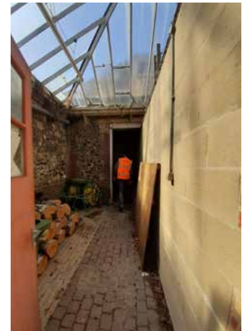
4.29 Gardener's cottage ground floor partitioned area to south G.15
