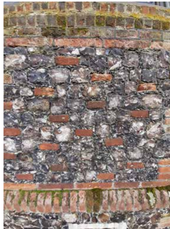
3.16 Wall finish flint and brick 1
