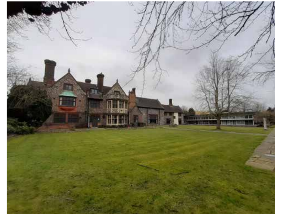
3.12 East elevation of Abbey with Dining Hall in background
