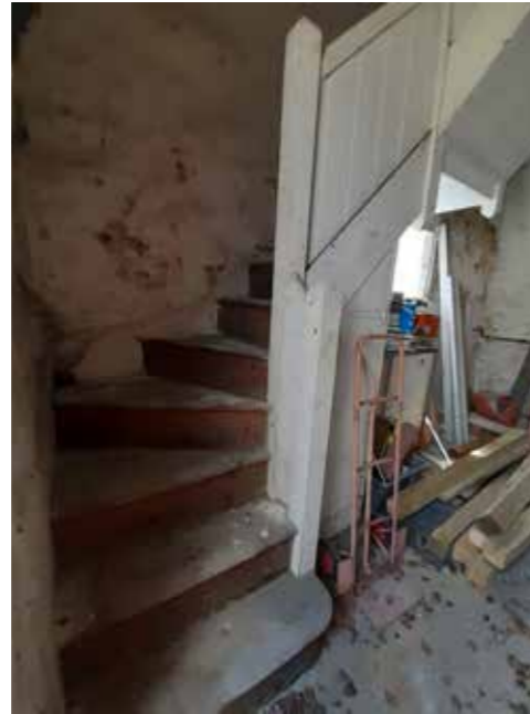
4.30 Gardener's cottage ground floor stair G.16
