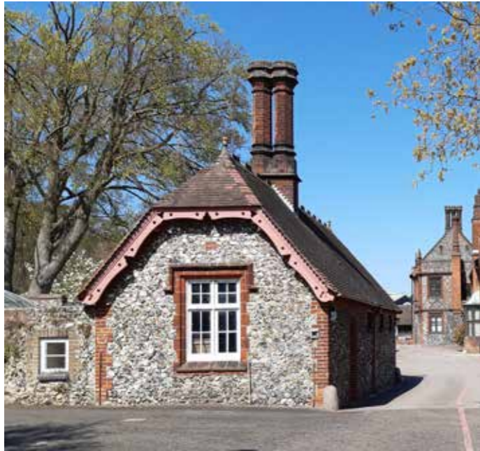
4.10 South elevation former cart shed
