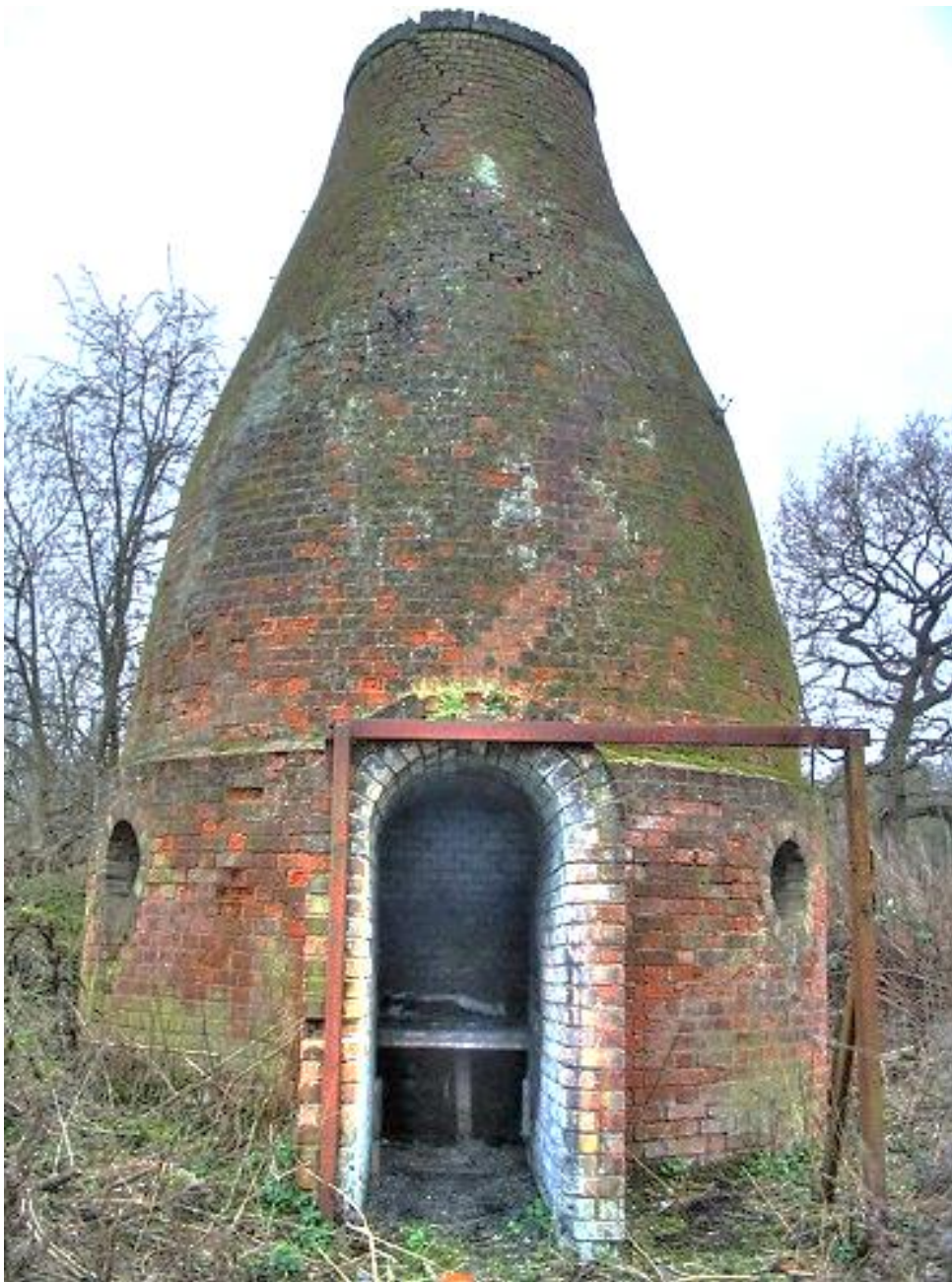
Fig. 19: Timber drying bottle kiln, Deal Ground.
