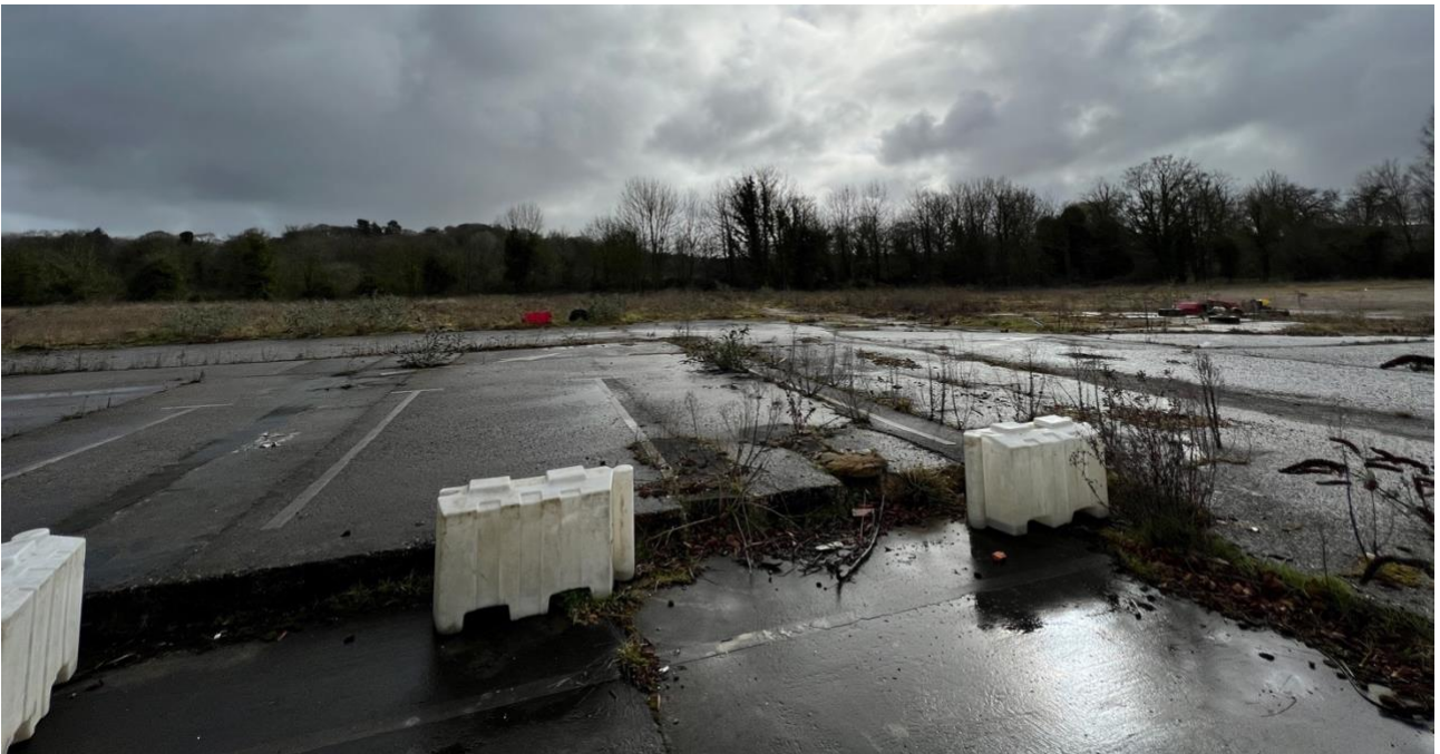
Fig. 25: View east from within the Site.
