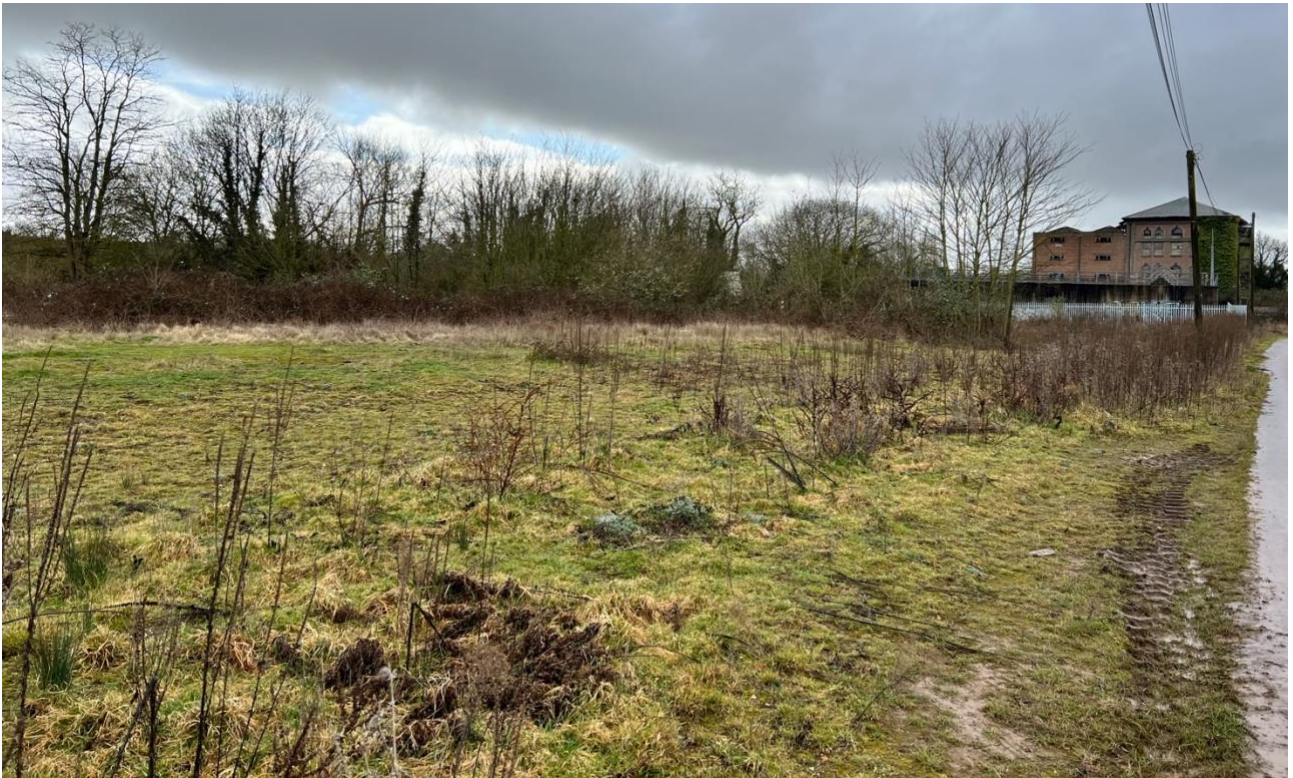
Fig. 32: View south from within the Site on the western side looking towards the grade II listed, derelict, 18 th century pumping station.
