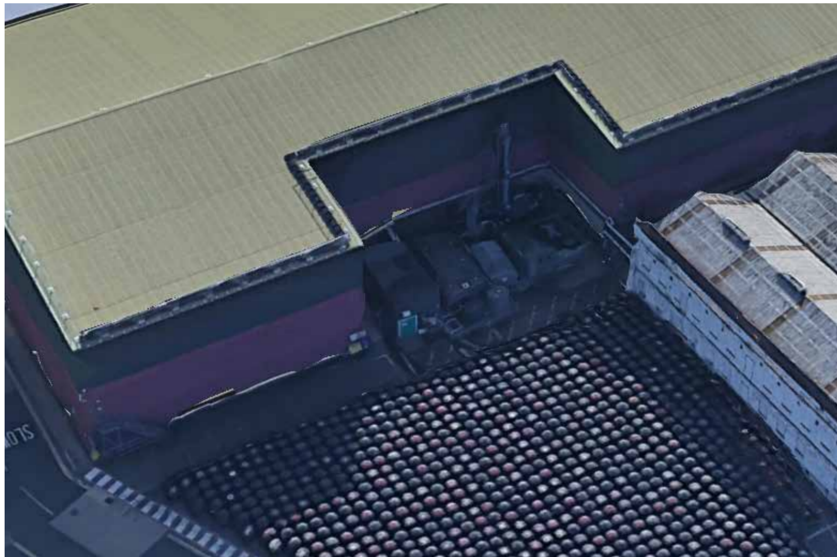
Existing Building To Be Demolished Aerial
