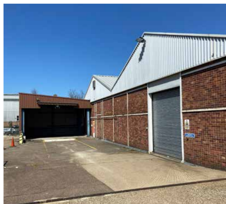
Existing Building To Be Demolished Photograph
