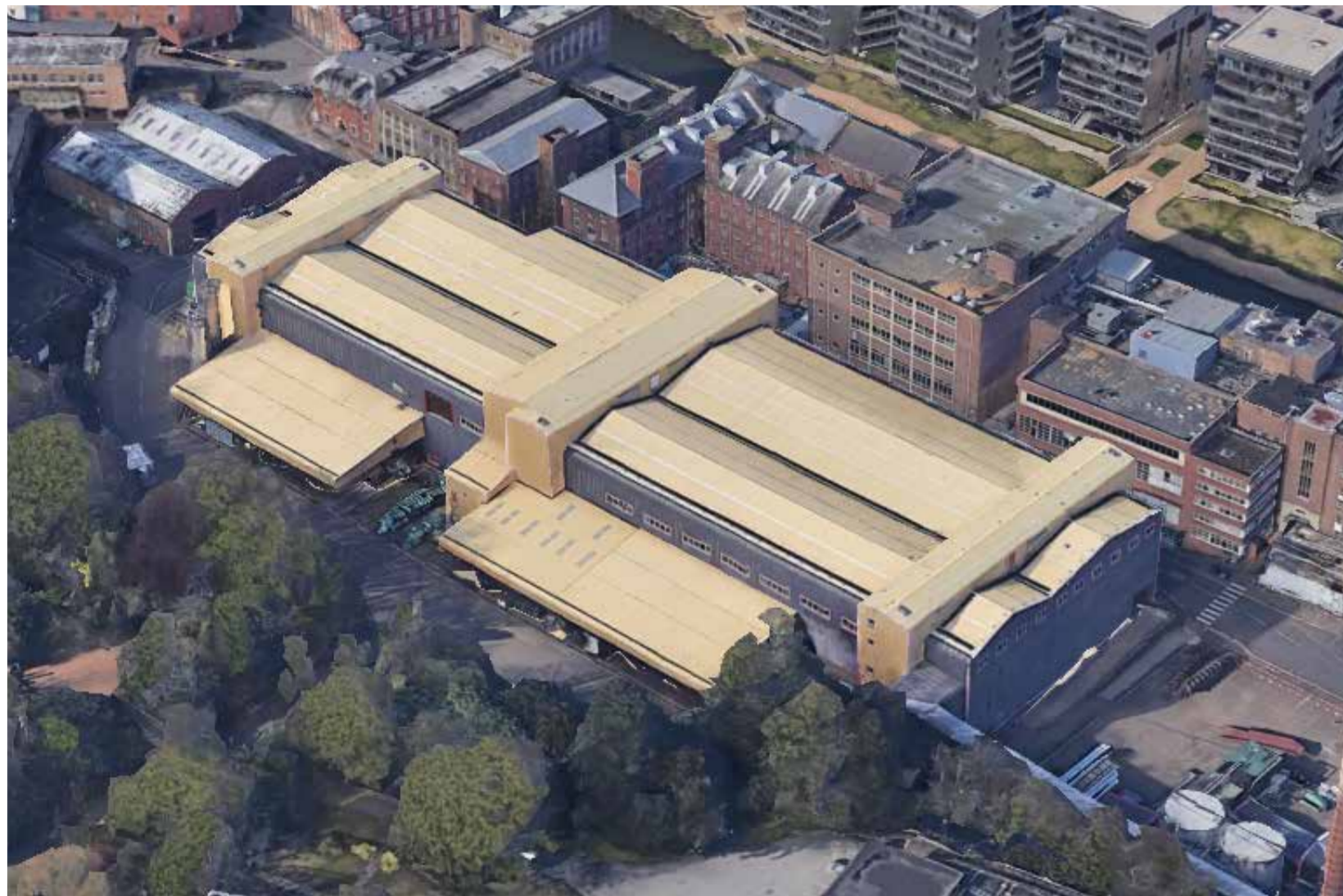
Existing Building To Be Demolished Aerial
