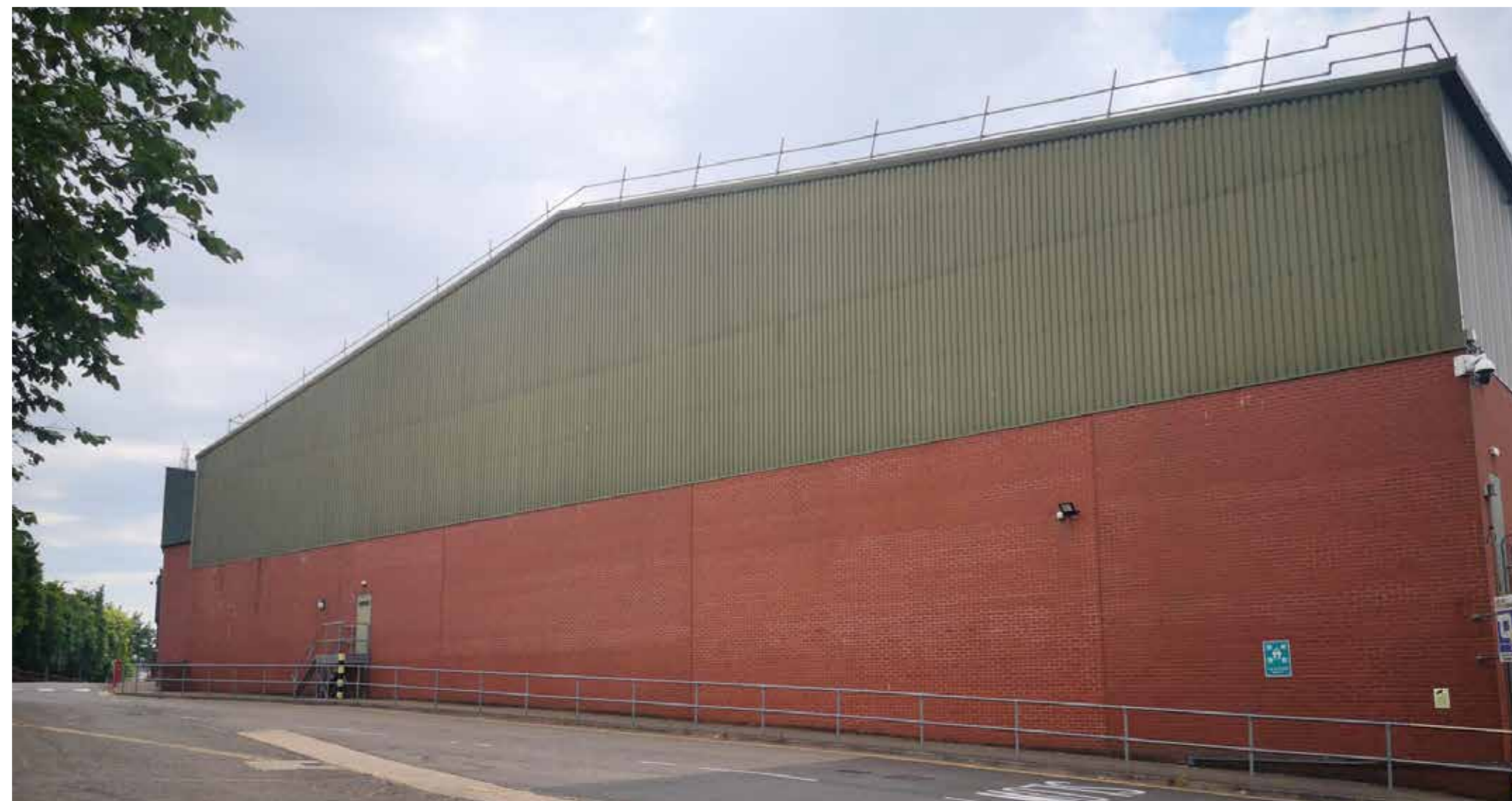
Existing Building To Be Demolished Photograph
