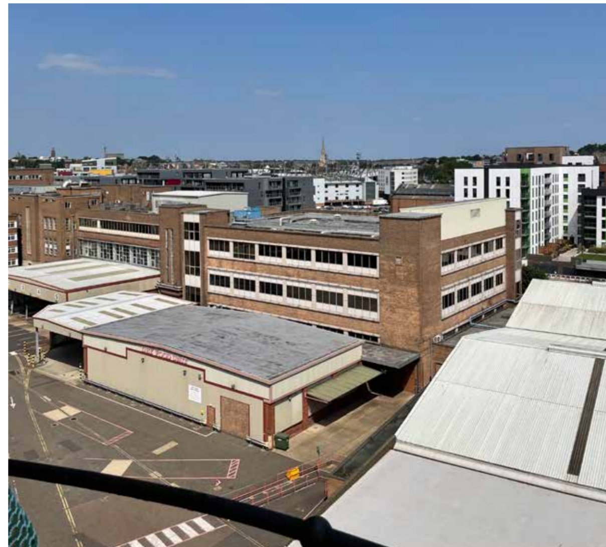
Existing Building To Be Demolished Photograph
