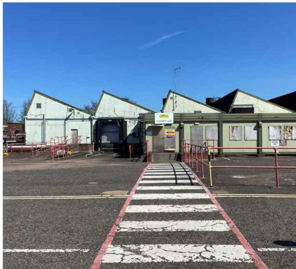
Existing Building To Be Demolished Photograph
