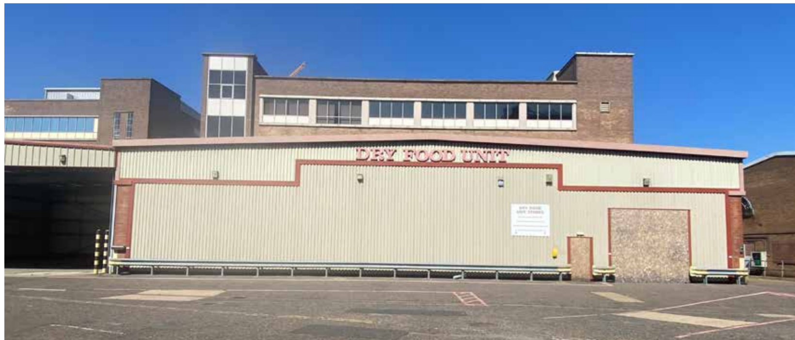
Existing Building To Be Demolished Photograph
