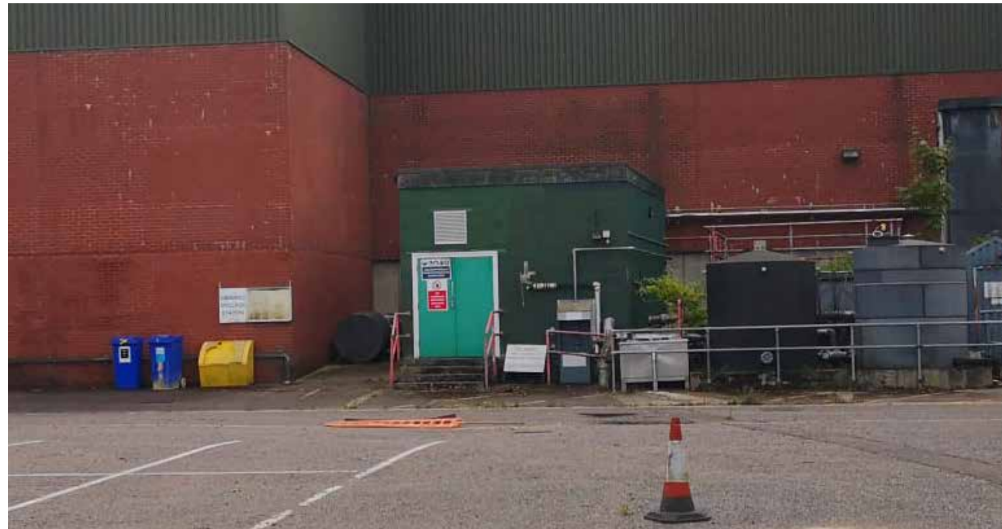
Existing Building To Be Demolished Photograph
