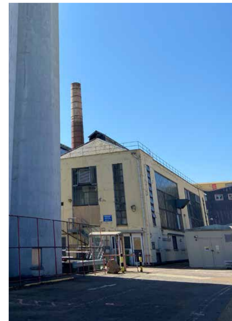
Existing Building To Be Demolished Photograph
