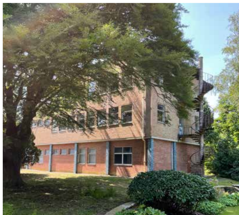
Existing Building To Be Demolished Photograph
