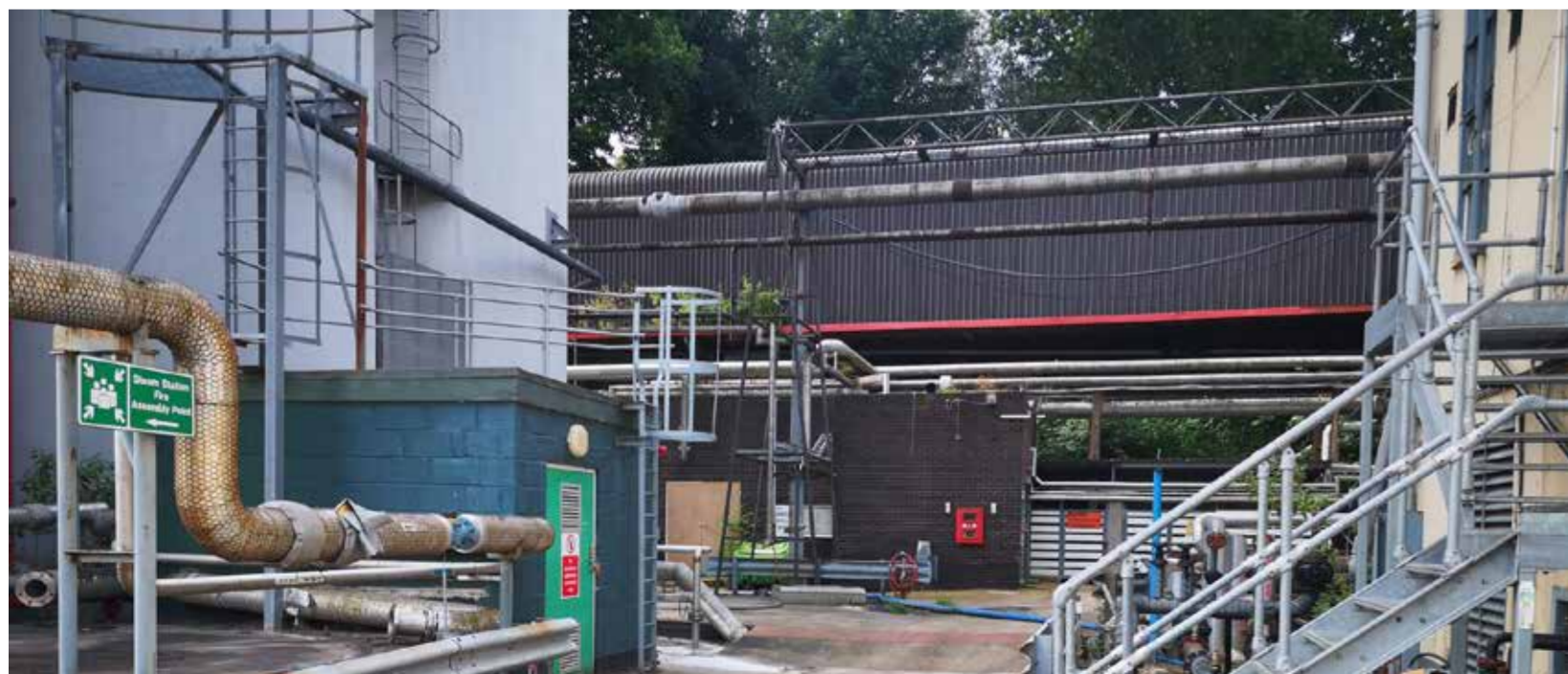
Existing Building To Be Demolished Photograph
