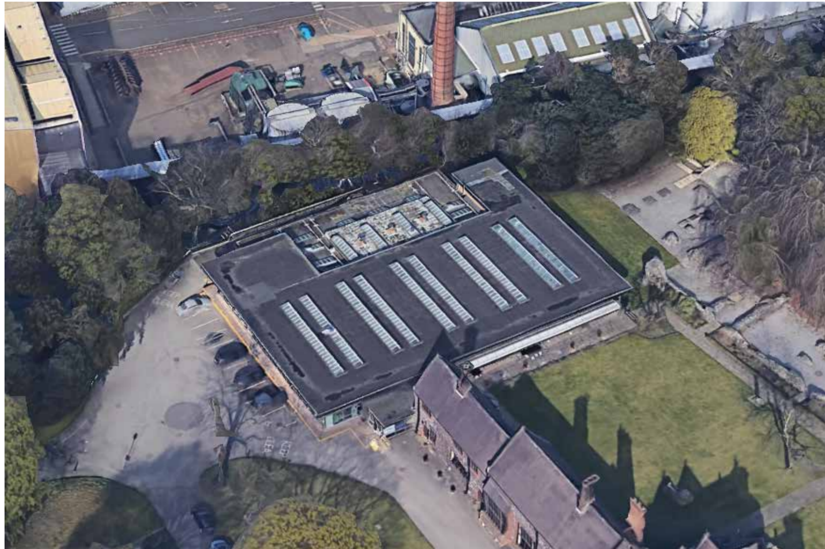
Existing Building To Be Demolished Aerial
