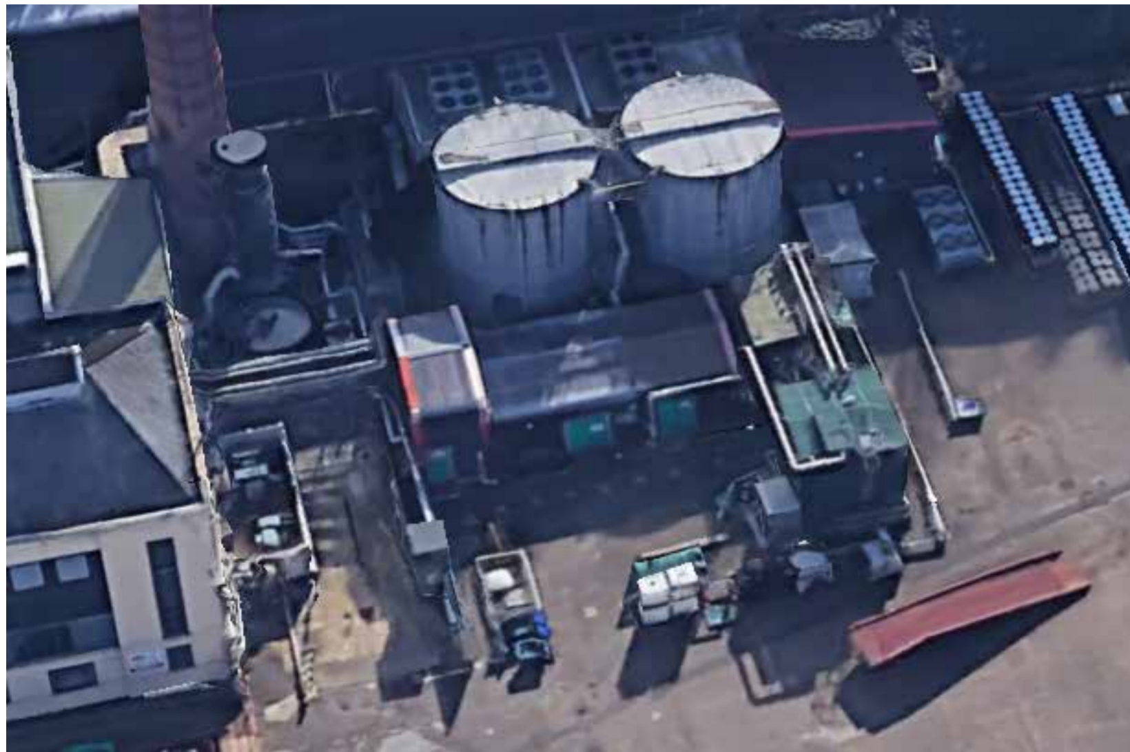
Existing Building To Be Demolished Aerial
