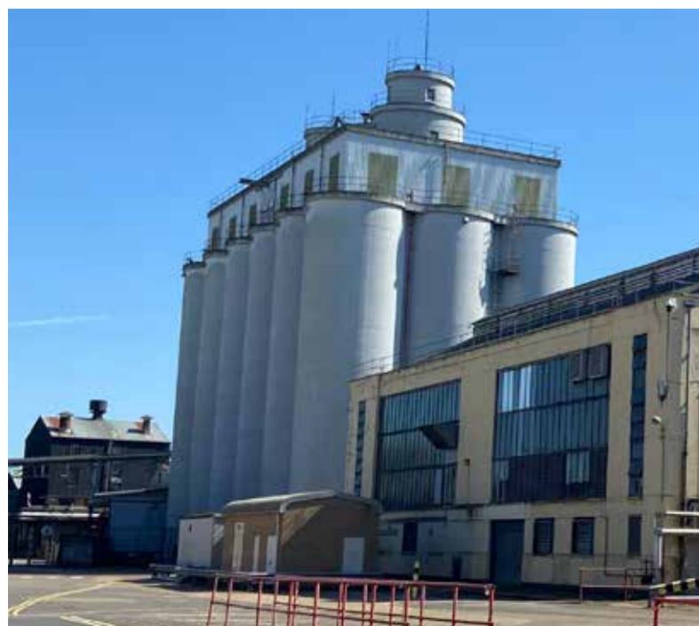
Existing Building To Be Demolished Photograph
