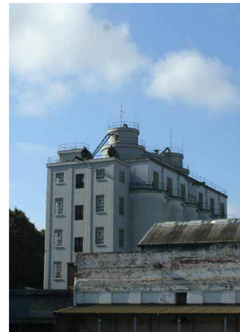
Existing Building To Be Demolished Photograph
