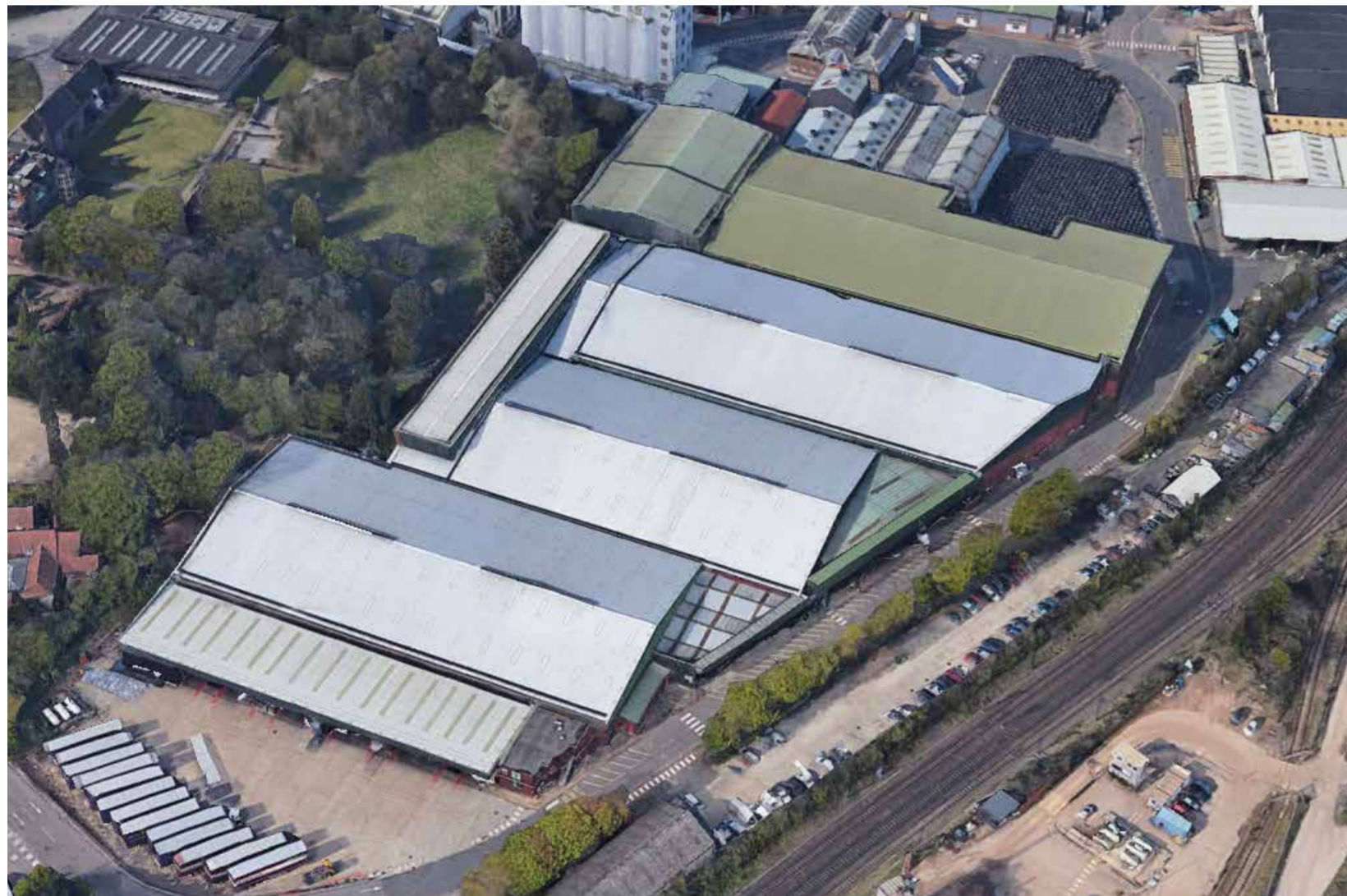
Existing Building To Be Demolished Aerial
