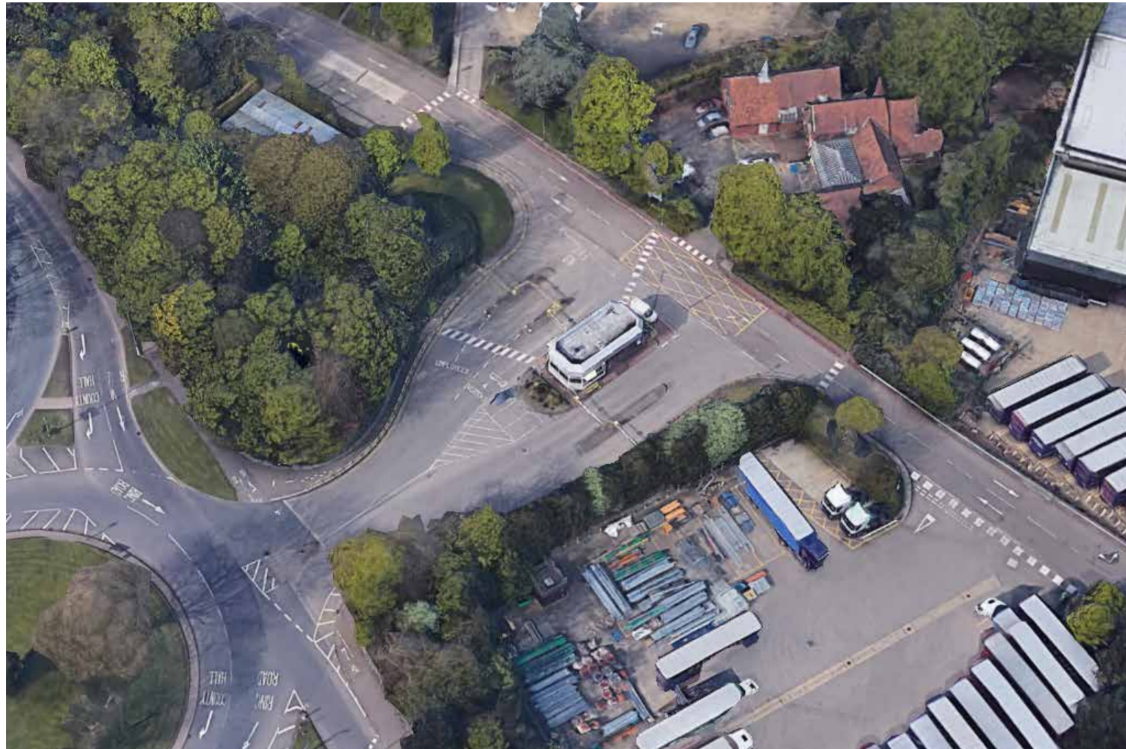
Existing Building To Be Demolished Aerial
