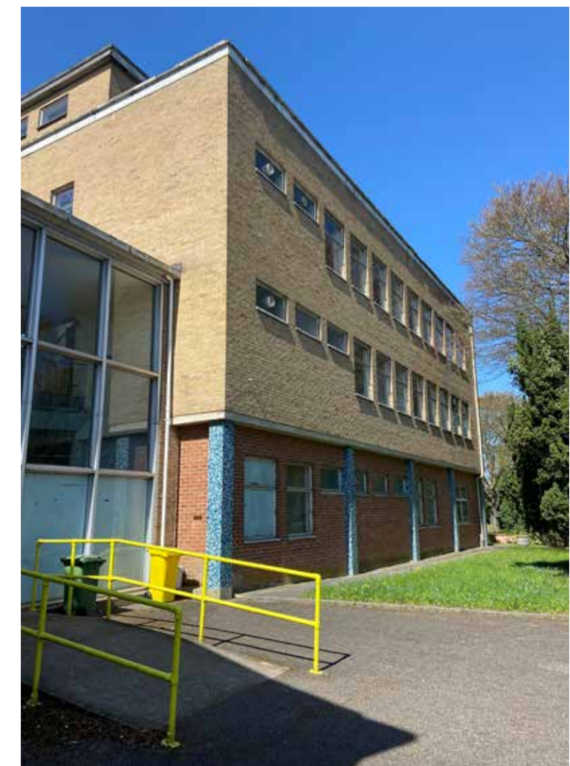
Existing Building To Be Demolished Photograph
