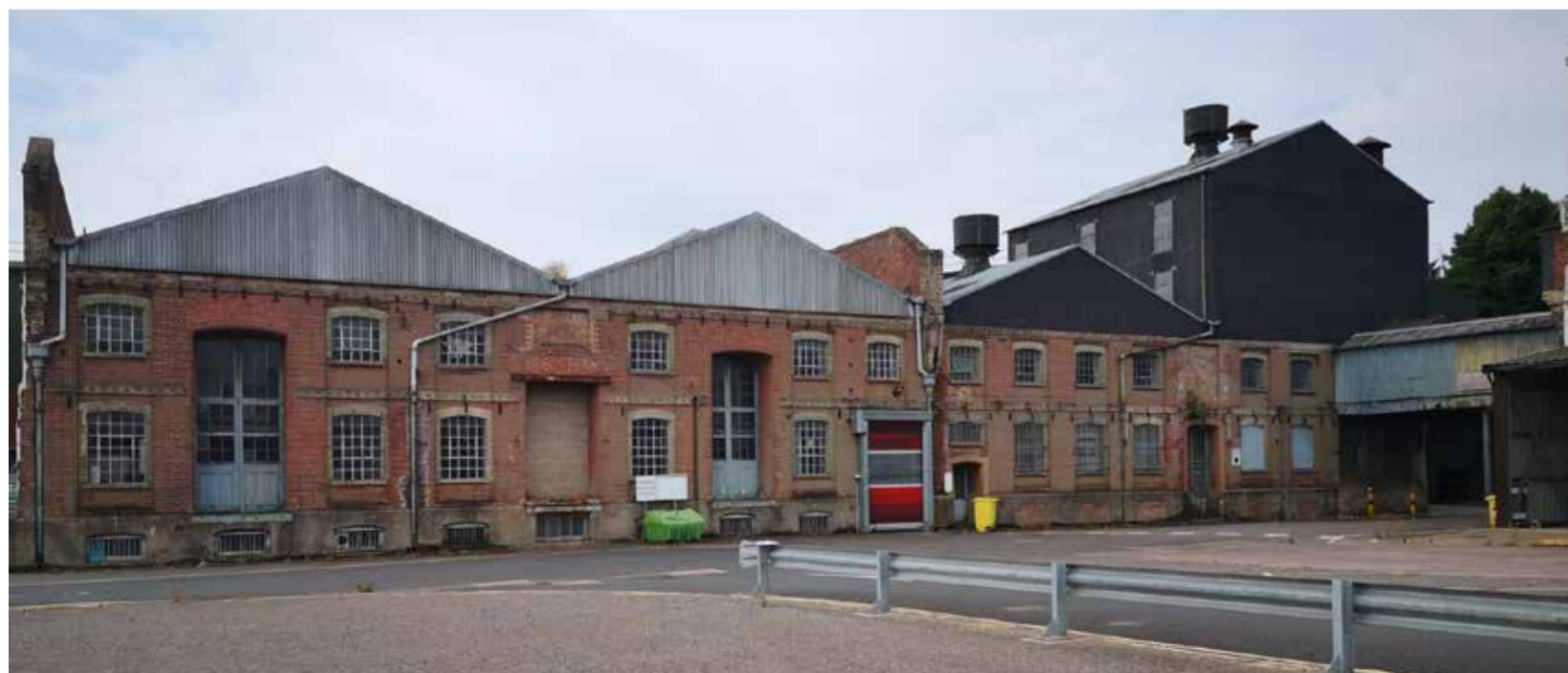
Existing Building To Be Demolished Photograph
