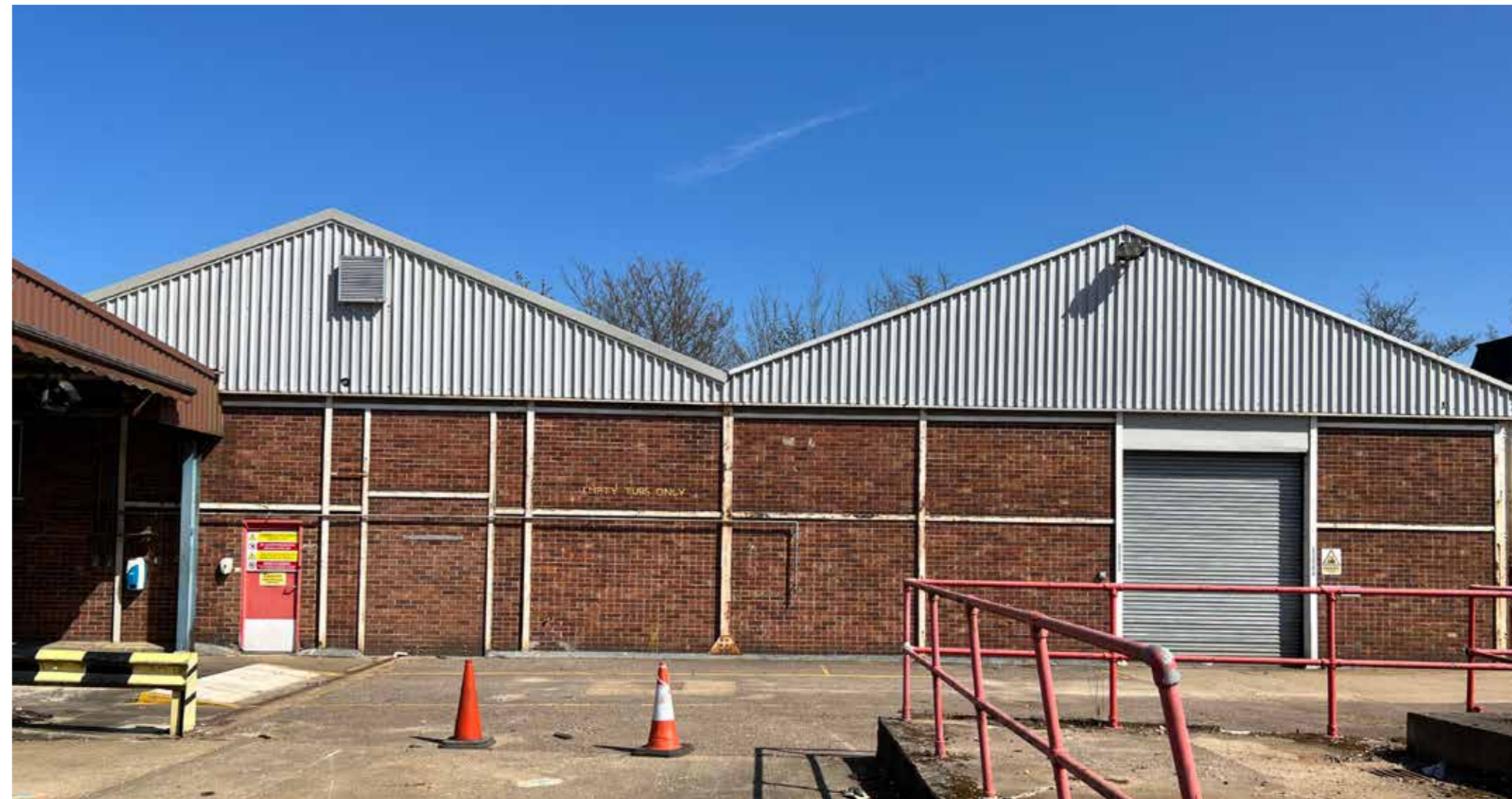
Existing Building To Be Demolished Photograph
