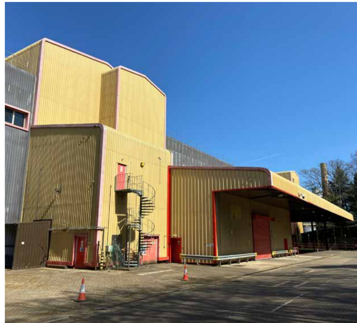
Existing Building To Be Demolished Photograph
