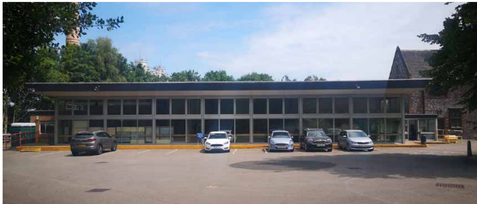
Existing Building To Be Demolished Photograph
