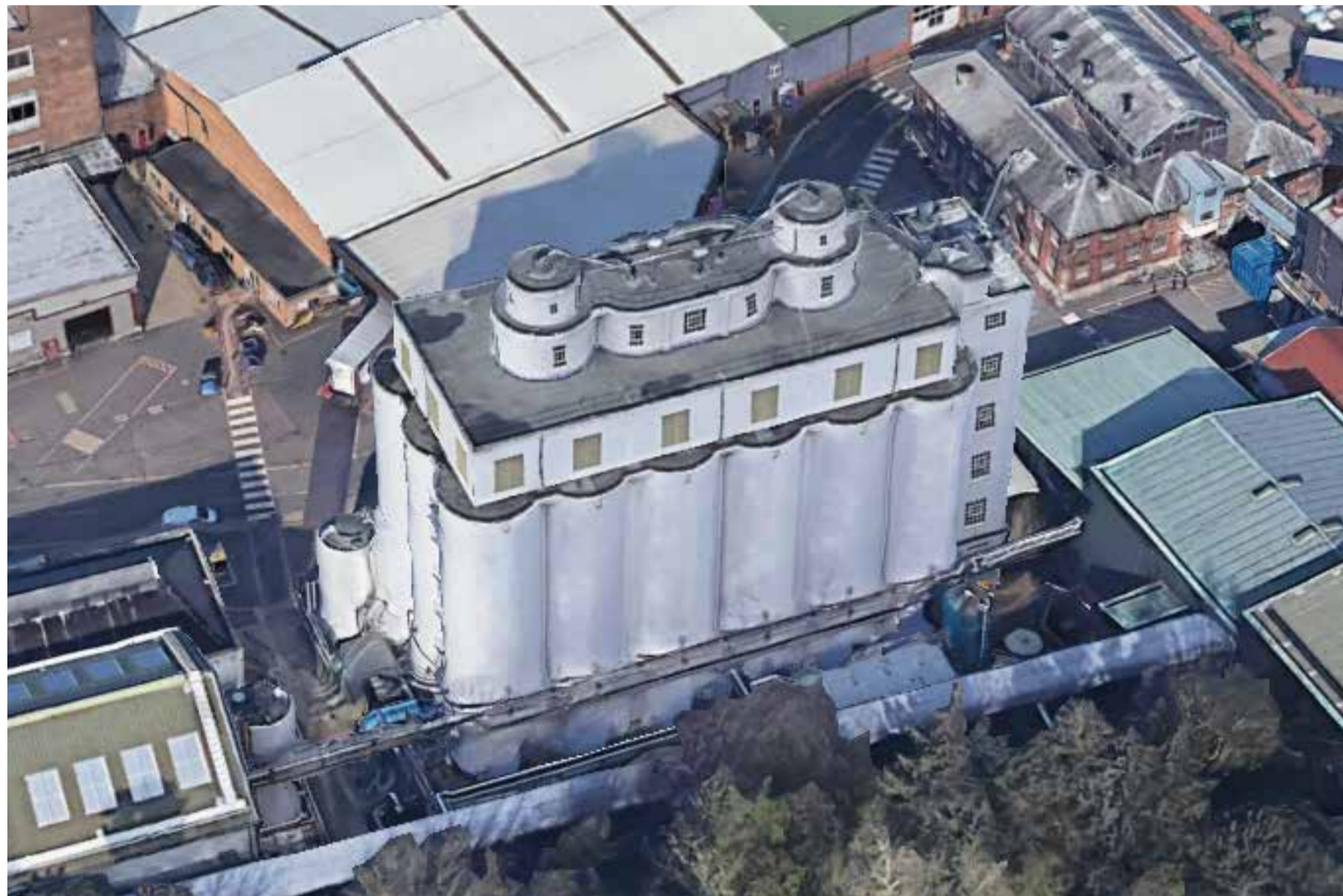
Existing Building To Be Demolished Aerial
