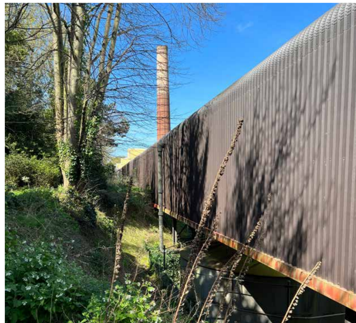
Existing Building To Be Demolished Photograph
