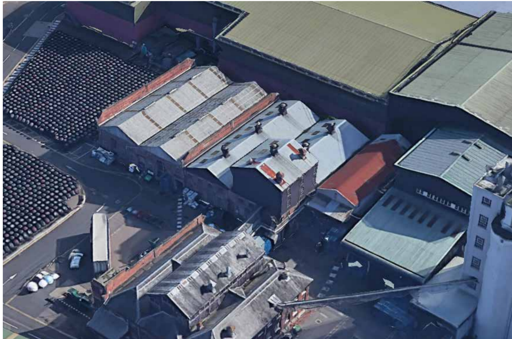
Existing Building To Be Demolished Aerial
