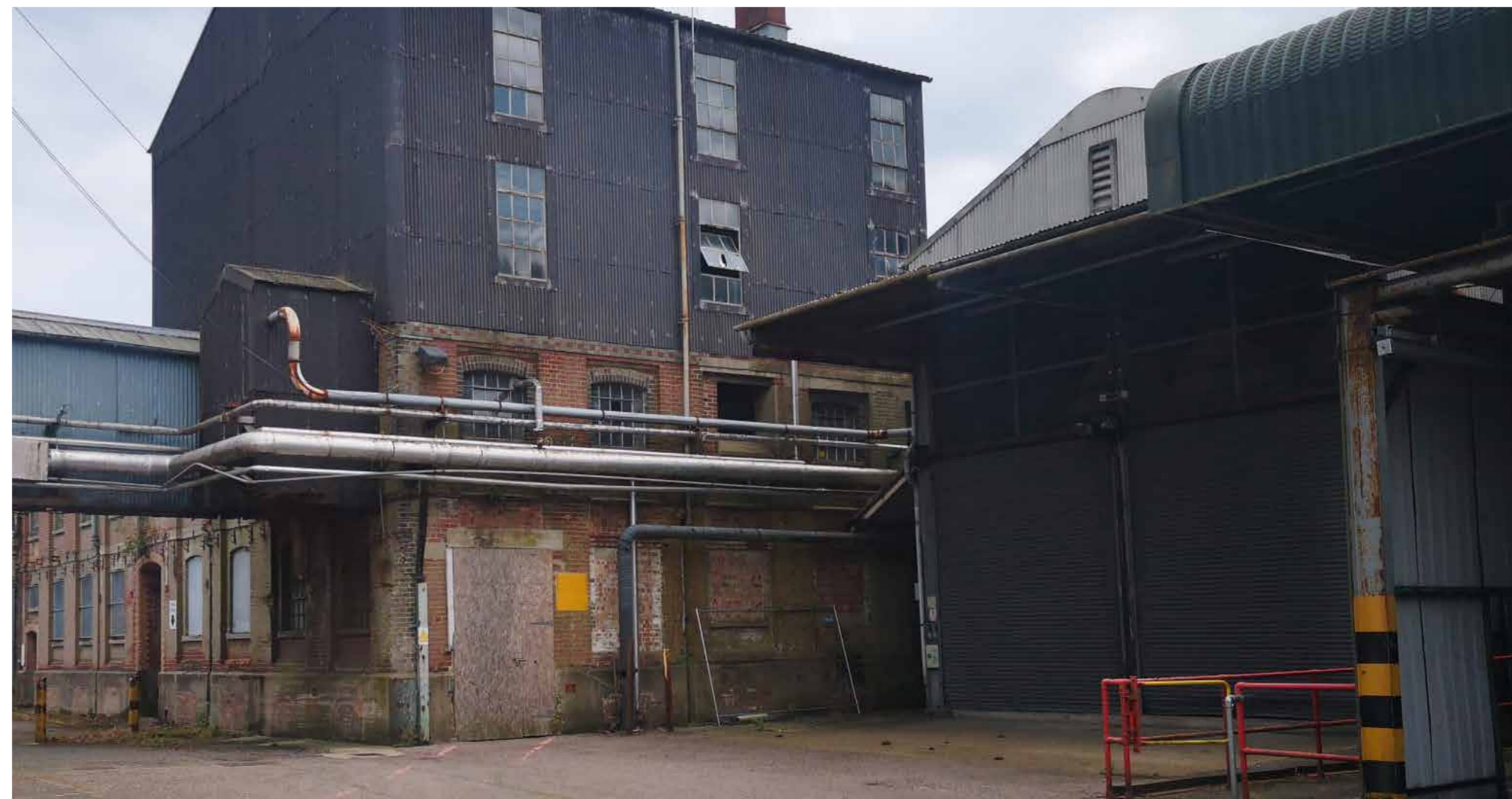
Existing Building To Be Demolished Photograph
