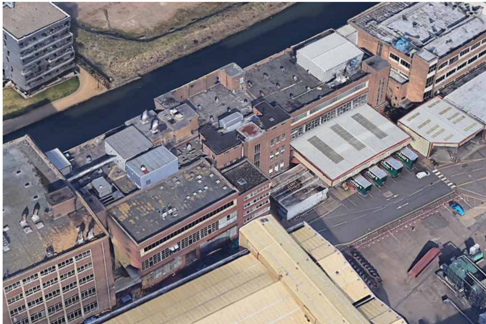
Existing Building To Be Demolished Aerial
