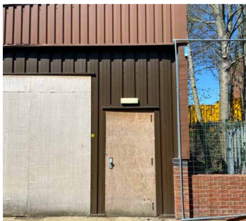
Existing Building To Be Demolished Photograph
