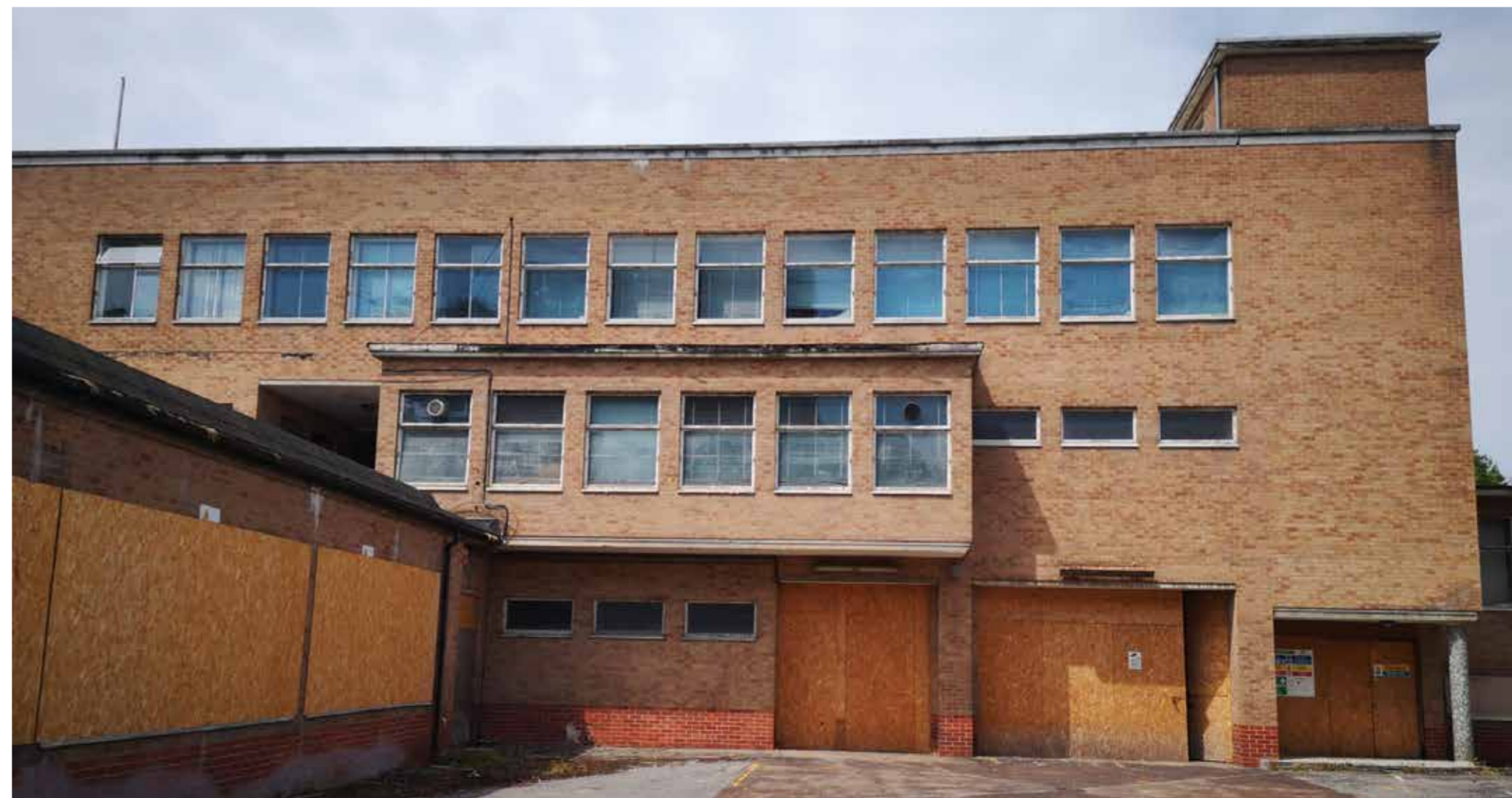
Existing Building To Be Demolished Photograph
