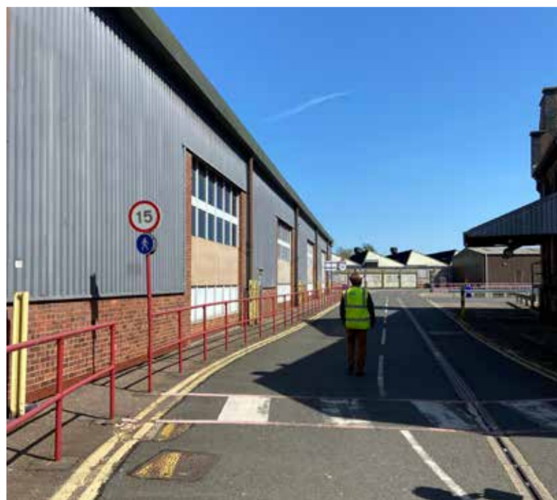
Existing Building To Be Demolished Photograph
