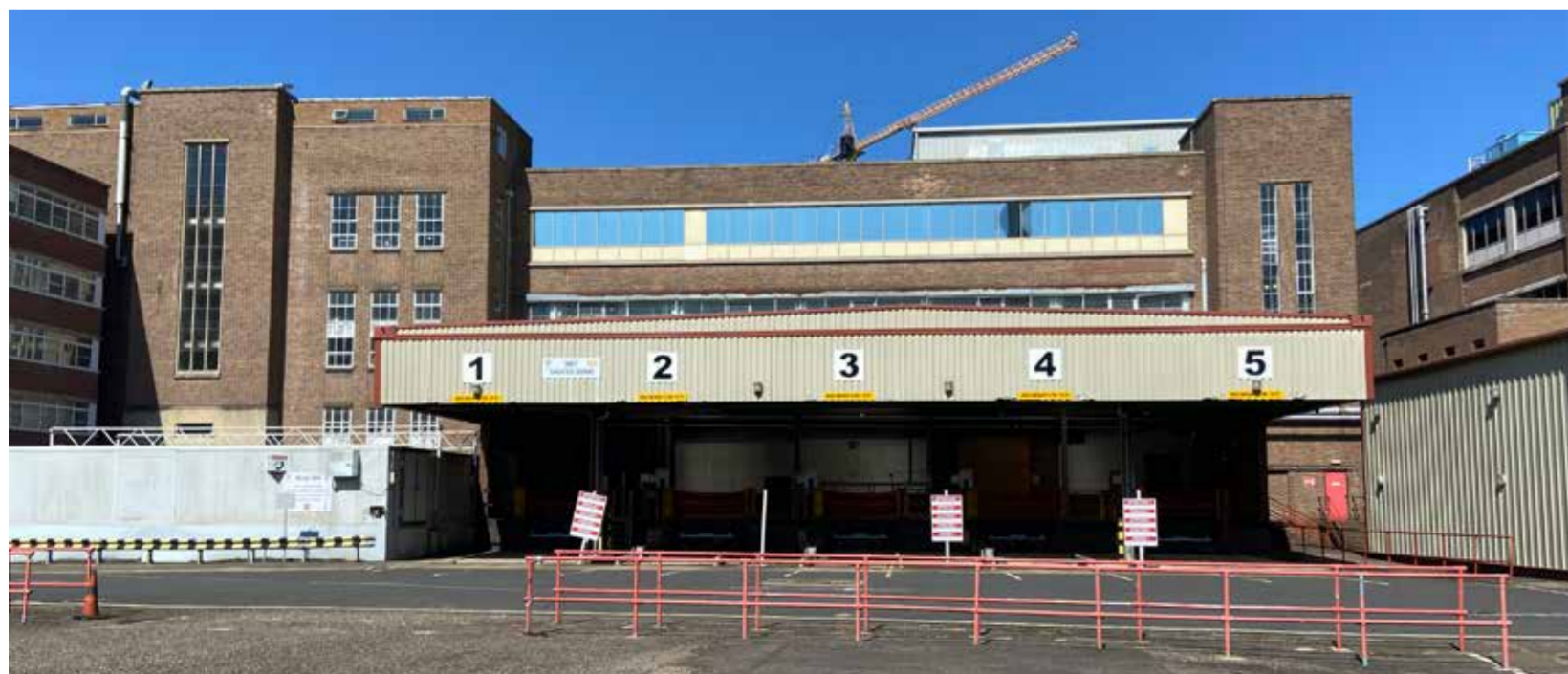
Existing Building To Be Demolished Photograph
