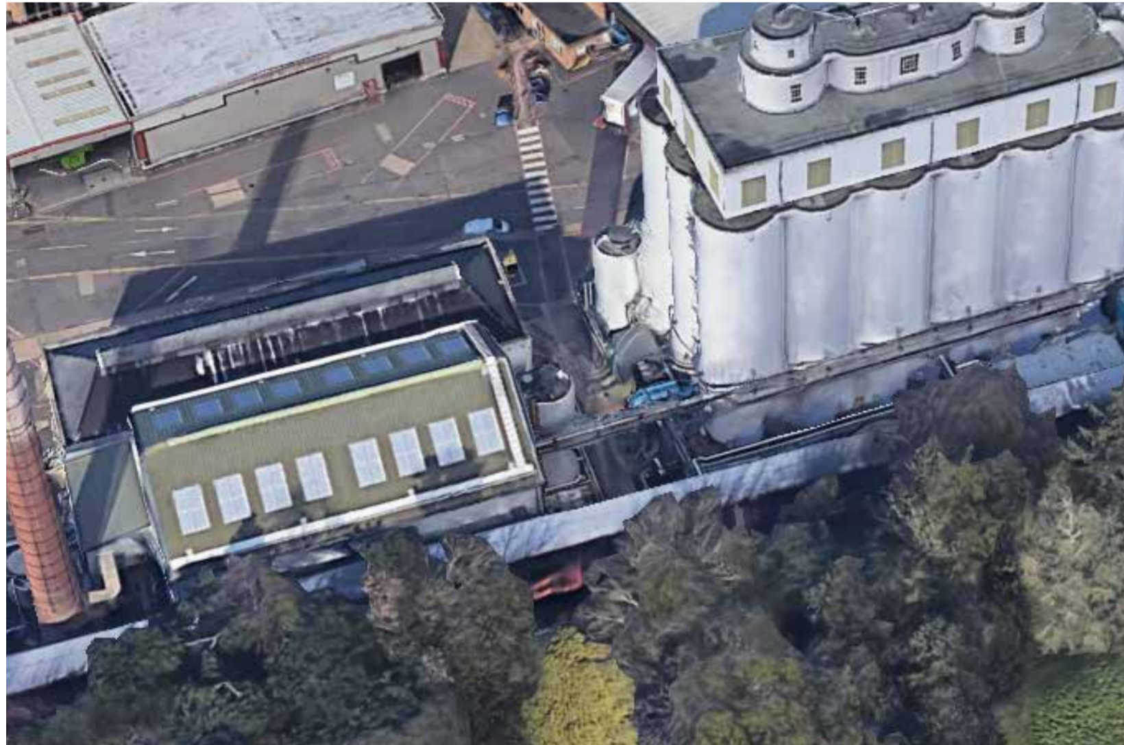
Existing Building To Be Demolished Aerial
