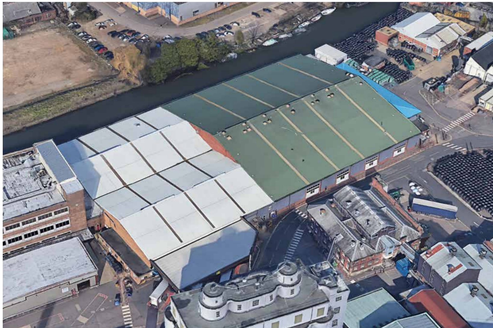
Existing Building To Be Demolished Aerial
