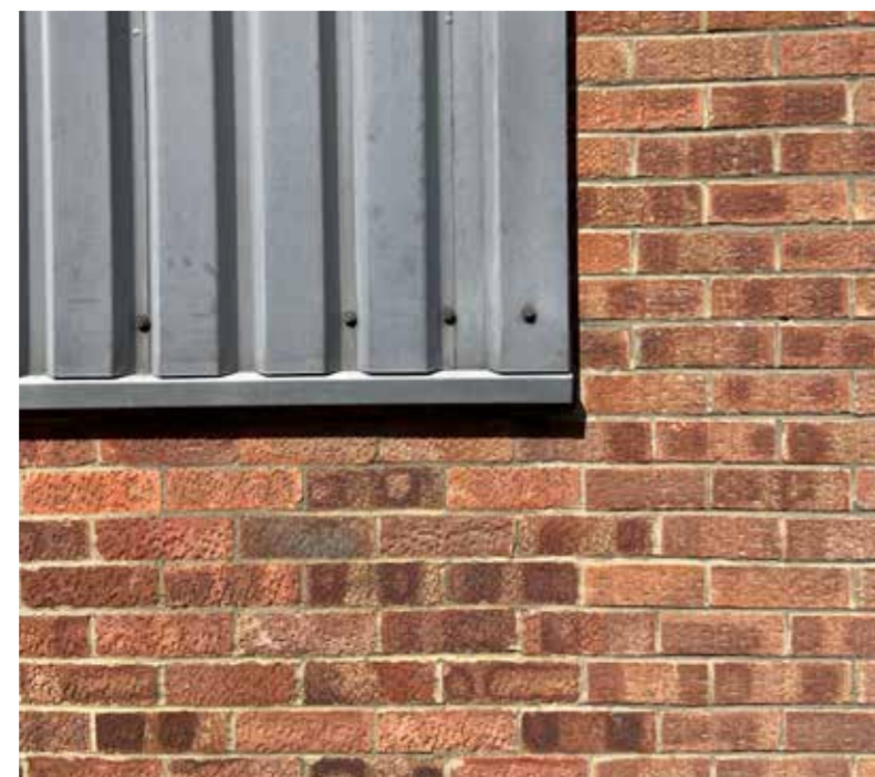
Existing Building To Be Demolished Photograph
