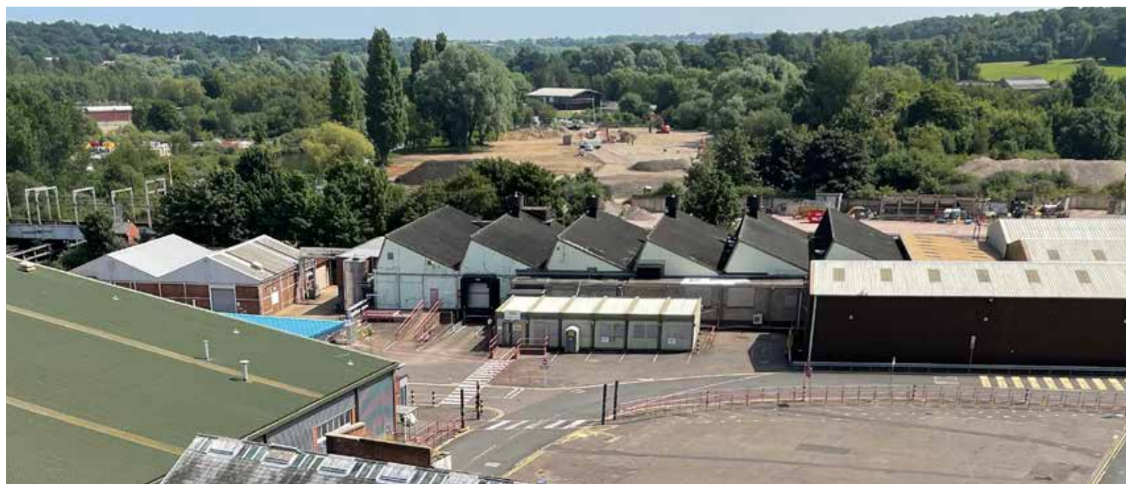
Existing Building To Be Demolished Photograph
