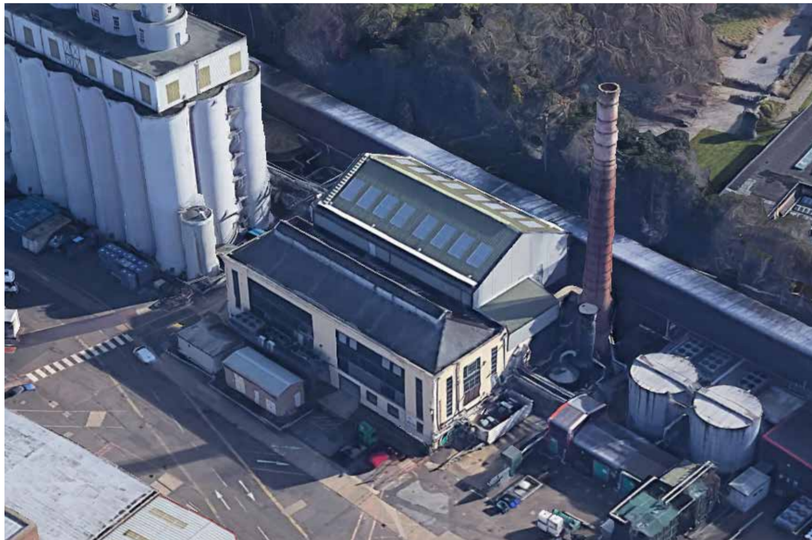
Existing Building To Be Demolished Aerial
