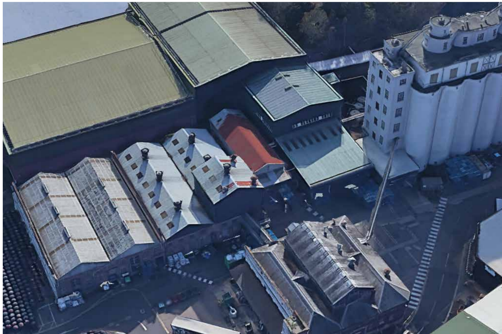
Existing Building To Be Demolished Aerial
