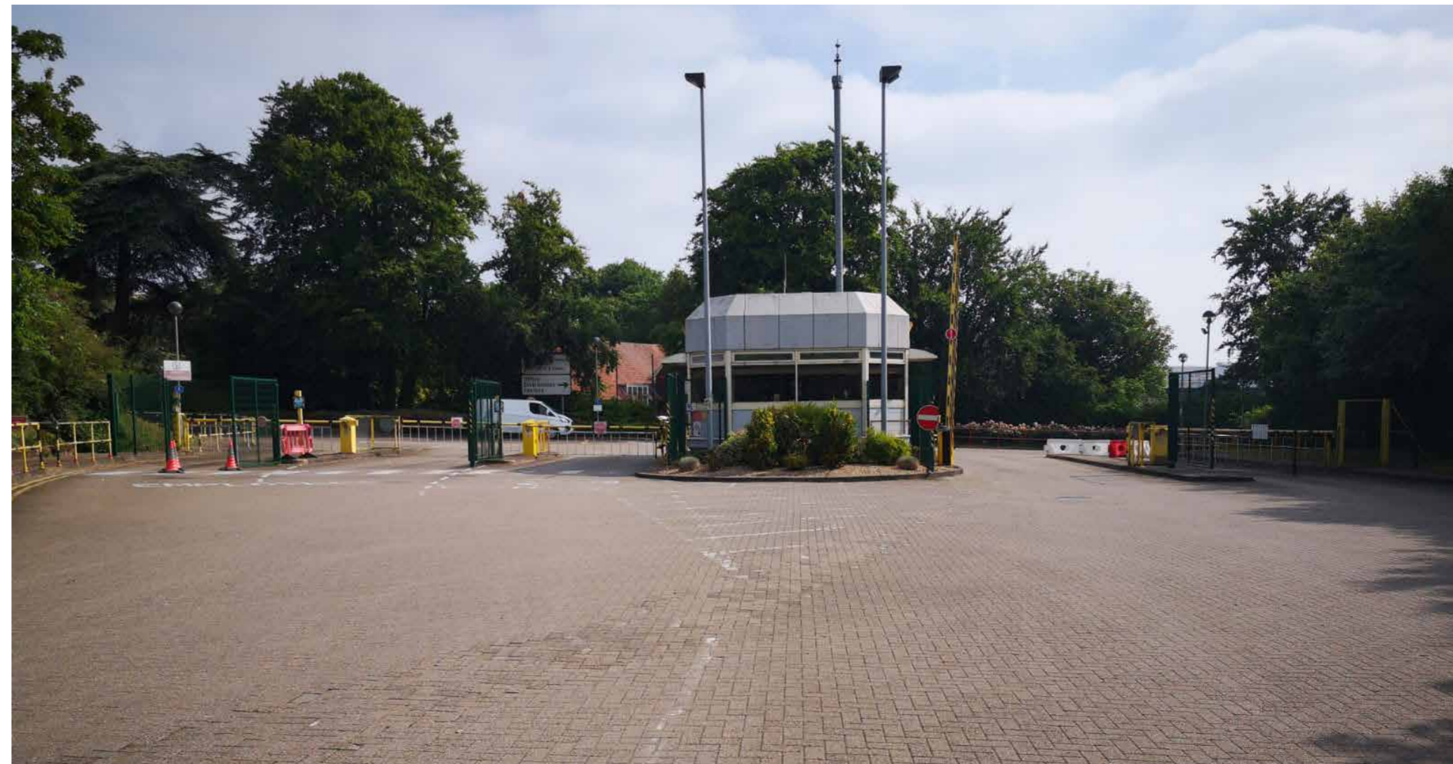
Existing Building To Be Demolished Photograph
