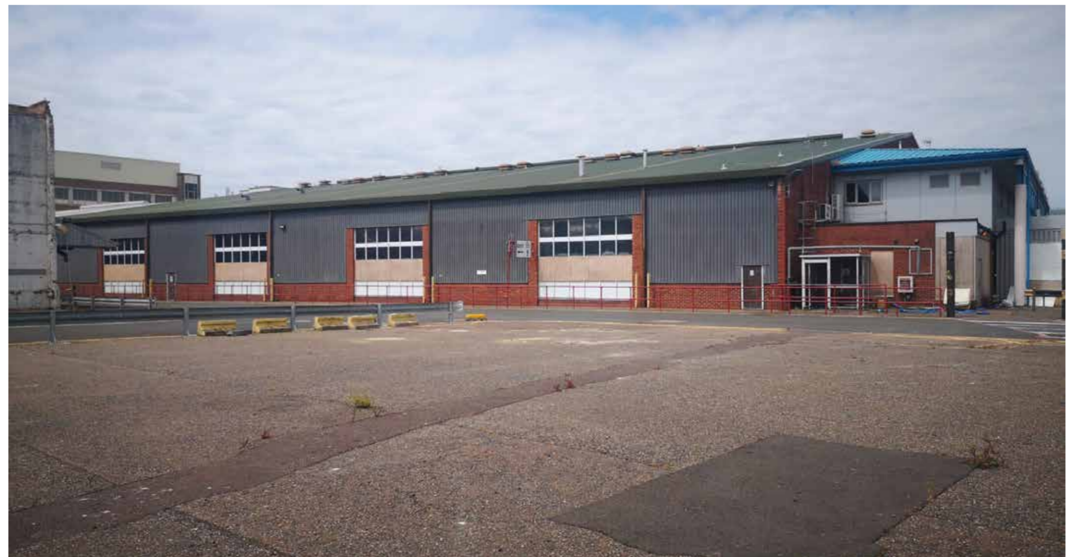
Existing Building To Be Demolished Photograph
