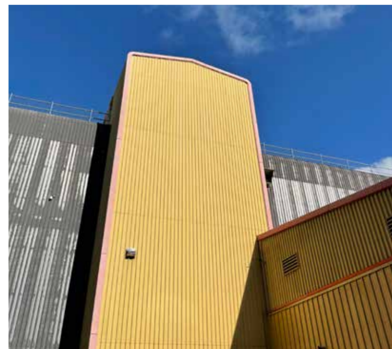
Existing Building To Be Demolished Photograph
