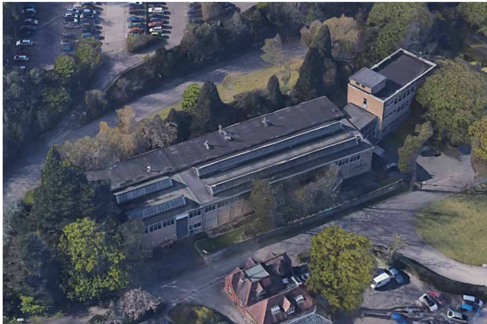
Existing Building To Be Demolished Aerial
