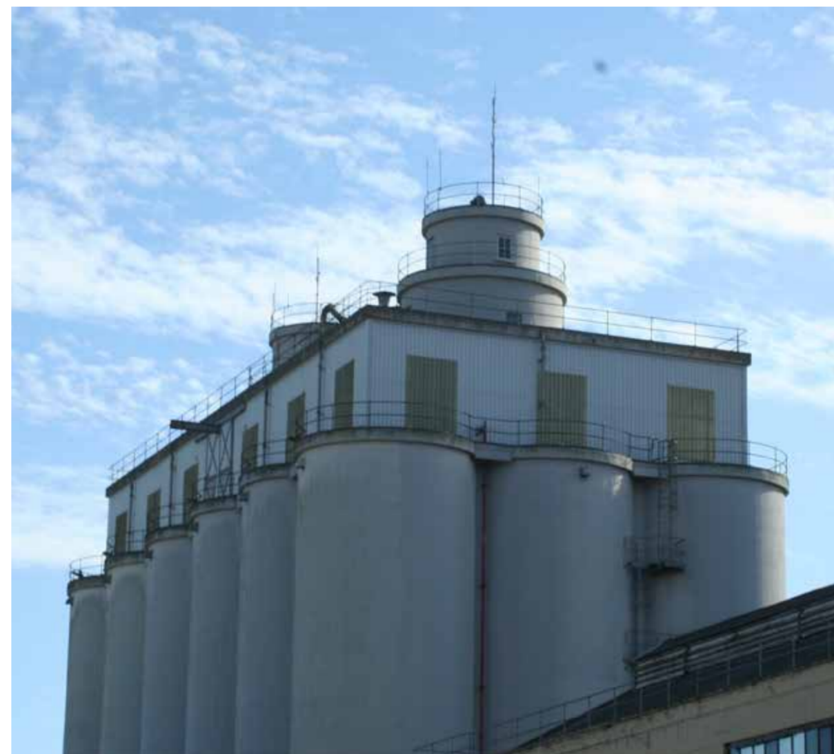
Existing Building To Be Demolished Photograph
