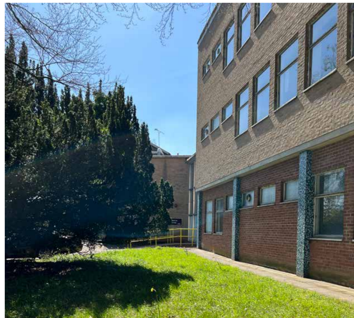
Existing Building To Be Demolished Photograph
