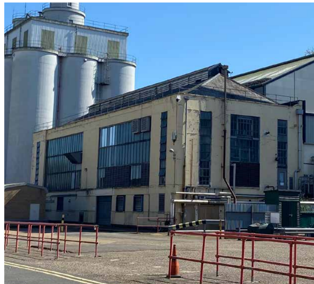
Existing Building To Be Demolished Photograph
