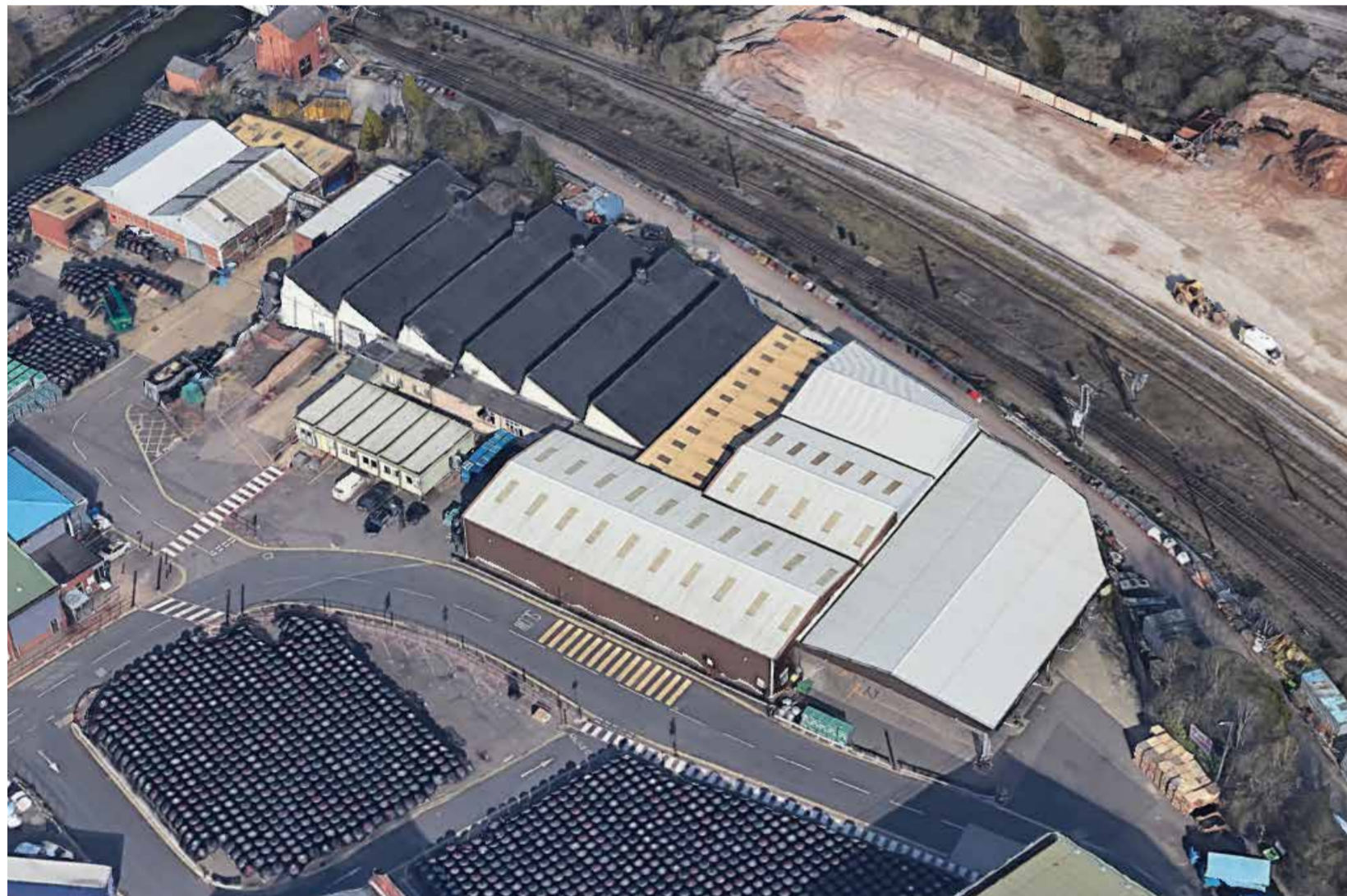
Existing Building To Be Demolished Aerial
