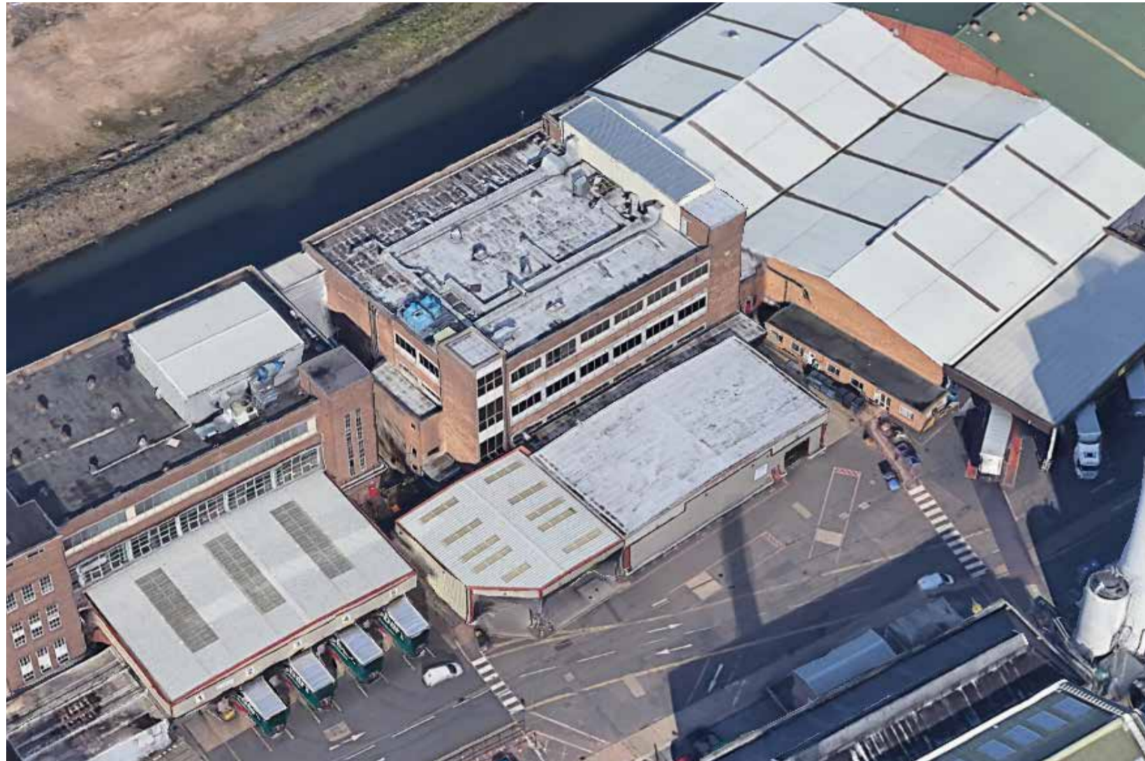
Existing Building To Be Demolished Aerial
