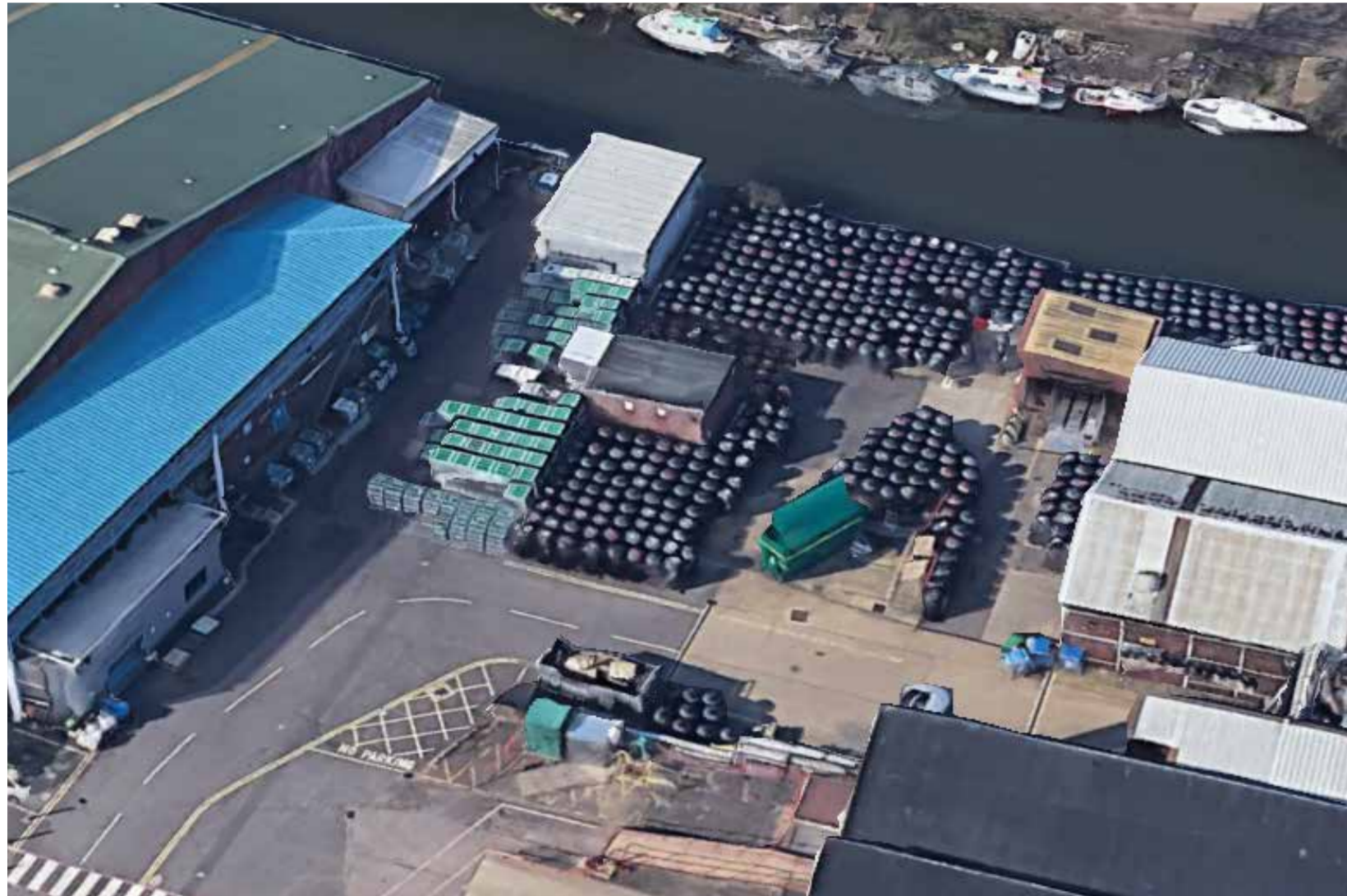
Existing Building To Be Demolished Aerial
