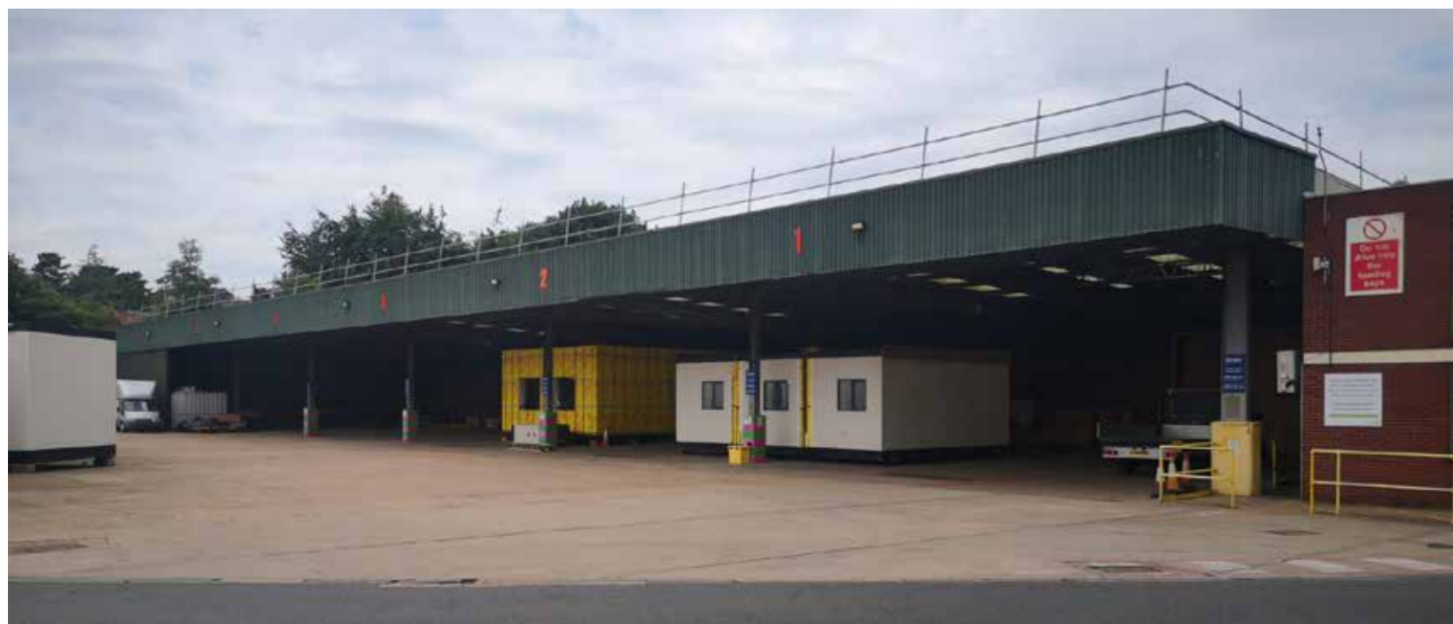
Existing Building To Be Demolished Photograph
