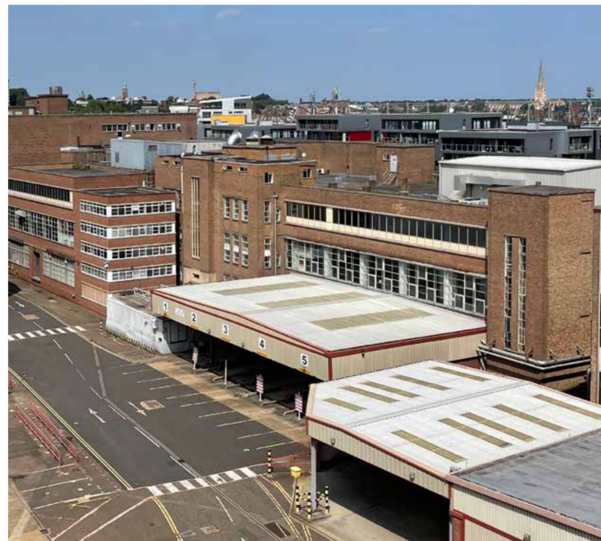
Existing Building To Be Demolished Photograph
