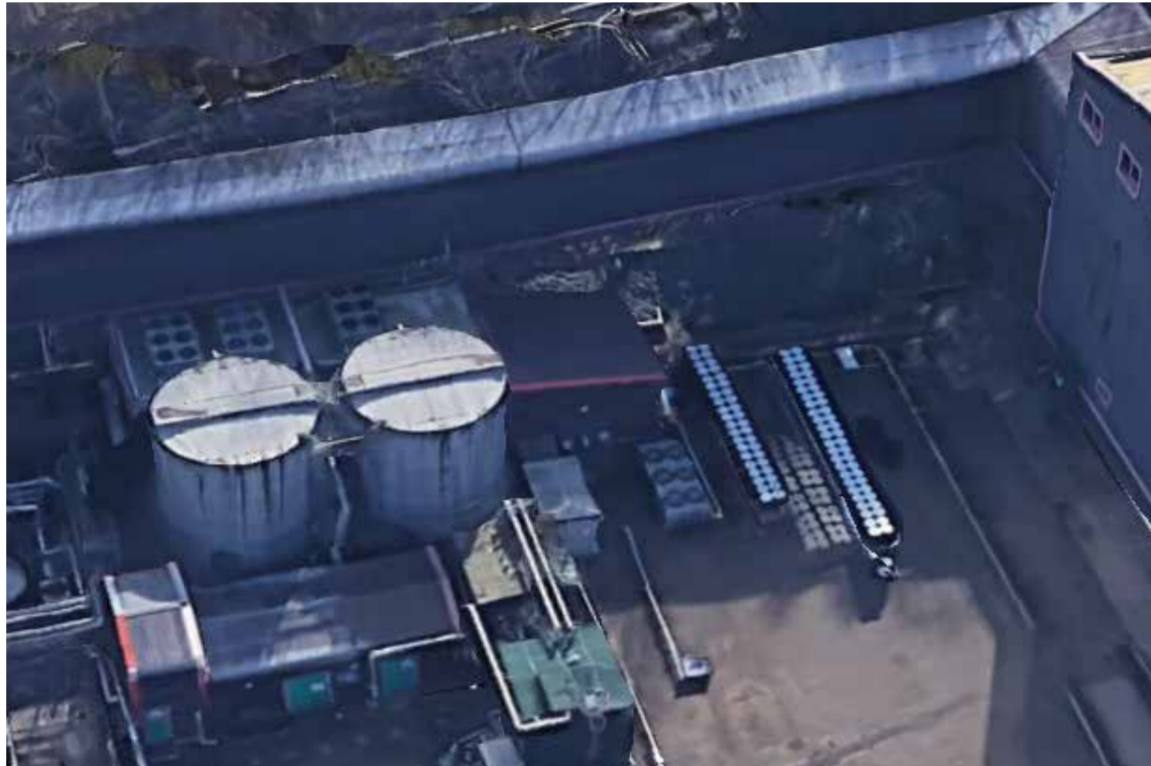
Existing Building To Be Demolished Aerial
