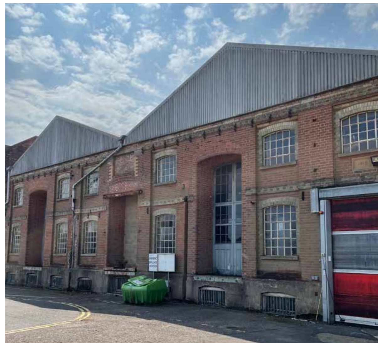
Existing Building To Be Demolished Photograph
