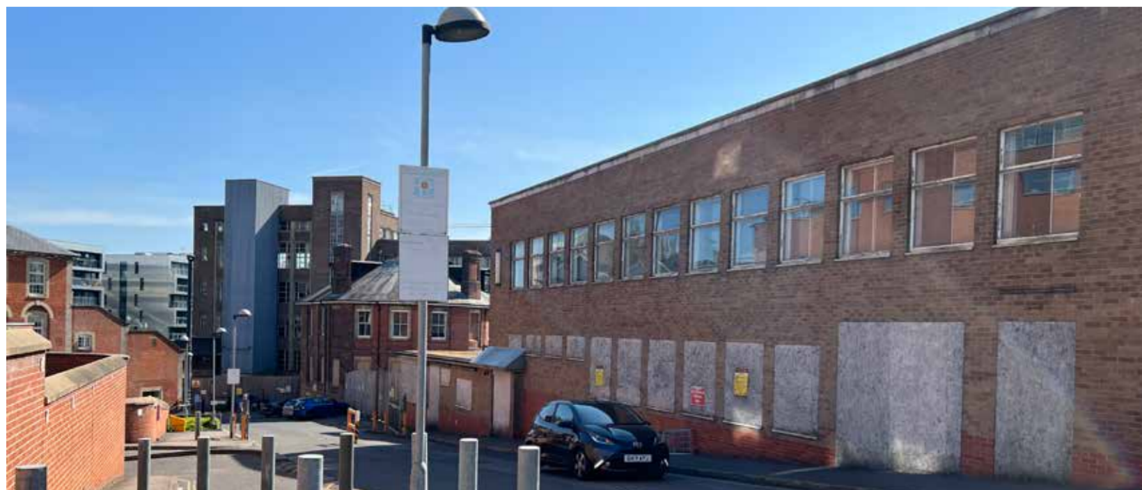
Existing Building To Be Demolished Photograph
