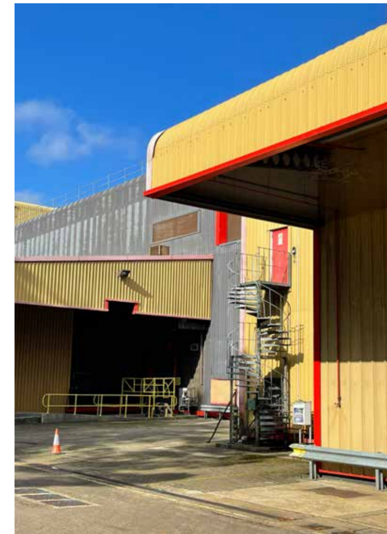
Existing Building To Be Demolished Photograph
