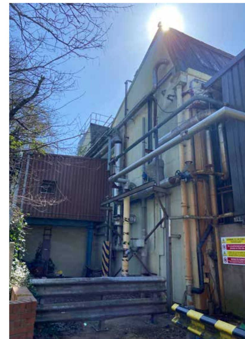
Existing Building To Be Demolished Photograph
