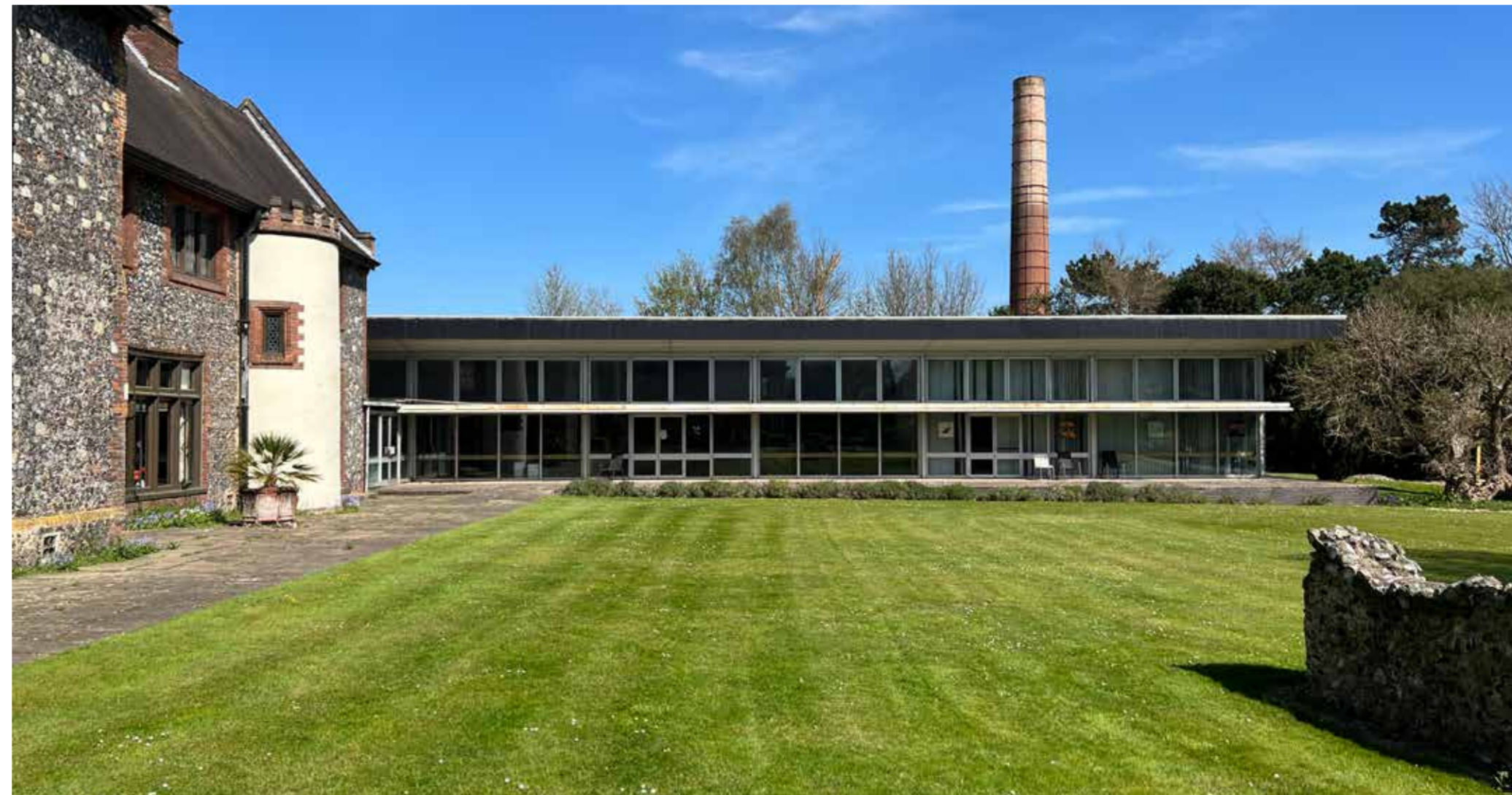
Existing Building To Be Demolished Photograph
